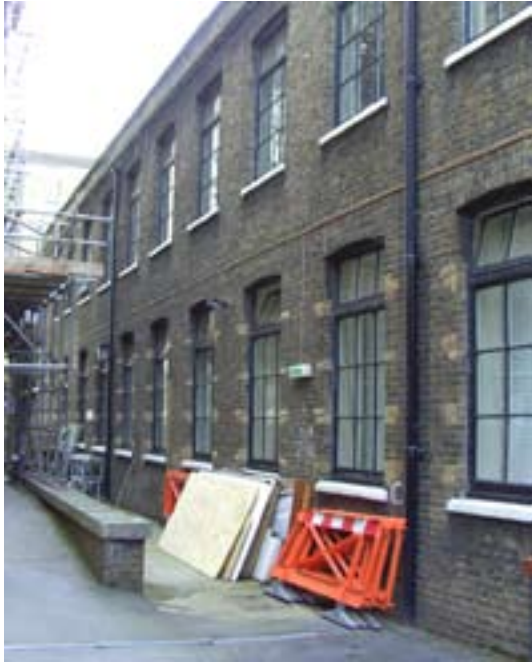
Figure 13 North elevation of the Bindery. Copyright English Heritage (DP070361)
