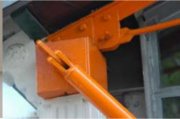
Figure 22 Gib and cotter joint, the 'Fish' restaurant, Cathedral Street, Southwark, 1897. Copyright English Heritage (DP070368)
