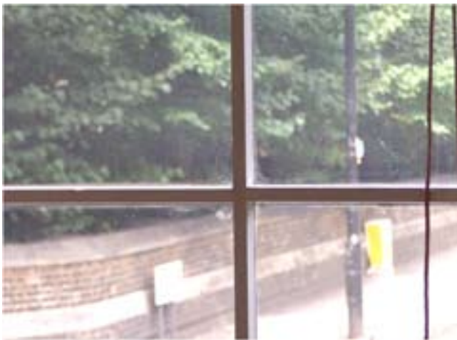
Figure 37 First-floor window, glazing bars without mouldings. Copyright English Heritage (DP070374)
