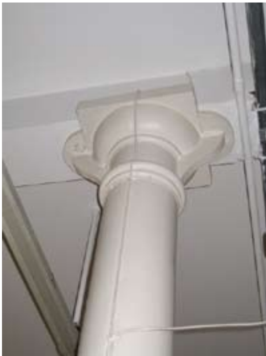
Figure 16 Cast iron column, ground floor, Bindery. Copyright English Heritage (DP070364)
