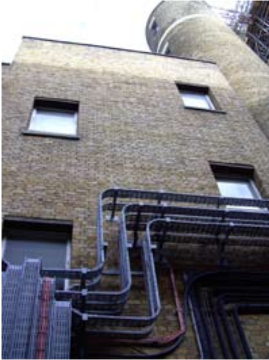
Figure 34 Rear elevation of 1–2 Montague Place, adjoining the staircase tower of the King Edward VII Galleries. Copyright English Heritage (DP070371)
