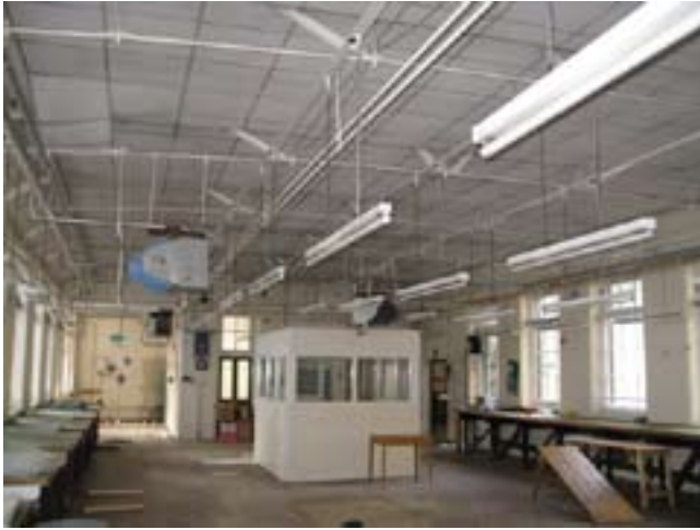
Figure 15 Interior view of the Bindery, first floor. Copyright English Heritage (DP070363)
