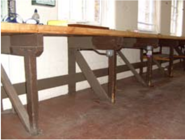
Figure 19 Bindery workbenches, showing the original substructure. Copyright English Heritage (DP070365)
