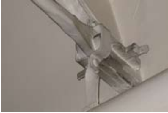
Figure 21 Gib and cotter joint, the British Museum Bindery, 1898. Copyright English Heritage (DP070367)
