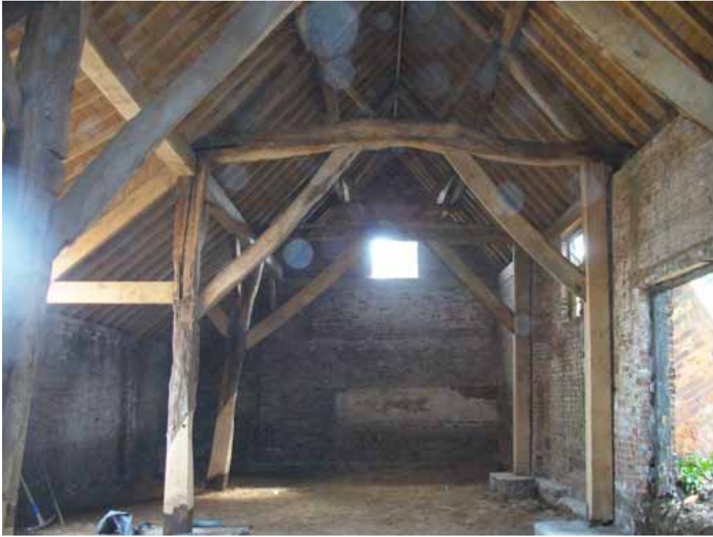
Figure 5: View of the trusses looking east
