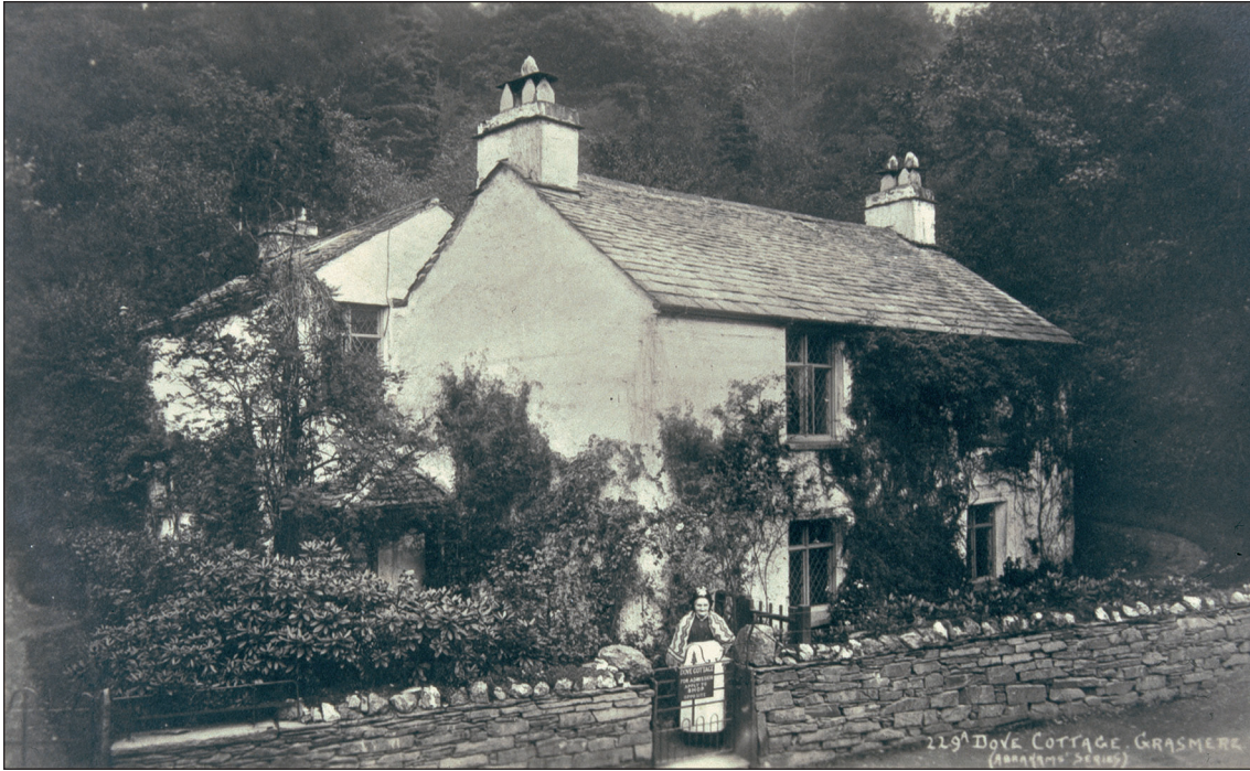
Fig 24: A c. 1900 postcard (by the Keswick-based Abraham family of photographers) showing the new windows to the front elevation. Mary Dixon, the first custodian, stands at the gate [WT]
