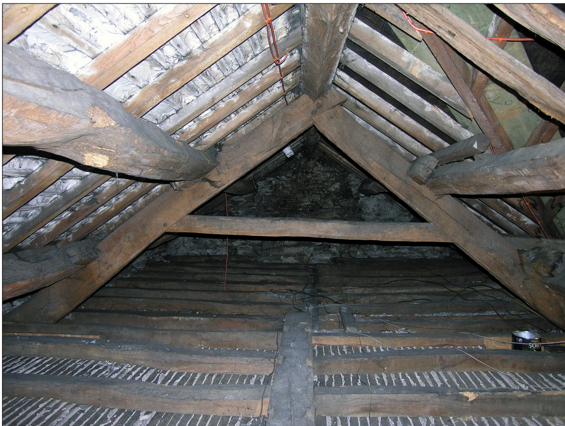
Fig 28: The roof of the front range, looking north-west [AM]
