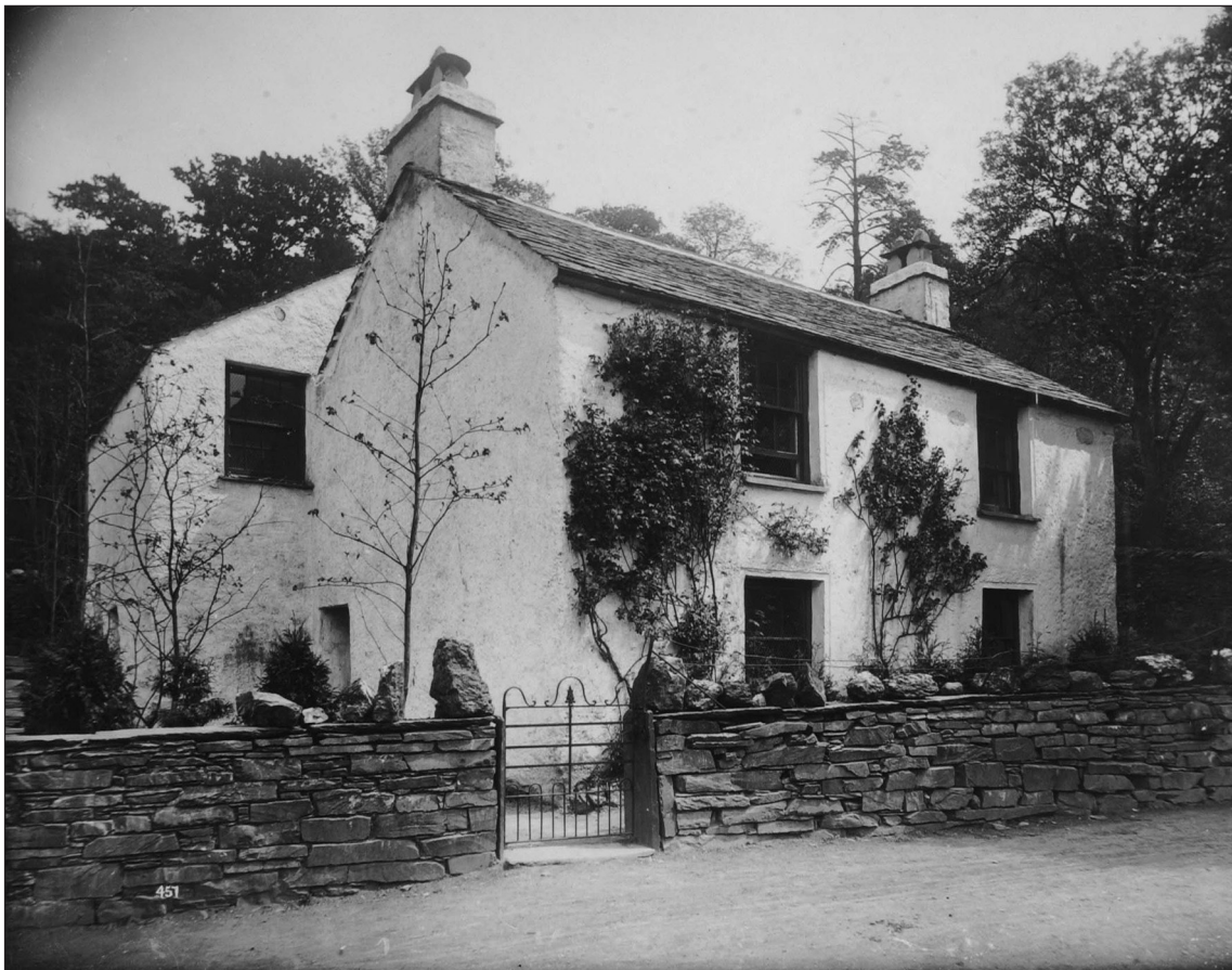
Fig 23: Herbert Bell photograph showing Dove Cottage prior to the replacement, in 1892, of late 19th-century sash windows [WT]
