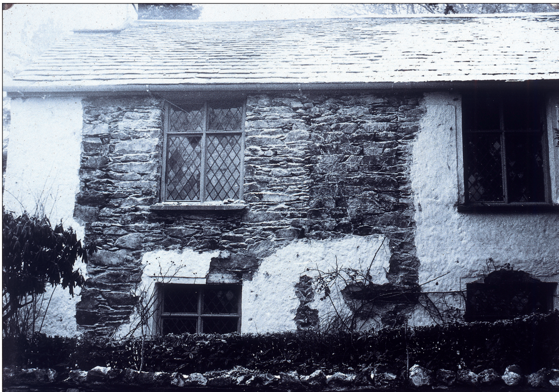
Fig 13: A 1970s photograph showing evidence for former first-floor window openings [WT]
