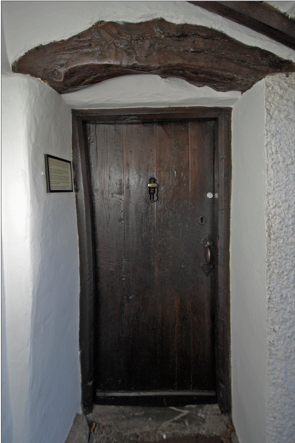
Fig 27: The lintel of the original entrance to Dove Cottage, exposed during the 1970s [dp056074]
