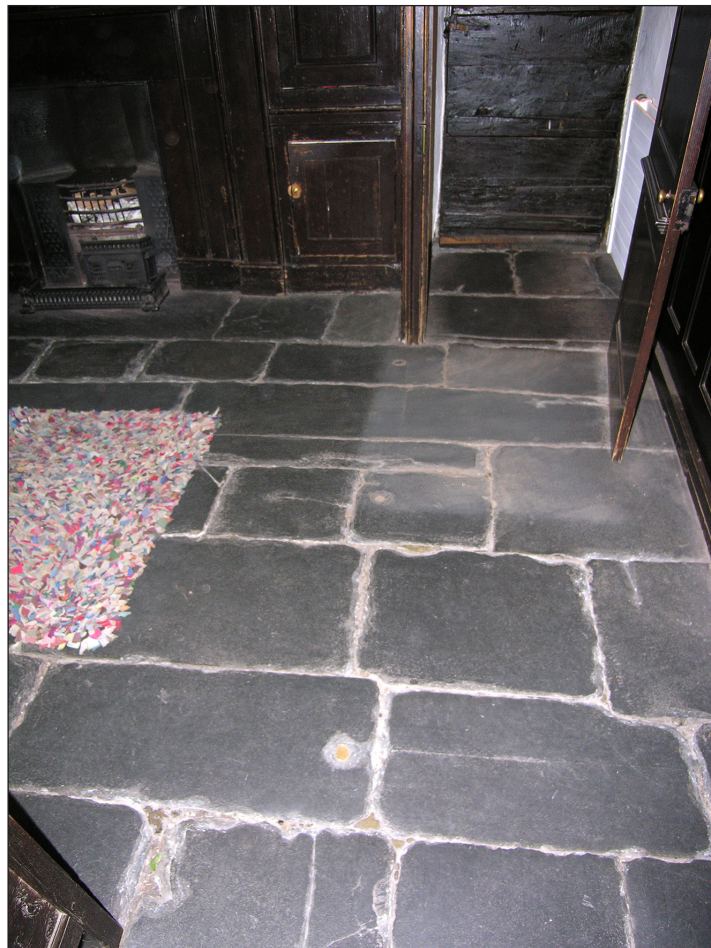
Fig 33: Evidence, in the form of infilled round holes in the floor, for the former partition defining a passage at the north-east end of the houseplace [AM]
