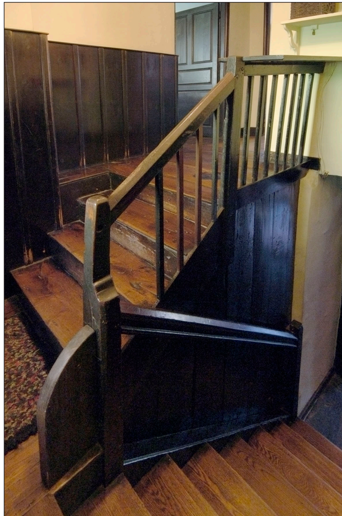
Fig 42: The stair seen from the garden entrance onto the half-landing [dp056086]
