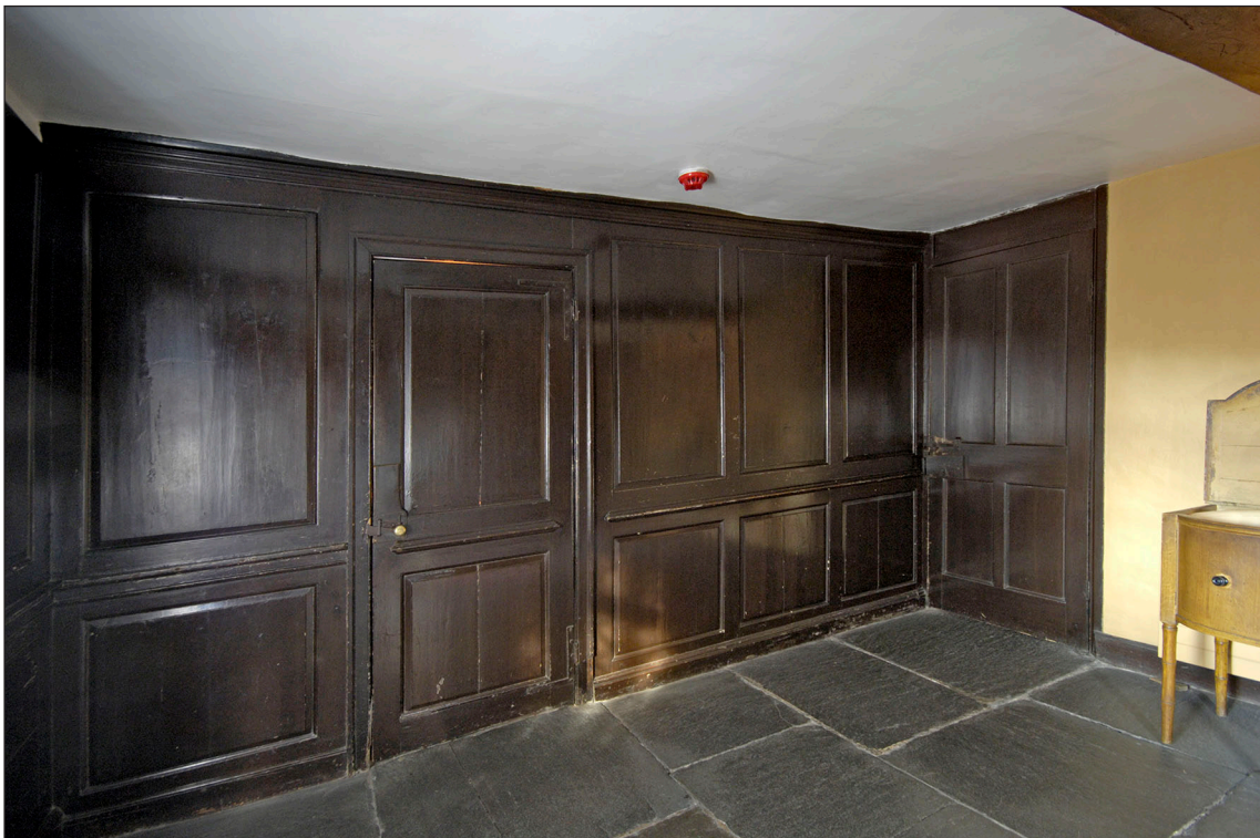
Fig 38: The wainscot partition forming the north-west side of the parlour [dp056083]
