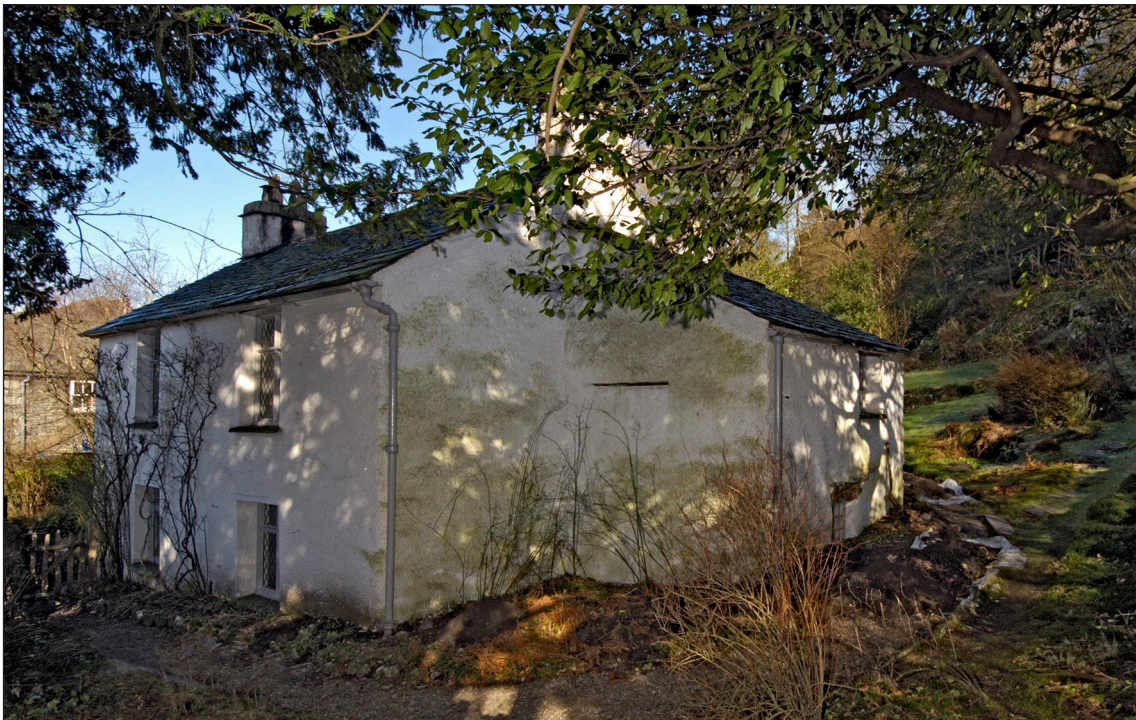
Fig 17: 'Out-jutting' showing the drip stone in relation to roof heights [dp056067]
