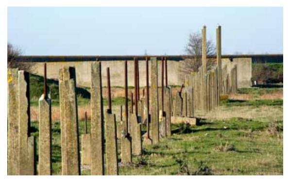
Figure 38: Part of **L1**, showing the posts at the north end aligned on a notch in the top of structure **24**, looking north. Also note the fall in post heights from north to south between structure **24** and the taller group of four posts, and again in the group of posts immediately to their south. Extract from NMR DPI41606 07-Mar-2011, Steve Cole © English Heritage.
