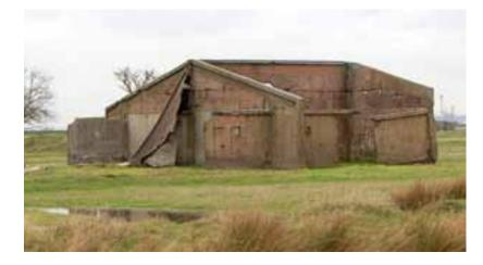
Figure 168: The remains of cordite drying stove **154** showing the characteristic reddening of the concrete caused by thermal remediation. Photograph: Rebecca Pullen 2011 © English Heritage.
