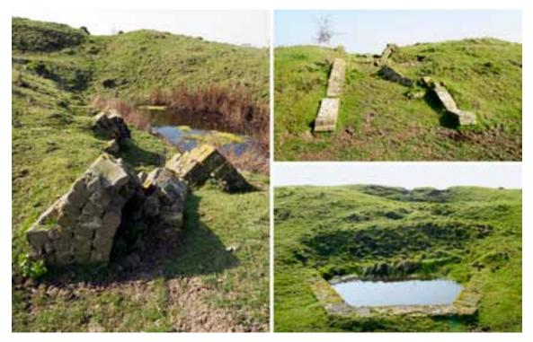
Figure 135: (clockwise from left) Collapsed vaulted brick tunnel on the north-east side of **166**; in-filled wide entrance on the south-west side of **166**; and trapezoidal tank or forecourt on the north side of **167**. Extracts from NMR DP141682, DP141683 and DP141679 08-Mar-2011, Steve Cole © English Heritage.
