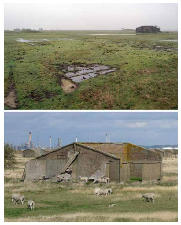
Figure 103: The two forms of cordite drying stove remains present in **Area E**, showing (top) the floor plan remains of former brick structure **147**, looking south-east, and (bottom) the standing reinforced concrete remains of structure **153**, looking north-east. Photographs: Rebecca Pullen 2011 (top) and Wayne Cocroft 2010 (bottom) © English Heritage.
