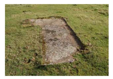
Figure 158: Structure **202** looking east, showing the low platform with L-shaped concrete floor with moulded floor drain. Photograph: Rebecca Pullen 2011 © English Heritage.
