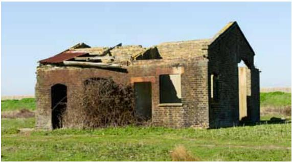
Figure 50: The south-east and north-east elevations of structure **23**, showing the two distinct forms of door and window openings, and the remains of the lightweight roof. NMR DPI41536 07-Mar-2011, Steve Cole © English Heritage.
