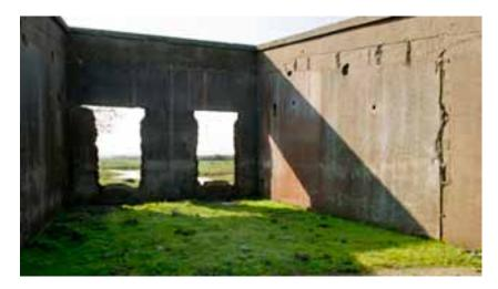
Figure 145: Inside a cell in press house range **247**, showing roof and walls scars, and various openings and conduit holes in the walls. Photograph: DP141655 08-Mar-2011, Steve Cole © English Heritage.
