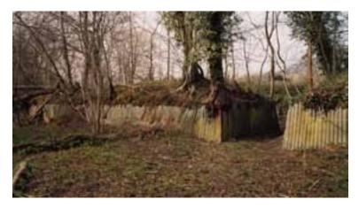
Figure 106: A corrugated iron earth-filled traverse known as a 'Chilworth Mound' shielding the front of an explosives magazine at the Chilworth Factory, Surrey. NMR AA044446, Wayne Cocroft © English Heritage.
