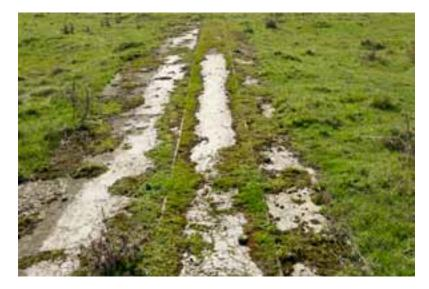
Figure 90: Iron tram rails and cambered cement tram-bed between structures **107** and **108**, looking south-west. NMR DP141543 07-Mar-2011, Steve Cole © English Heritage.
