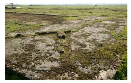
Figure 153: Acetone recovery stove foundation **240**, showing traces of the angled brick wall scars. Photograph: NMR DP141670 08-Mar-2011, Steve Cole © English Heritage. contemporary shift in opinion towards the general belief that steam dries more efficiently if it enters the building at top.
