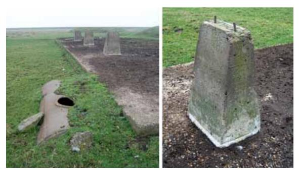
Figure 88: (left) South edge of structure **101** showing the iron tank and trapezoidal concrete plinths, looking west; (right) detail of one of the trapezoidal concrete plinths. Photographs: Rebecca Pullen 2011 © English Heritage.
