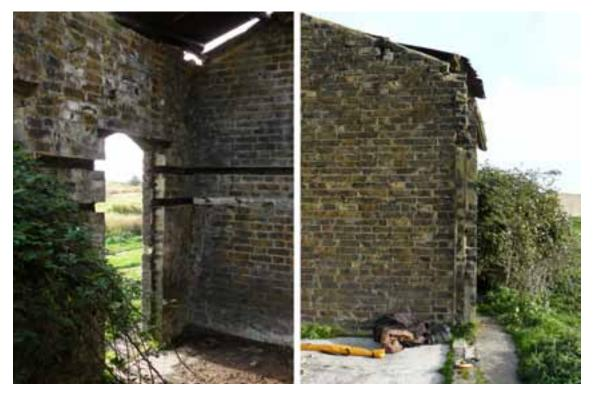
Figure 51: (left) Recessed grooves within the west room of structure **23**, with part of a wooden baton in situ. Photograph: Wayne Cocroft, 2010 © English Heritage.
