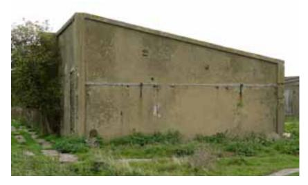
Figure 146: Cordite Press House **246**, showing iron brackets and witness marks for a lean-to structure at the west end. Photograph: Wayne Cocroft, 2010 © English Heritage.
