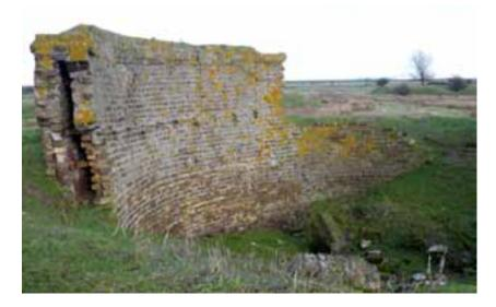
Figure 60: The interior face of the revetment wall belonging to structure **30**, showing the wall cavity and the midheight line of joist sockets. Photograph: Rebecca Pullen, 2011 © English Heritage.
