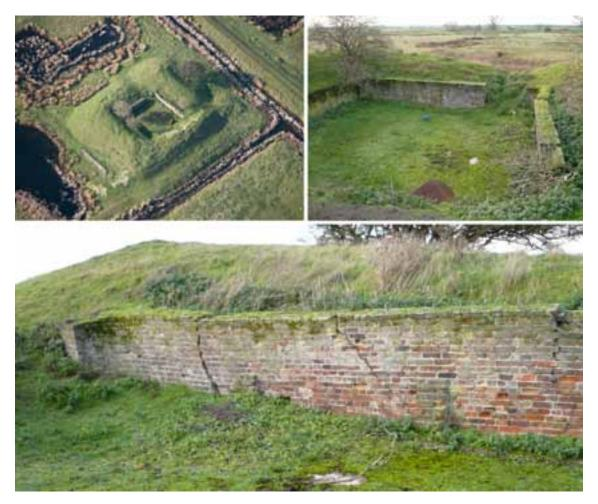
Figure 105: Structure **156** (clockwise from top left): oblique aerial view looking north-west; interior looking west; detail of the north stretch of the internal revetment wall suffering with subsidence. Photographs: Extract from NMR 26890/039 08-Mar-2011, Damian Grady (top left), and two ground shots, Rebecca Pullen 2011 © English Heritage.
