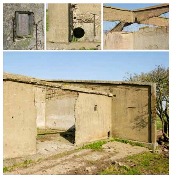
Figure 157: Cordite drying stove **205** (clockwise from top left): squint window detail; circular opening for a pipe at the base of the front wall; damage and degradation of the walls; and south- and west-facing elevations of the south-west stove compartment showing the roof scar and smooth square floor for the lean-to porch. Photographs (clockwise from top left): Wayne Cocroft 2010; NMR DP141706; DP141707; DP141705 08-Mar-2011, Steve Cole © English Heritage.
