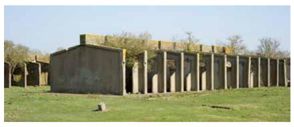
Figure 149: Structure **245** showing the cement rendered outward-facing cells, looking northeast with **244** behind. NMR DP141685 08-Mar-2011, Steve Cole © English Heritage.
