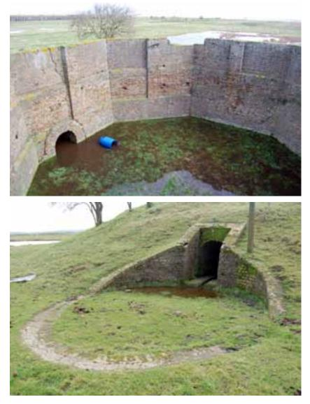
Figure 131: The waterlogged interior of **168**, showing the construction of the revetting wall, with the low tunnel entrance on the north side, and notch in the brick parapet at the northeast side. Photograph: Sarah Newsome 2011 © English Heritage.
