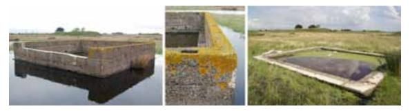
Figure 107: Structure **158** (left and centre) as recorded during the survey at the start of 2011, detail of hole cut into the corner to hold a superstructure or cover, and (right) with the sides reduced to ground level, as seen in Summer 2012. Photographs: Sarah Newsome 2011 and 2012 © English Heritage.
