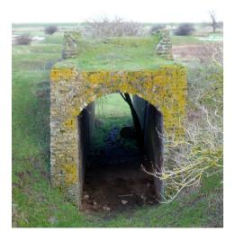
Figure 57: (far left) Entrance to the access tunnel inside nitroglycerine hill **31**, with possible evidence for a structure on top of the brick arch. Photograph: Rebecca Pullen, 2011 © English Heritage.
