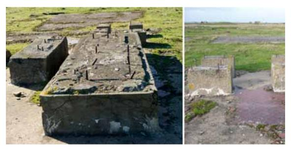
Figure 124: Structure **192** (left): large plinth showing the clear imprint of a machine preserved in its top, (right) smaller concrete plinths surrounded by remnants of a red quarry tile floor, looking north with structure **190** in the background. Photographs: NMR DP141572 07-Mar-2011, Steve Cole (left), and Rebecca Pullen 2010 © English Heritage.
