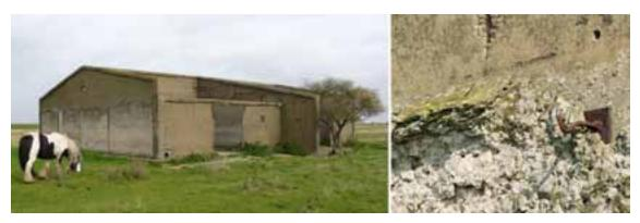
Figure 156: Cordite drying stove **205**, showing the rough-surfaced coating on the west gable end (left); and a detail of the pitched top, iron hooks, bitumen stain and small holes. Photographs: Rebecca Pullen 2011 © English Heritage.
