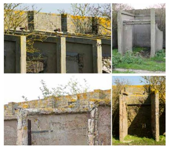
Figure 151: (upper pair) Acetone recovery stoves **245** (left) and **244** showing the outwardfacing rendered cells; (lower pair) structure **244** showing the inward-facing cells without render. Photographs: (top left) NMR DP141686 08-Mar-2011, Steve Cole; (top right and bottom left) Wayne Cocroft 2010; (bottom right) NMR DP141659 08-Mar-2011, Steve Cole © English Heritage.
