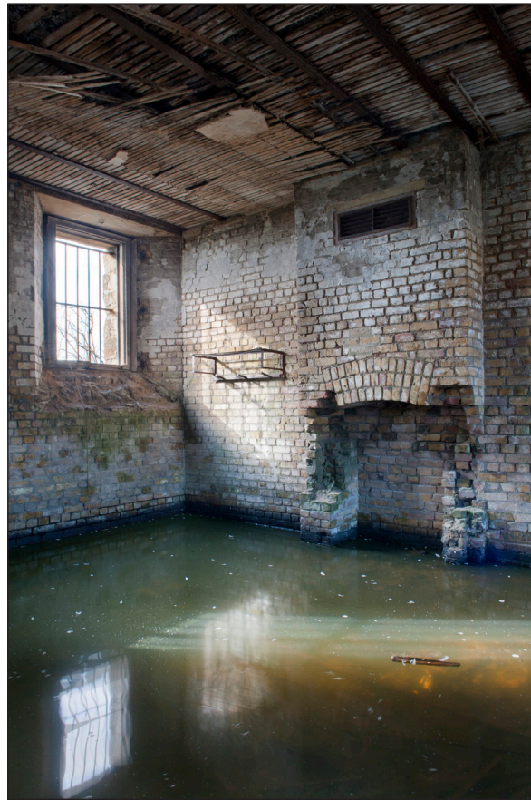
Figure 34: The interior of a Barrack Room intended for nine men [45]. The vent above the fireplace and the equipment rack set midway up the wall to the left of the chimney breast are visible. The iron shutters and the accompanying sill have been removed from the window. (DP 097489)
