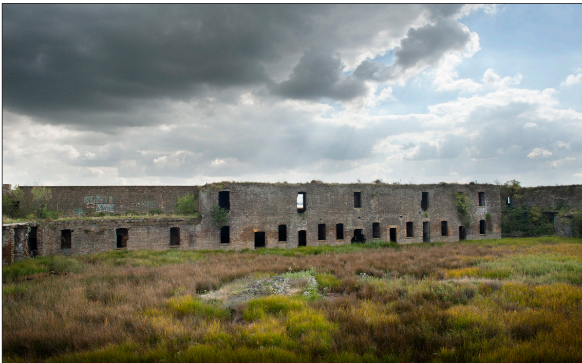
Figure 30: View of the south range across the parade ground. On the left are the single storey officers' quarters with loopedholed parapet above. The two-storey section on the right has the barracks on the ground floor with the hospital above. (DP 097500)
