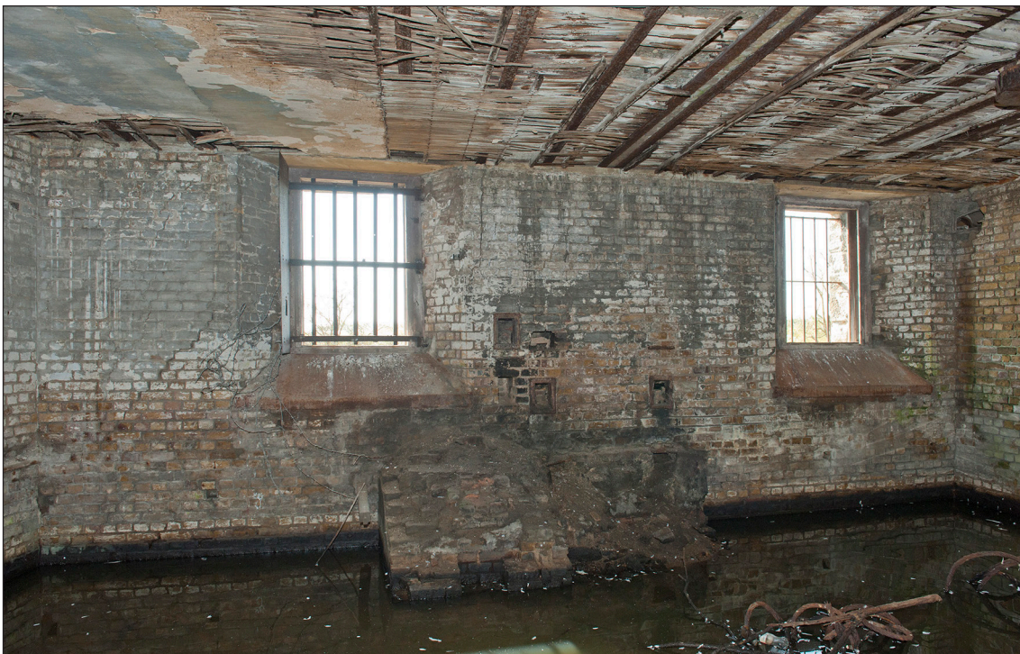
Figure 37: The brick bases for the washing coppers on the south wall of the Wash House and Laundry. (DP097511)
