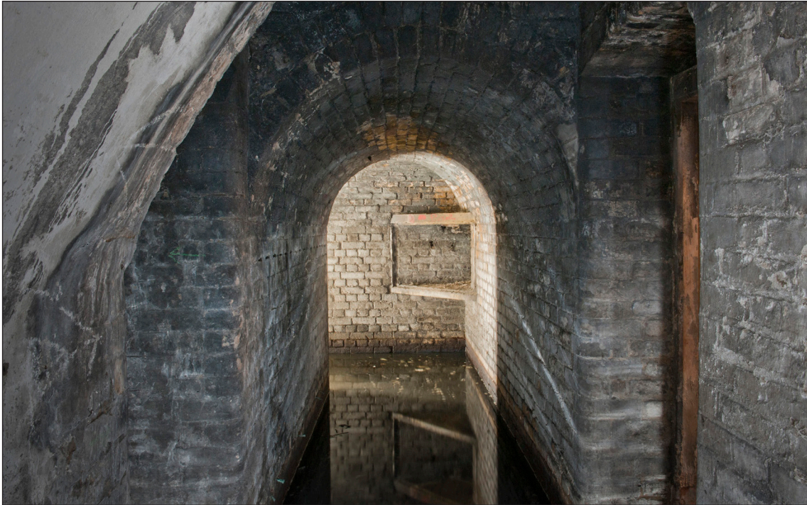
Figure 7: View looking south from a branch shifting passage into the intermediate dog-leg entrance passage. The area of white render and disturbed brickwork in the foreground on the left of the picture indicates the position of the removed wall. Beyond this is the crossing with the main lighting passage. The angled light box for the 90 degree turn in the dog-leg passage can be seen in the background. (DP 097426)
