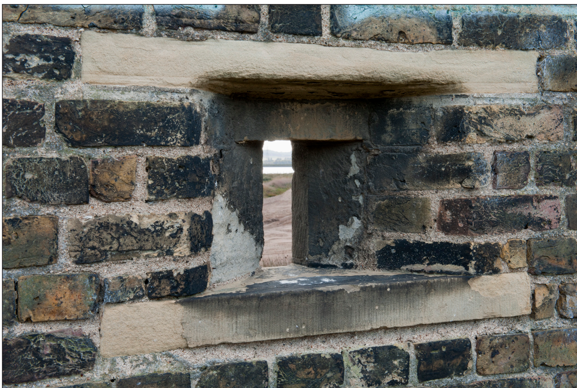
Figure 24: The interior of a loophole in the southern face wall of the fort. (DP 097575)
