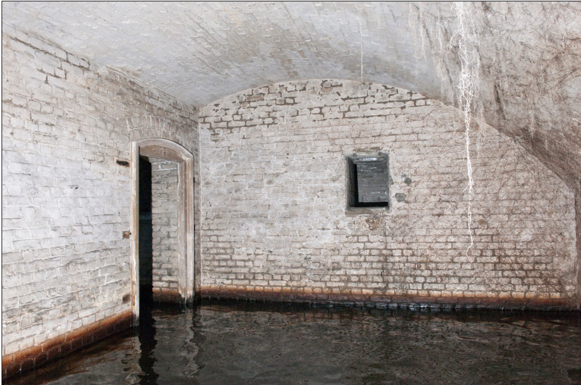
Figure 10: Interior of No 5 Spare Shell Store [92] which retains the plan and appearance of the ammunition stores as built. Note the light box in the rear wall and the sturdy timber door-frame with pegged joints and retained by noggins set in the brickwork. (DP097445)
