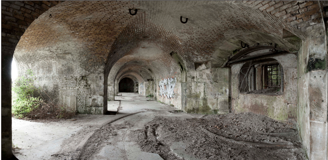
Figure 19: Interior of casemates 10 to 14, looking south showing the open casemated gun floor on the west side of the battery. The change in the direction of the vaulting between the gun positions and the elongated piers of the blind casemates can be clearly seen as can the gun slinging hoops set in the vault and the course of the removed racer rails in the floor. (DP097616)
