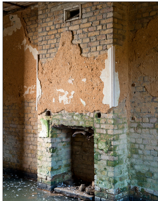
Figure 33: A chimney stack in the one of the officers' rooms with remains of the plaster moulding indicating the better quality decoration of these higher status rooms. (DP097480)
