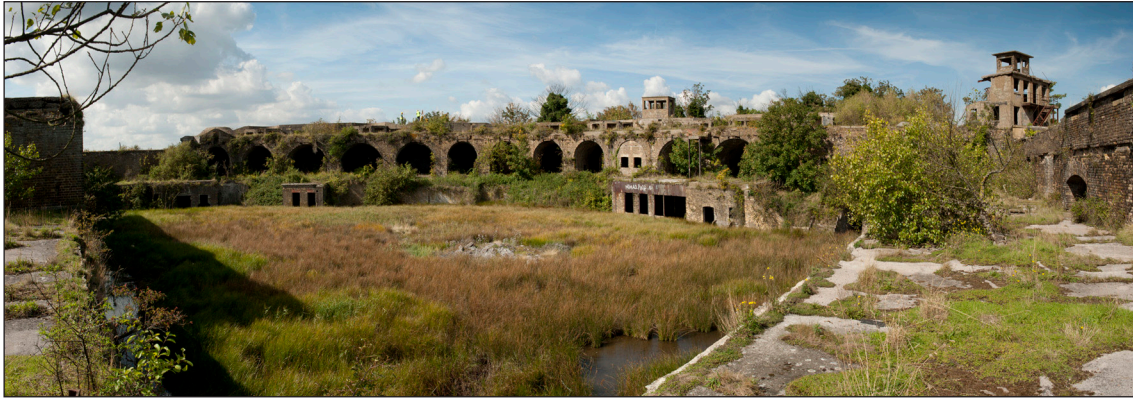
Figure 5: The interior of the fort in September 2010 from the south-east corner. From right to left, the main features that can be seen are the gorge wall with the recess for the murder holes over the entrance, the First World War Battery Observation Post, the gun casemates with the Submarine Mining Test and Engine Rooms below and the early-20th century barbettes and emplacements for breech loading guns on the roof. (DP 097569)
