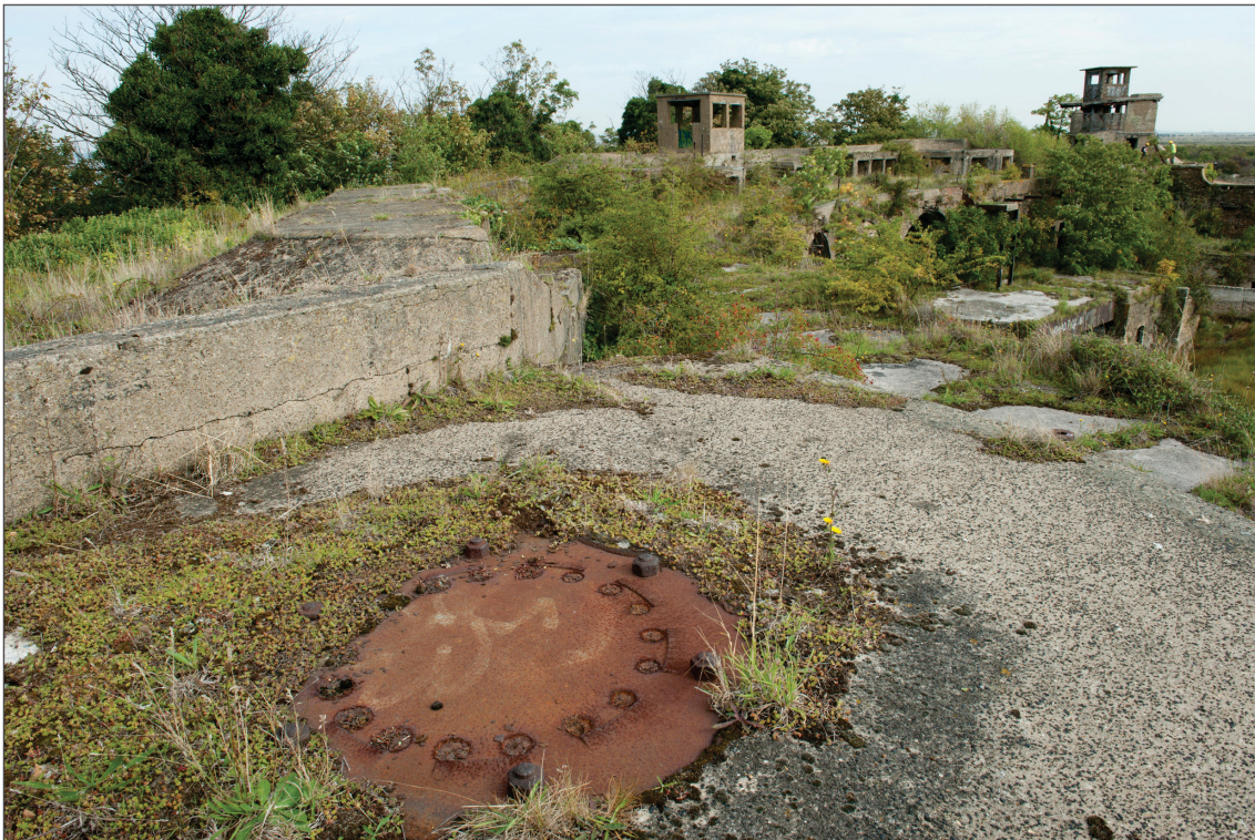
Figure 47: View of the north end of the fort roof from the 12-pounder B group, with a holdfast for this weapon in the foreground. The hut in the centre of the photograph dates from the Second World War; beyond it are the 6-inch gun positions and the associated BOP tower. (DP097739)
