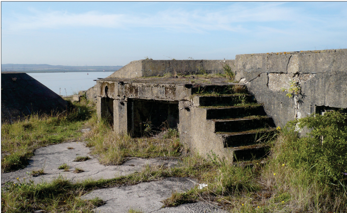
Figure 48: The most southerly of the surviving 12-pounder gun emplacements with ammunition lockers, steps to the gun floor and metal brackets for the guard rail visible at the rear of the emplacement. © Historic England
