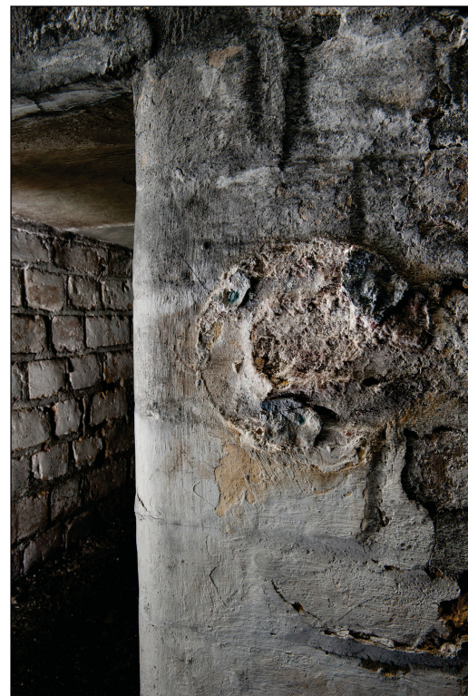
Figure 44: Lightbox to No 13 Cartridge Store showing the position of a copper number plate. (DP097434).
