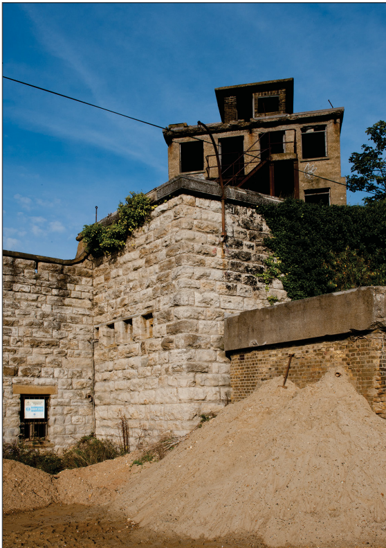
Figure 74: The external oil store located outside the north-east bastion. (DP097698)
