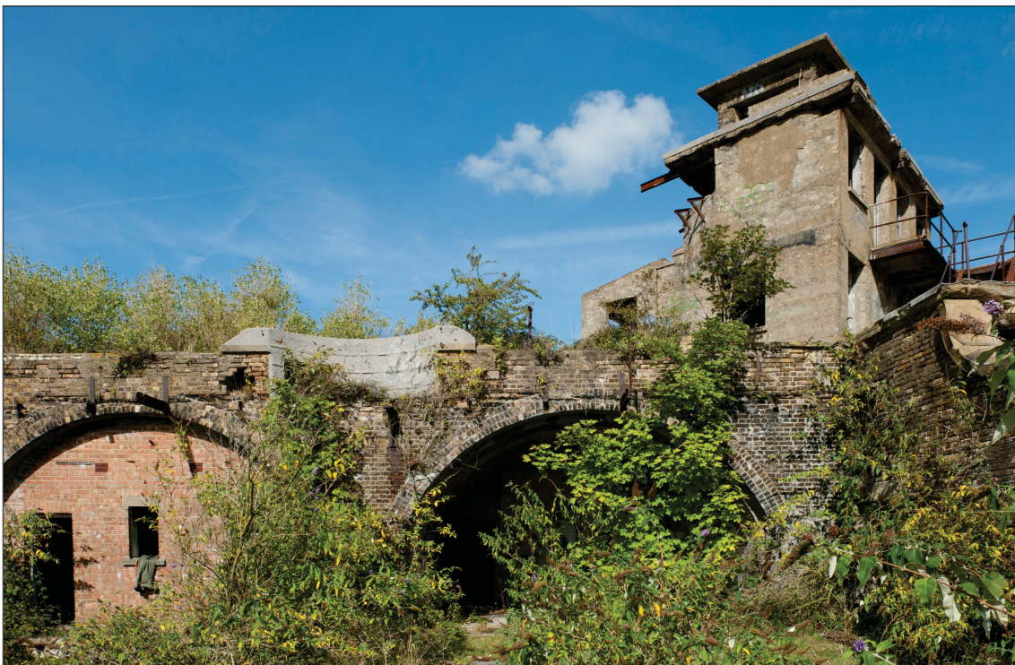
Figure 45: Exterior of Casemates 2 and 3 showing the semi-circular recess for the DRF position and the stanchions for its associated walkway set in the parapet wall above the casemates. The circa 1913 Battery Observation Post can be seen above. (DP 097568)
