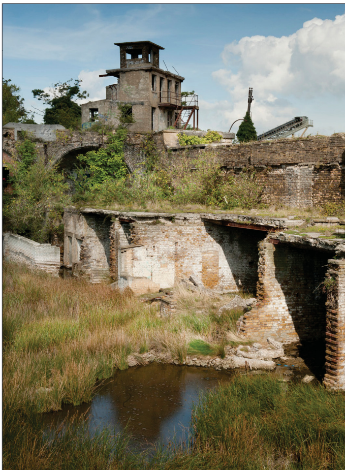
Figure 80: The north end of the East range. In the foreground are the remains of the Guard House and the cell block. Beyond them are the Ablutions and Latrines with their new front wall and the heavily weathered modesty wall in front. On the right hand side of the picture, the lighter coloured patch on the parapet wall is the position of the brick outbuilding to the demolished timber hut which extended from here to the left hand side of the frame. (DP097523)
