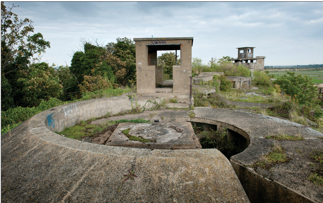
Figure 51: The western barbette of the 6-inch gun emplacements, the large concrete block (for mounting a Second World War 6-pounder gun) cast in the original gun pit can be seen in the centre of the photograph. (DP097671)
