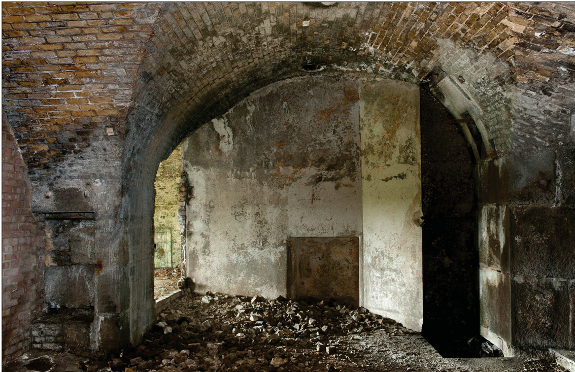
Figure 41: View from Casemate 2 west into Casemate 3 where the gun position has been filled with a concrete traverse and an ammunition recess created. (DP097588)
