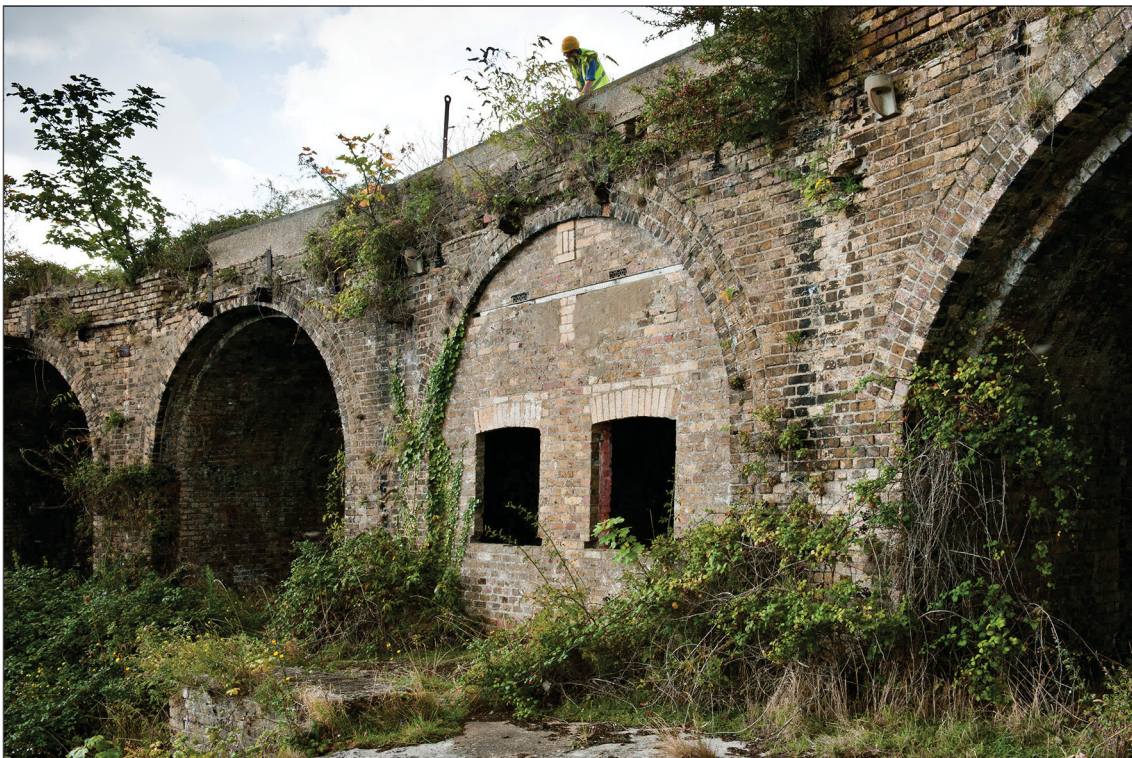
Figure 55: Casemate 6 was probably enclosed with a permanent brick wall at the time the 6-inch battery was built on the roof in order to provide a crew shelter. (DP097599)
