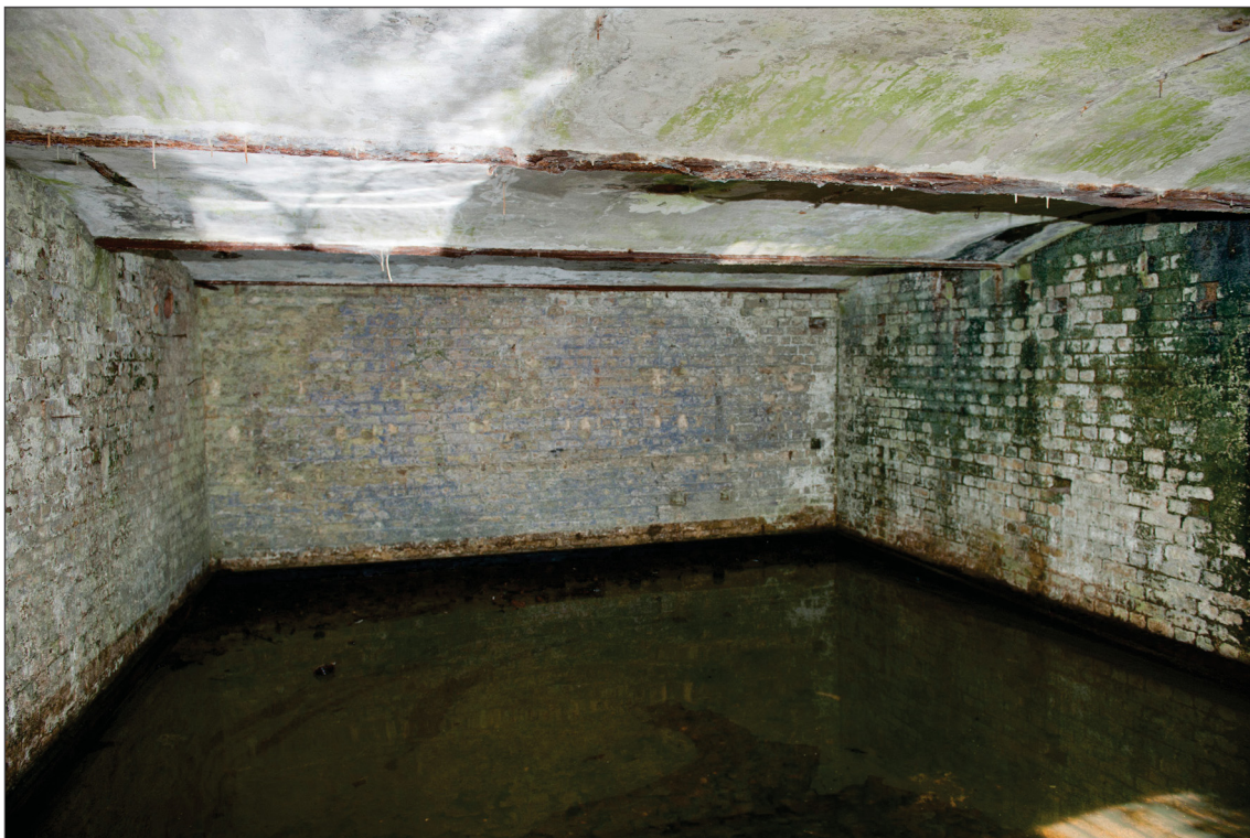
Figure 72: The interior of the Test Room [72] showing the vaulted roof and the various marks on the walls showing the positions of the connection boards and benches. (DP 097565)
