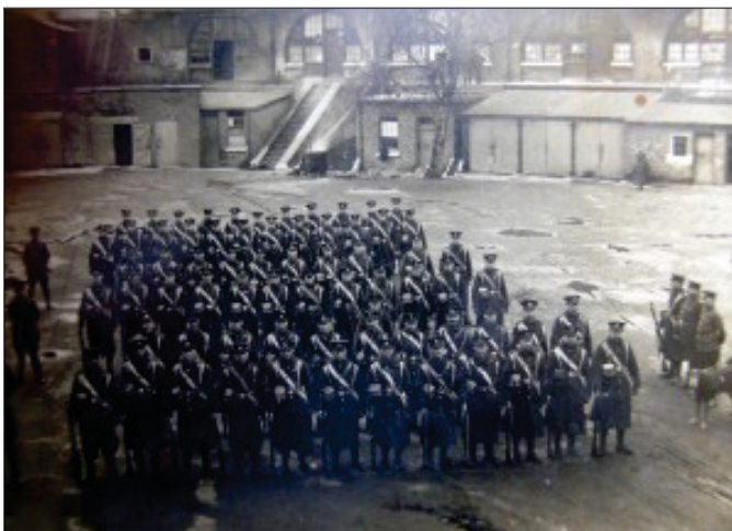
Figure 49: The parade ground dated circa 1915 by the equipment of the men on parade. Behind and to the right are the QF Gun Shed and the Stores RA and RE. To the left of the picture an open door, the entrance to the Brennan Torpedo installation, disused at this time, can be seen. Courtesy of Victor Smith
