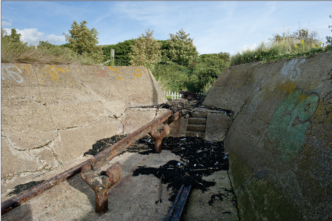
Figure 58: The north slipway and launching rail looking back towards the open battery of Cliffe Fort. The slots for the timber boards mentioned in the letter of 1889 are in the flanking walls above the short flight of steps. (DP097353)
