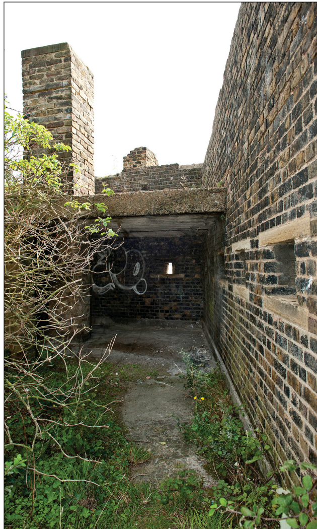
Figure 56: The probable First World War defensive position constructed in the south-east demi-bastion. (DP097579)
