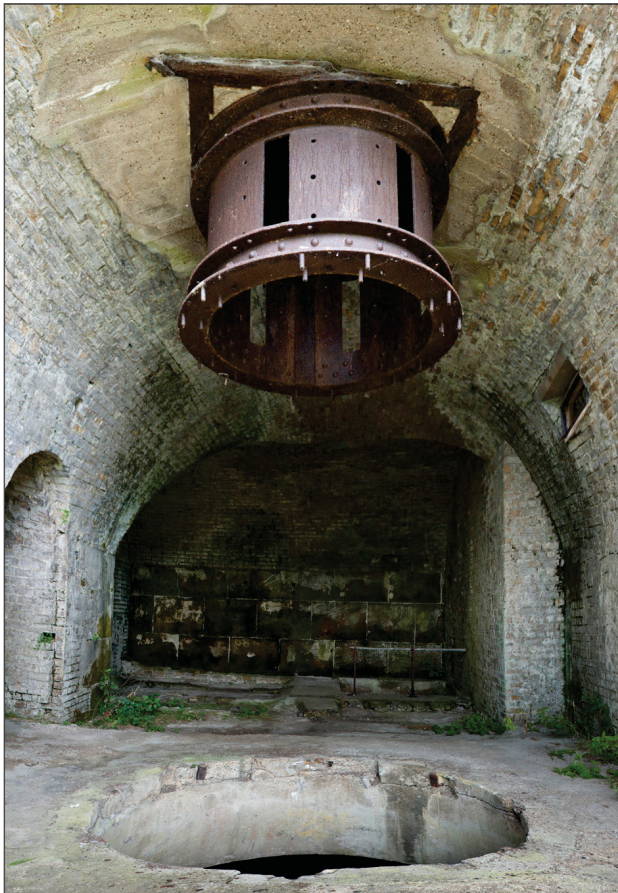
Figure 70: The interior of Casemate 15 looking west with the iron collar for the rising tower set in the vault. The corresponding hole visible in the floor opens into the former lighting passage and casemate below. On the right hand side of the photograph is the corner of the brick wall inserted to support the 6-pounder gun battery on the roof. The arched doorway on the left hand side of the picture leads to the former open gun positions. (DP097638)
