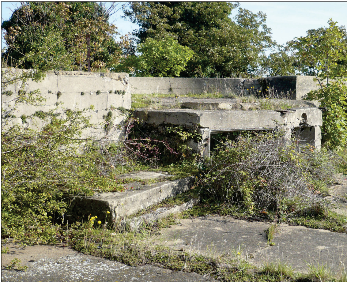
Figure 46: Shallow steps protruding from one of the flank walls of the 12-pounder battery which may represent the remains of an earlier rooftop battery © Historic England
