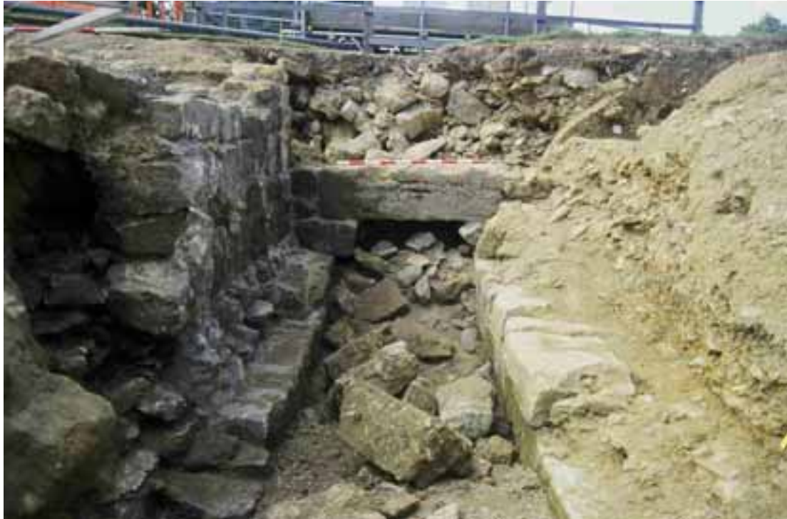
Figure 7: Excavated culvert (looking north-west), showing culvert walls [1052] (left) and [1051] (right), with re-pointed section of culvert wall [1053] on the left; modern rubble fill [1001] is in the centre (photo by D Stirk)
