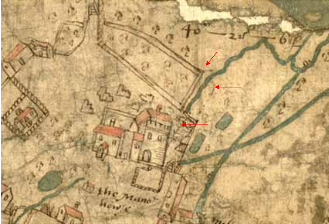
Figure 13: Detail from Treswell's 1587 map (MF/1/59, The National Archives UK), showing possible outline of former pond and line of culvert. North is to the left of the image
