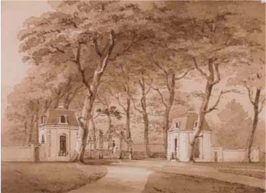
Figure 151 'The Silsoe Lodges' (Steve Cole © English Heritage DPI 10080, by permission of a descendant of Thomas, Earl de Grey)
