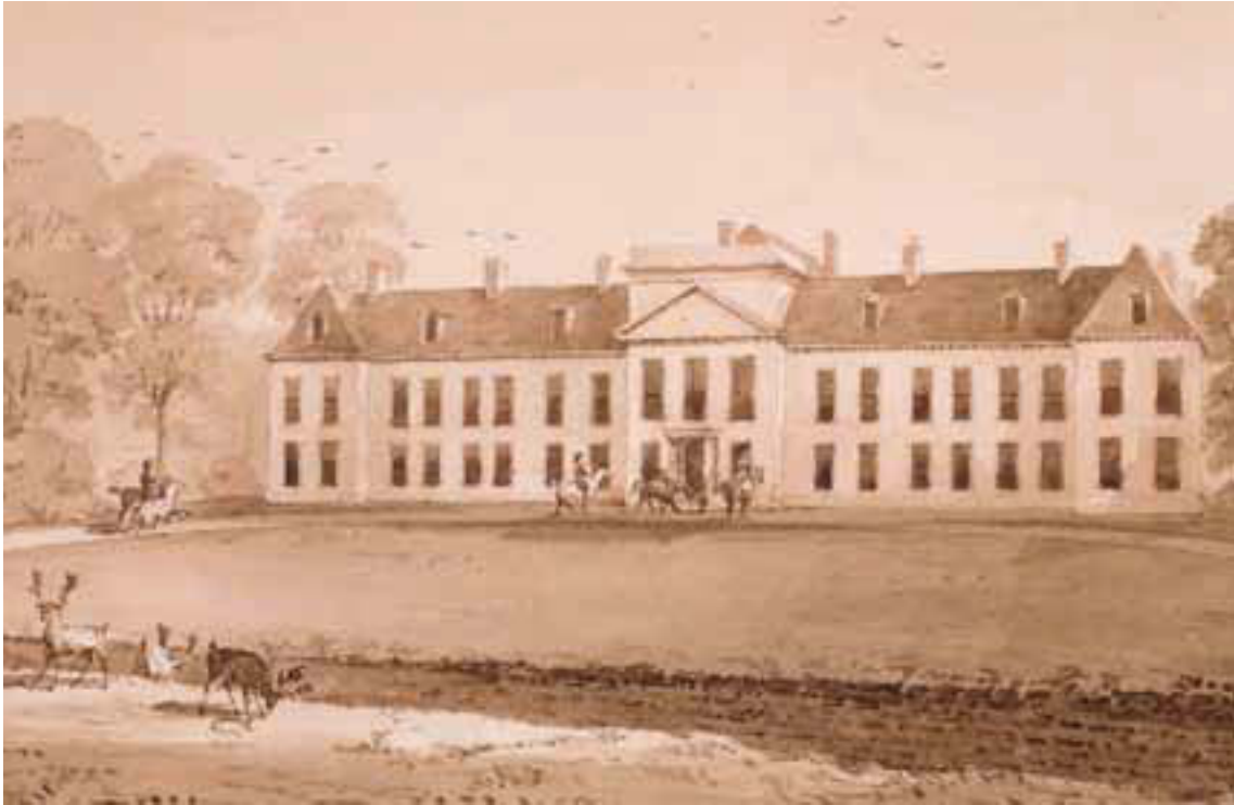
Figure 20 Sketch of the north front of the old house from the 1831 sketchbook (Steve Cole © English Heritage DPI 10020, by permission of a descendant of Thomas, Earl de Grey).
