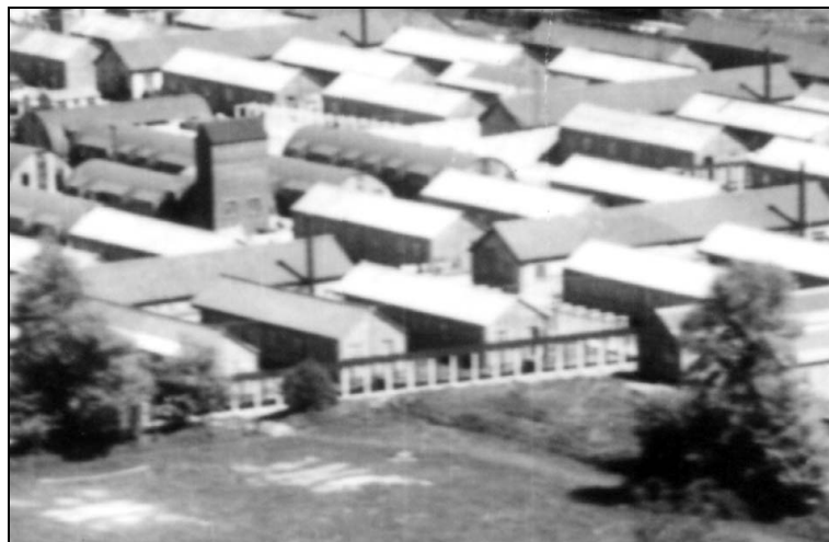
Figure 44 New buildings at Devizes barracks, part of the southern hospital (with rounded roofs and a wooden tower) connected to the existing barrack buildings (pitched roofs) by a network of covered walkways, in the foreground. Detail of US/31GR/LOC50 5125 30-April-1944. English Heritage USAAF Photography
