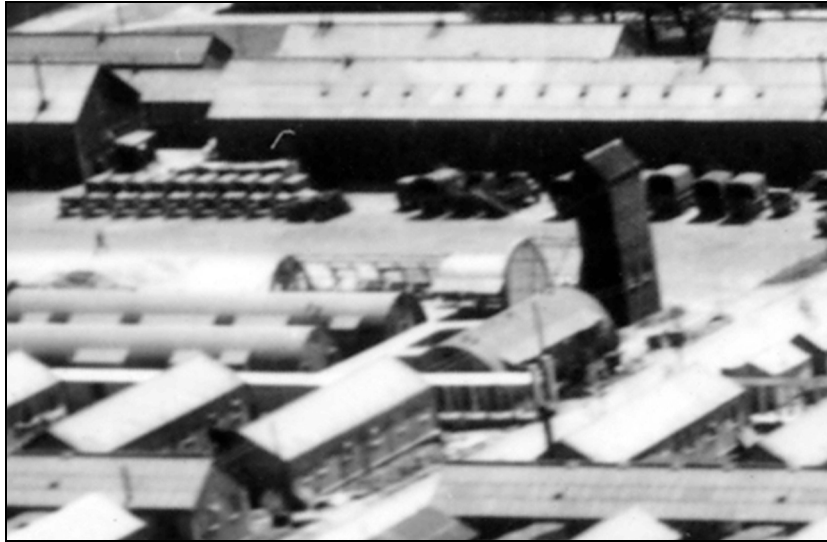
Figure 43 The framework is visible of a building under construction at Devizes Barracks. At the western end is a wooden tower. Detail of US/31GR/LOC50 5129 30-Apr-1944. English Heritage USAAF Photography
