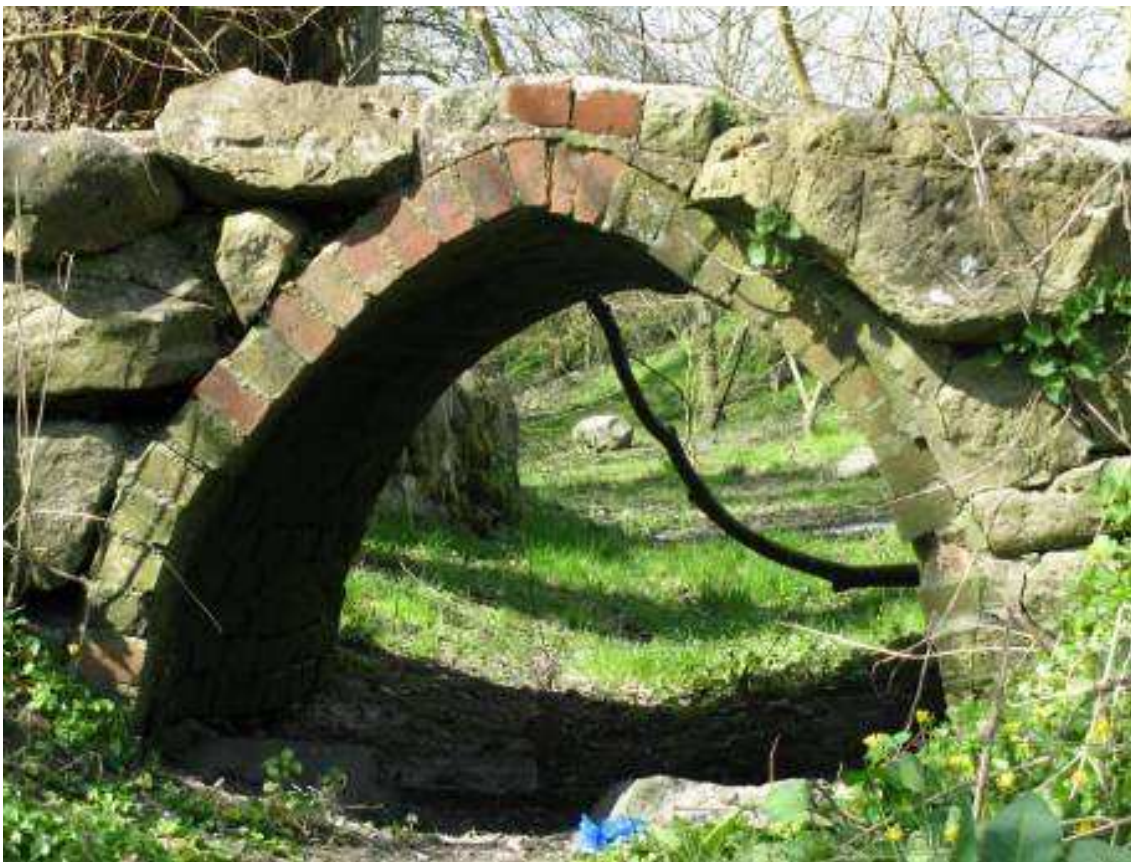
Figure 13: Dry stream bed at Avebury
