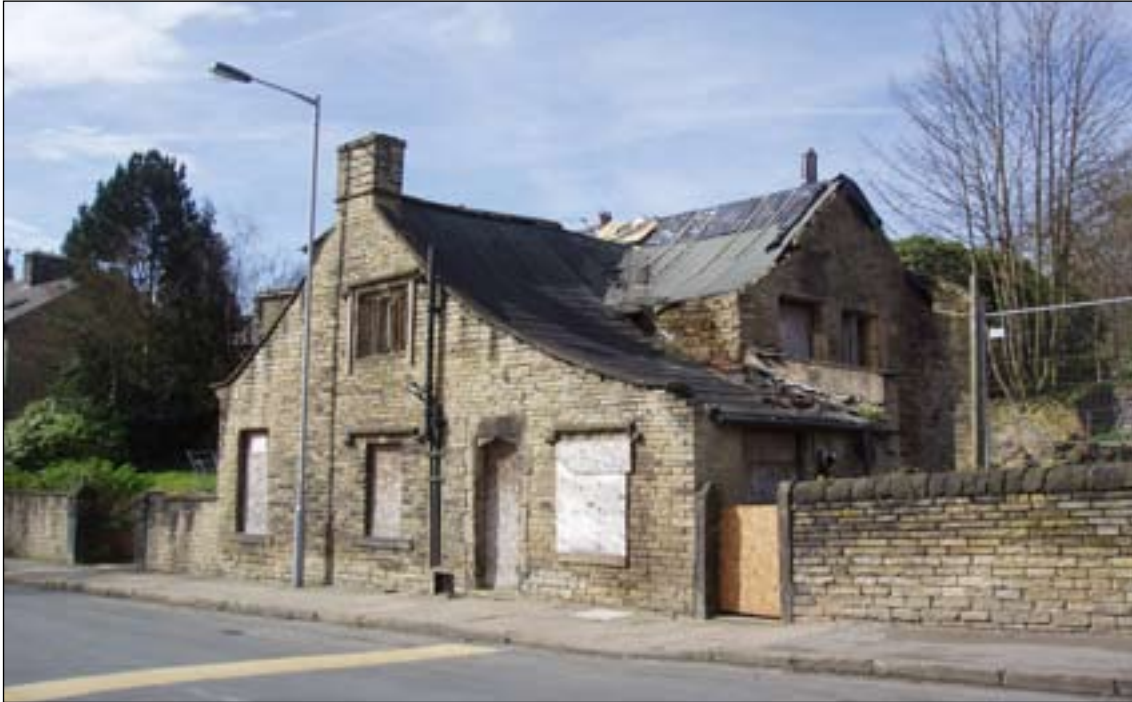
Fig 19: Old Manor House from north-east: the aisled structure of the medieval house was retained in the 17th century rebuilding in the area of the housebody: the roof sweeps down to single-storey height to both north and south (© English Heritage)
