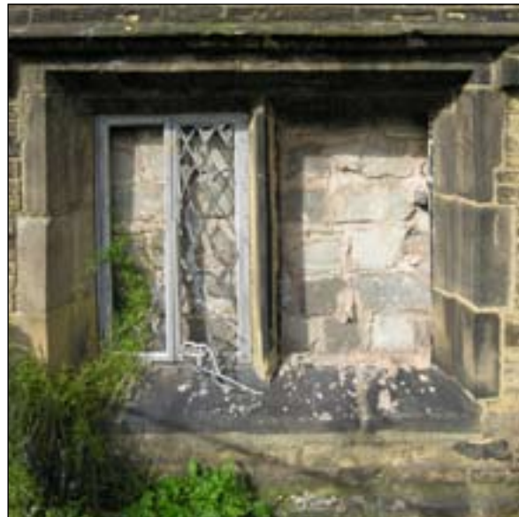
Fig 11: west wing, south wall: formerly mullioned and transomed window (© English Heritage)
