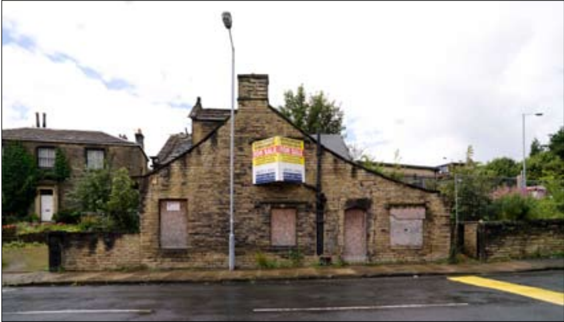
Fig 25: east wall, built on the truncation of the house c.1890 (DP065452 © English Heritage)
