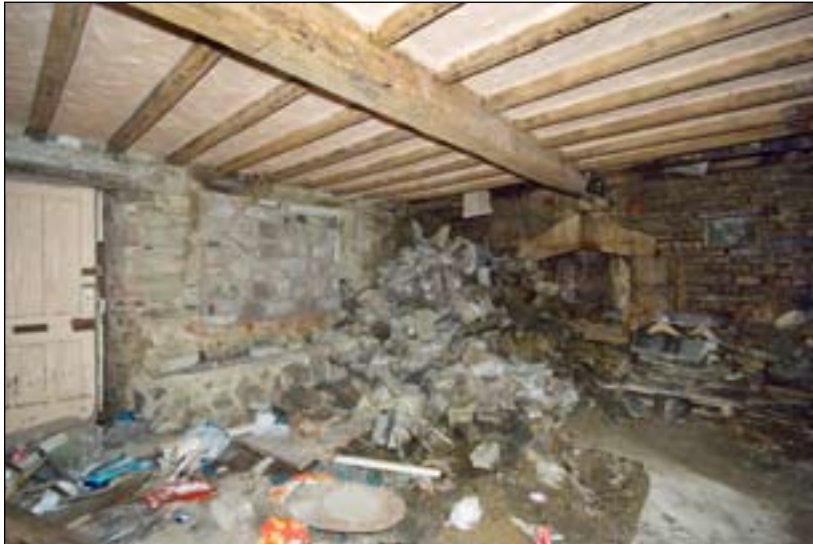
Fig 13: west wing, parlour, showing fireplace on west wall (DP071440 © English Heritage)
