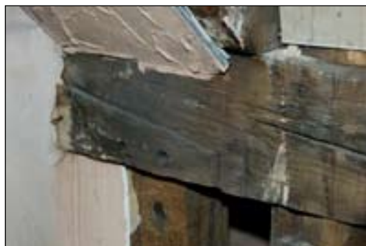
Fig 7: detail of scarf joint in arcade plate (DP071435 © English Heritage)
