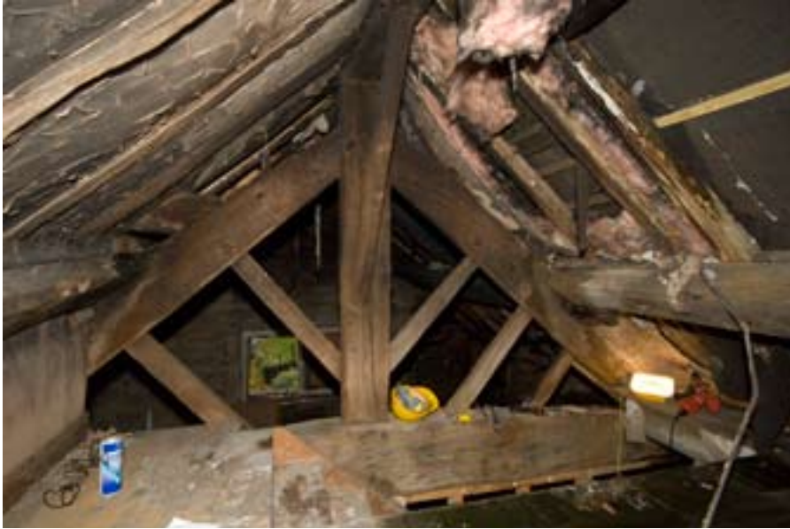
Fig 18: west wing, central roof truss, view from north (DP071455 © English Heritage)
