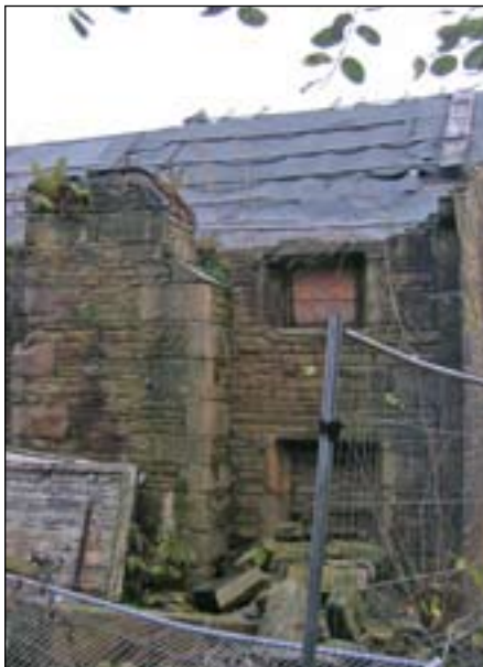
Fig 10: west wing, west wall, showing quoined masonry and external stack (© English Heritage)
