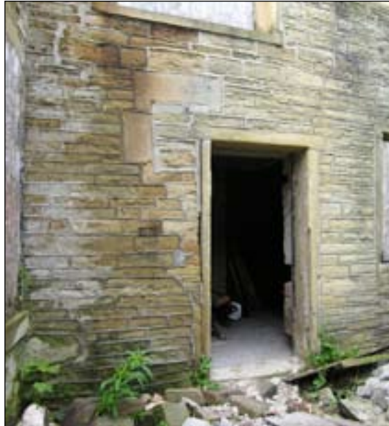
Fig 16: west wing, north wall, blocked raised window for original stair (© English Heritage)
