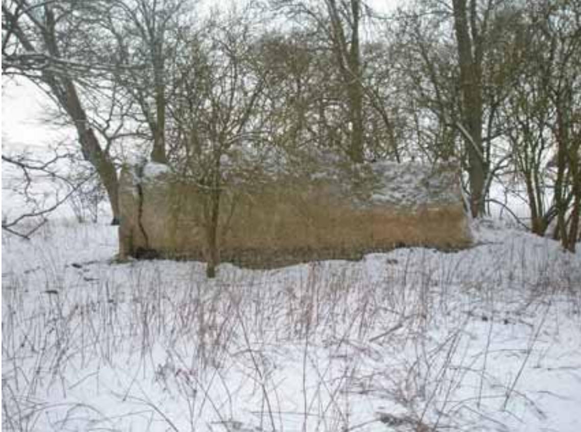
Fig 4: Remains of the well house in Spring Bottom south of Springbottom Farm, near Lake, built of cob and clunch with brick facings; the well house in Stonehenge Bottom to the south of the Cursus was probably similar.
