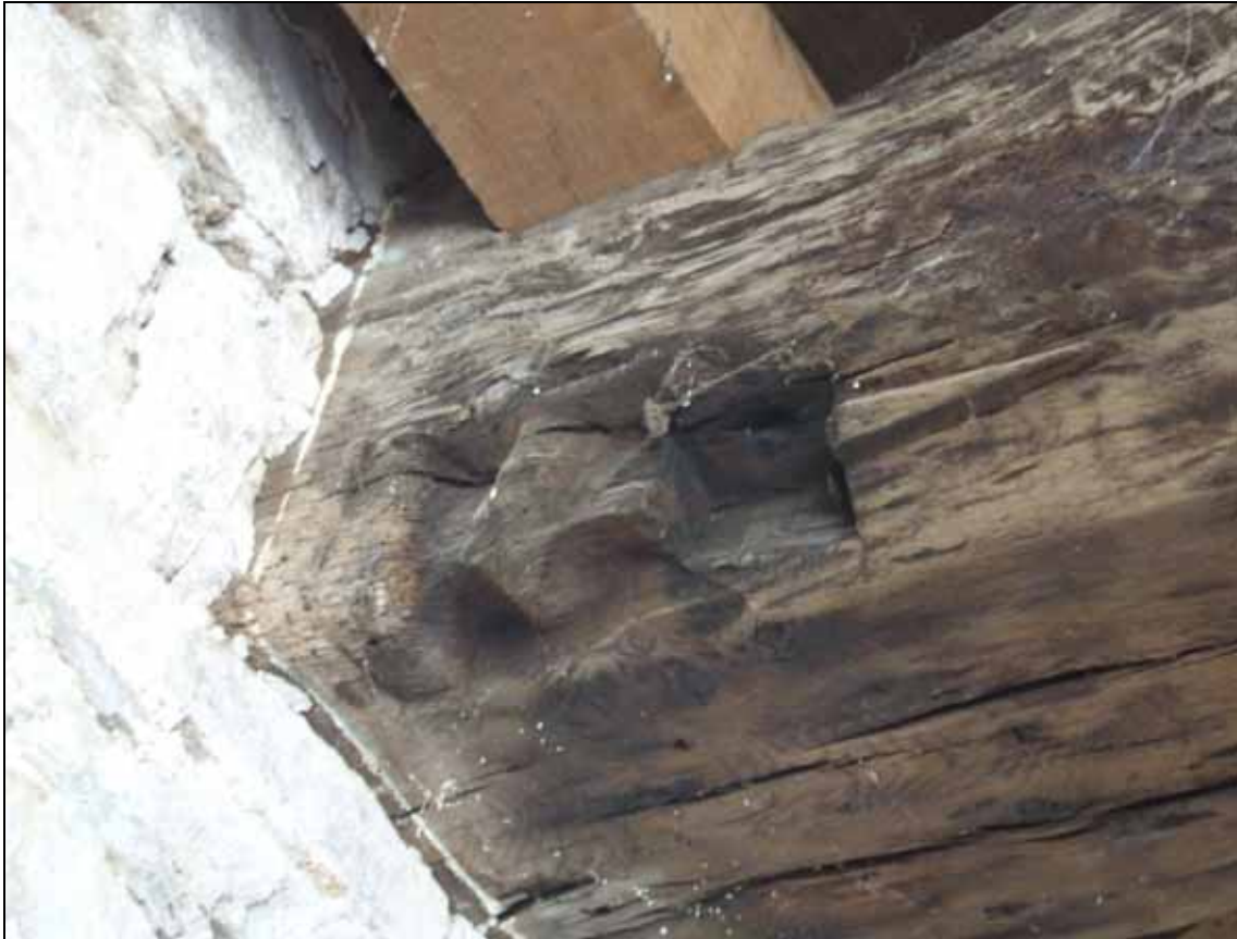
Figure 3: One of the elaborate chamfer-stops to the first-floor beams at Pengersick Castle. Photograph Martin Bridge
