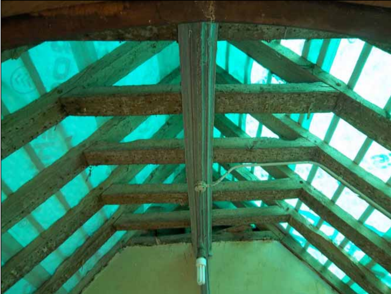
Figure 6: Porch roof (photograph taken from the south). Photograph Robert Howard
