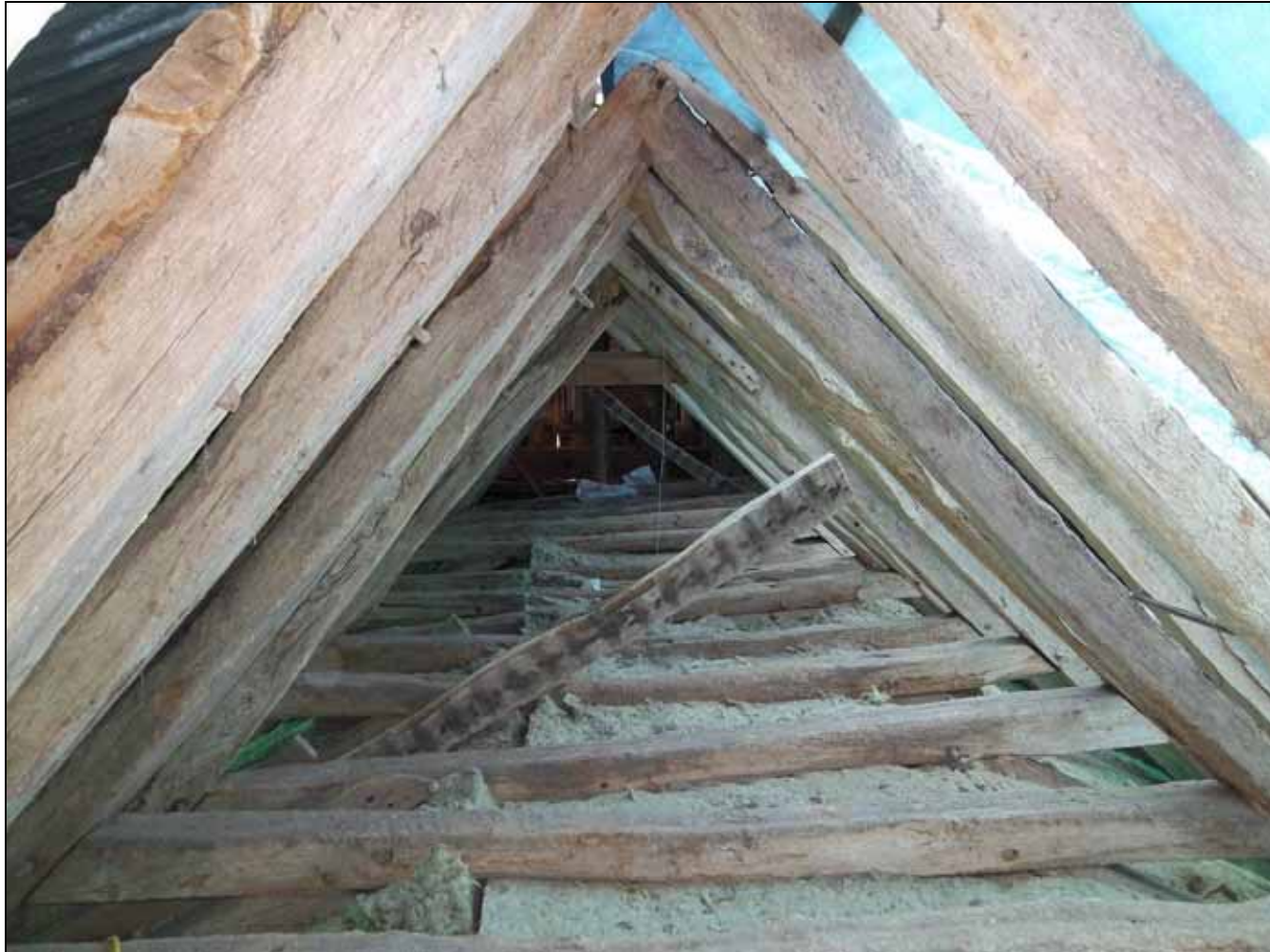
Figure 5: South aisle roof (photograph taken from the west). Photograph Robert Howard
