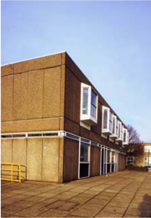
Figure 4.22: The CLASP Mark V elevations of the Chilwell lower school. © Elaine Harwood.
