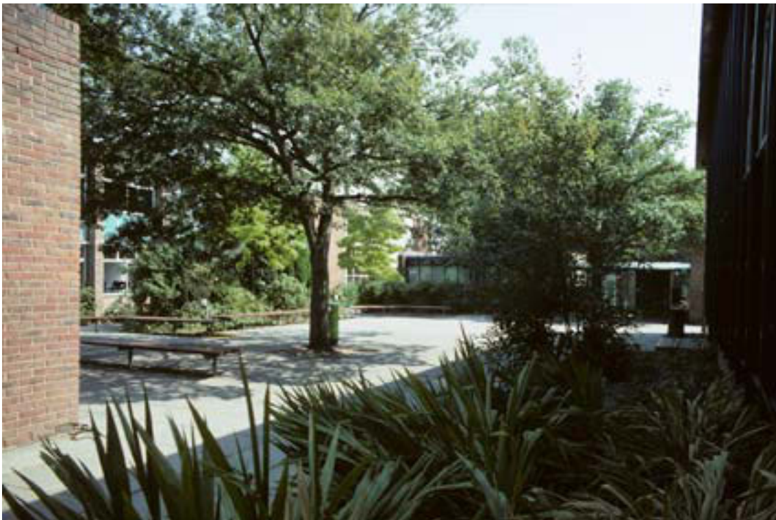
Figure 3.19: Additions of 1983-85 to the Hurst School in Tadley, Hampshire, by Aldington, Craig and Collinge. When the Hampshire county architect Colin Stansfield Smith commissioned the scheme, he cautioned Peter Aldington 'it's not a building scheme, it's a landscape scheme – don't you dare spend it on building!' (Powers 2009, 96). Photograph reproduced by kind permission of Peter Aldington.
