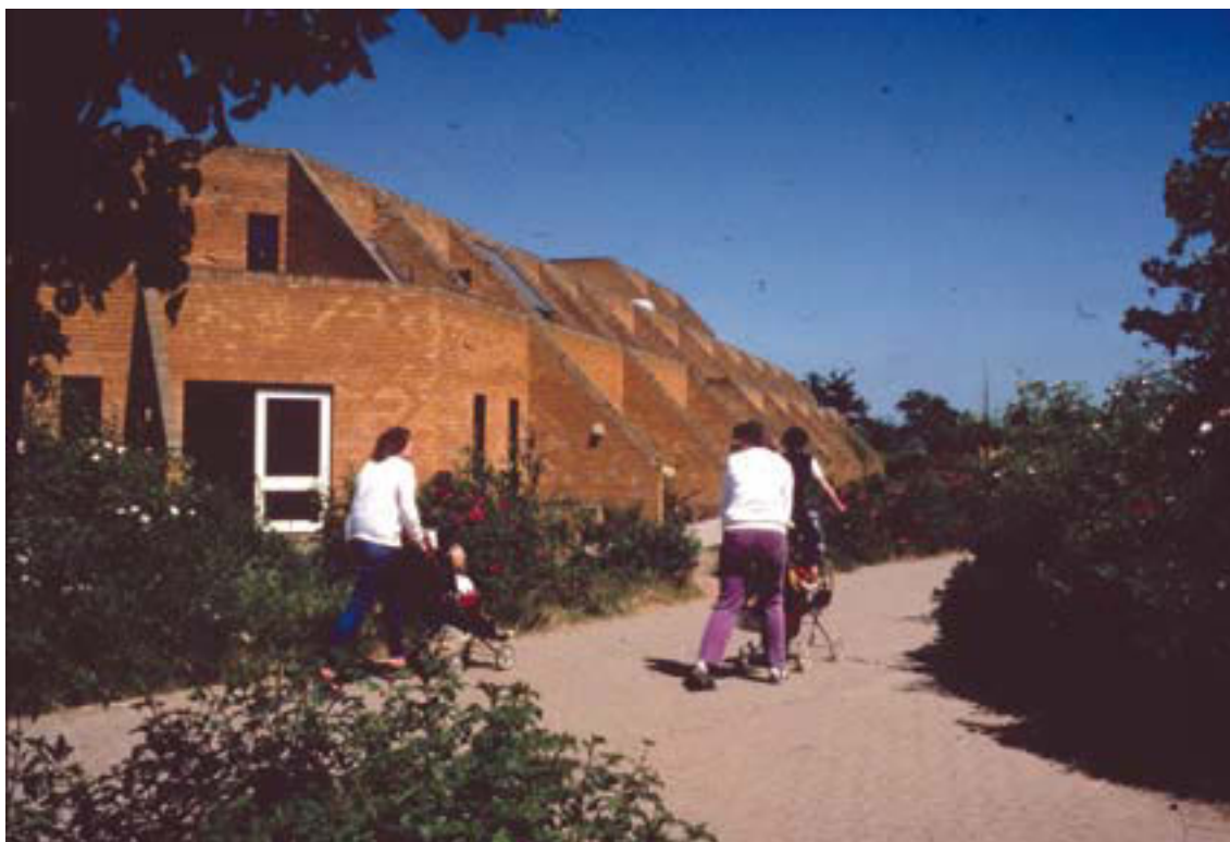
Figure 2.11: At the Cresset Centre, Peterborough (completed 1978, demolished c.2006) a sophisticated gradation was planned between exclusive and communal facilities, which allowed the Bretton Woods Comprehensive School its own site whilst pupils enjoyed use of the library and sports hall of the adjacent community centre, planned by the Peterborough Development Corporation. 156 See also fig. 1.2. Institute of Education Archives: ME/E/19/18.
