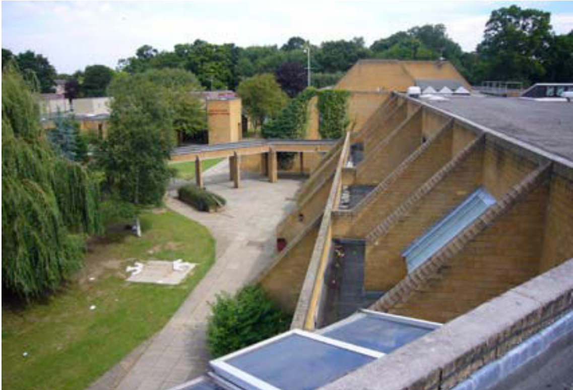
Figure 1.2: The Bretton Woods Community School opened in 1977 to serve the first of Peterborough's new townships, Bretton, begun in 1970. Community facilities were shared with the adjoining Cresset Centre. The snaking teaching block, designed by Ken Matthews and Stuart Denham of Cambridgeshire County Council, included a set-back upper floor which, together with the sloping cross walls, created a ziggurat effect. The school's demolition in 2007, after an unsuccessful attempt to list the building, highlighted the need for more research into later twentieth-century school buildings. Patricia Roberts – © English Heritage.
