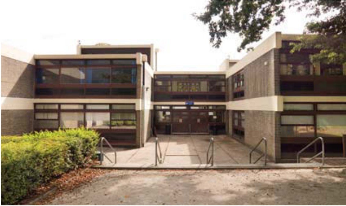
Figure 3.12: The main entrance to Lilian Baylis Secondary School, LB Lambeth; Architects' Co-Partnership, 1960-64. Photograph by James O. Davies – English Heritage; DP031012.
