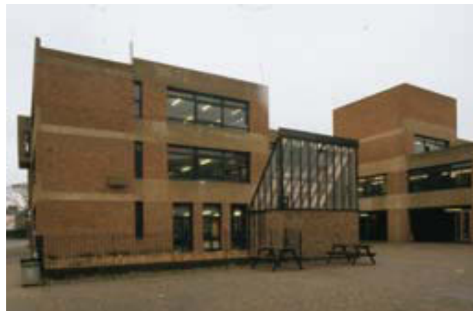
Figure 3.11: Stillman & Eastwick-Field received more commissions for London schools than any other firm. The finest of these was Stoke Newington Secondary School, Clissold Road, LB Hackney, built in 1967-70 to the designs of job architects Ralf Smorzewski, Denis McCoy and Michael Plunkett. It was remodelled with a cor-ten steel facade by Jestico + Whiles in 2009-10. 71 © Elain Harwood.
