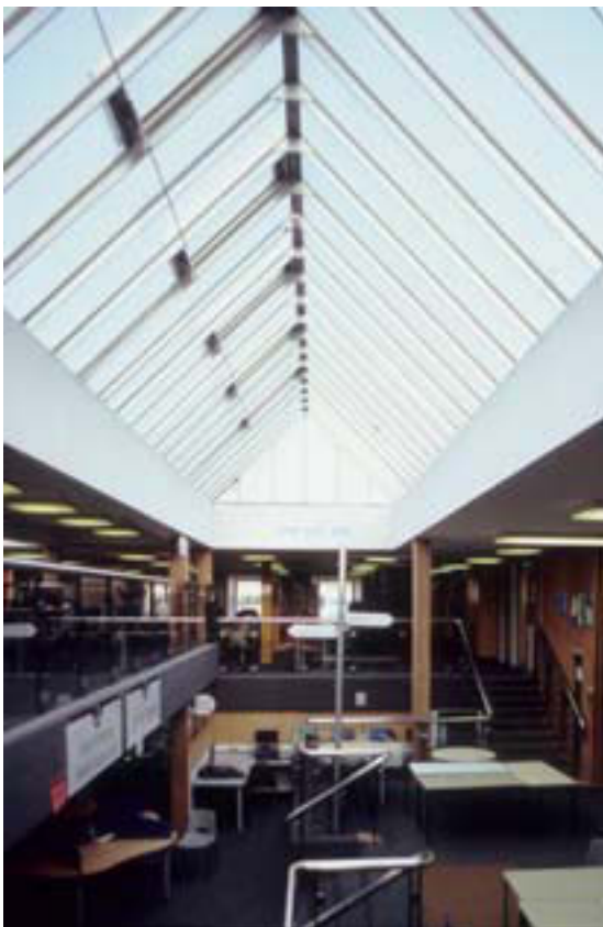
Figure 4.34: The lower school at Chilwell, added in 1975-76. The glass roof brings light into the very deep plan. © Elain Harwood.
