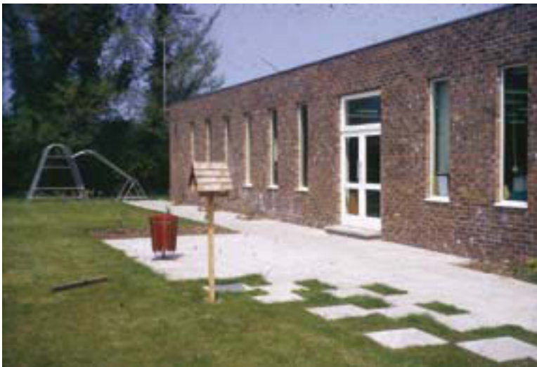
Figure 3.15: The 1970s saw a reduction in the glazed area of many schools. Eastergate School, seen here shortly after completion, was criticised by DES architects for its separation of ‘inside’ and ‘outside’: there were no verandas or opening windows. Institute of Education Archives: ME/2/5/2/179
