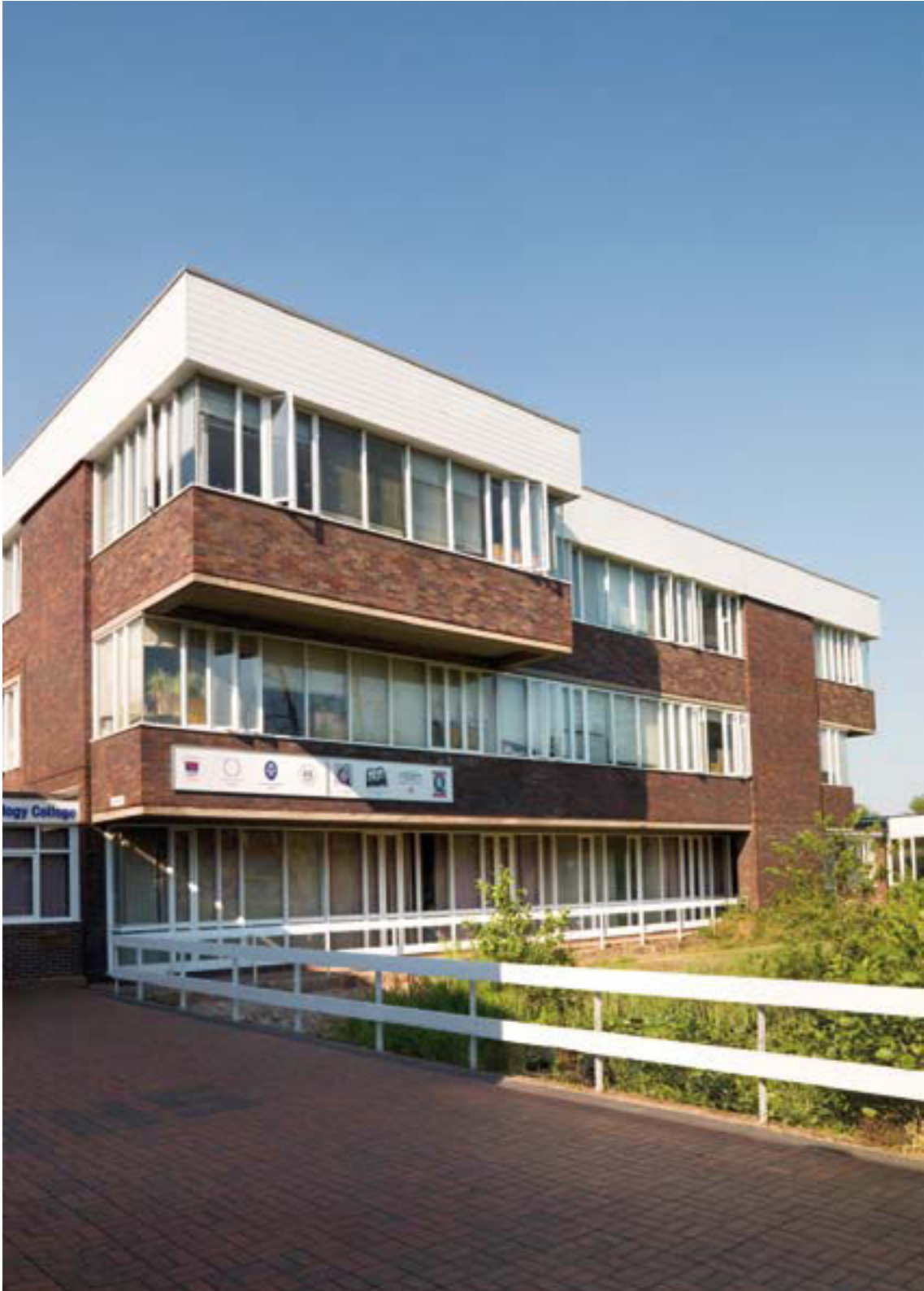
Figure 3.8: A complex rhythm of window mullions at South Bromsgrove High School, Bromsgrove; Richard Sheppard, Robson & Partners, 1968. Photograph by James O. Davies – English Heritage; DP030985.
