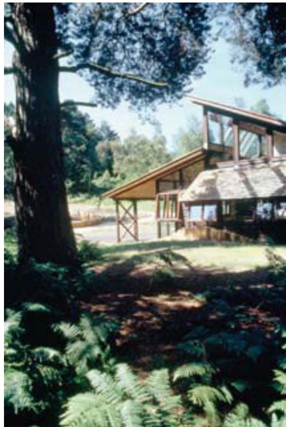
Figure 3.13: Woodlea Primary School, Whitehill; Hampshire County Council Architect's Department, 1990-91. The Rousseauian image of a 'school in the woods' is a recurrent one: the German Waldschulen (forest schools) appealed to the Edwardian builders of open-air schools, and Mary Medd (née Crowley) was inspired by similar schools in pre-war Sweden. Photograph kindly supplied by Nev Churcher.
