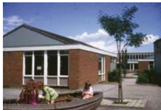
Figure 4.6: A 1971 view of Eveline Lowe Nursery and Primary School, Southwark; DES Development Group, 1965-66. Institute of Education Archives: ME/Z/5/2/86.
