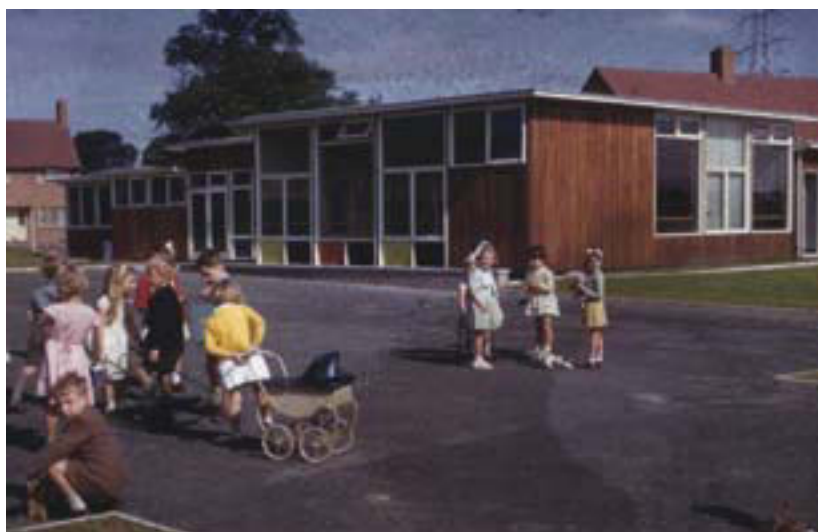
Figure 3.3: Hawkesley Farm Infant and Nursery School in Birmingham, an early 'Derwent' building. Institute of Education Archives: ABB/B/1/28/11.
