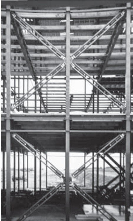
Figure 4.17 (left): Toot Hill School, Bingham, under construction c.1965. The spring-loaded bracing was unique to CLASP. Reproduced by kind permission of Nottinghamshire Archives.
