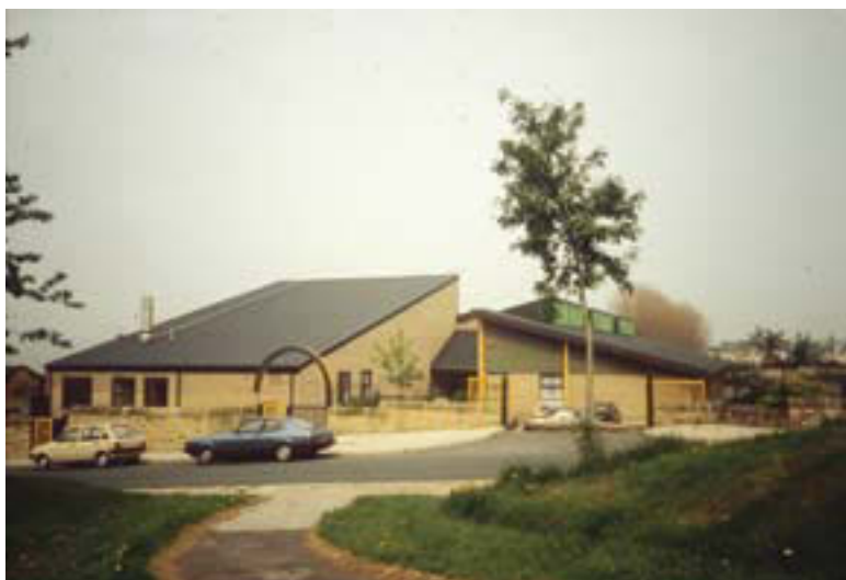
Figure 4.43: Newby First School, Bowling, Bradford; City Architect's Department (job architect Ron Furniss), 1985. The 'Bradford Schools Programme' involved several new schools of similar design. Institute of Education Archives: ABB/B/1/52/6
