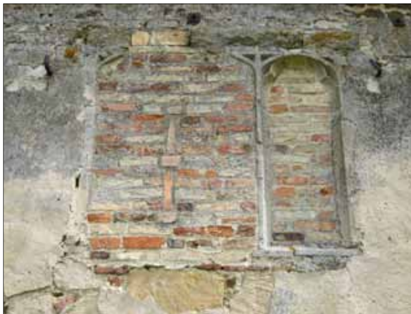
Figure 7. Blocked three-light window at upper level on west façade.
