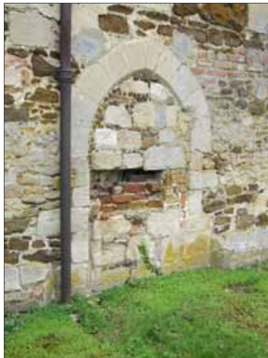
Figure 8. Infilled doorway on west façade.
