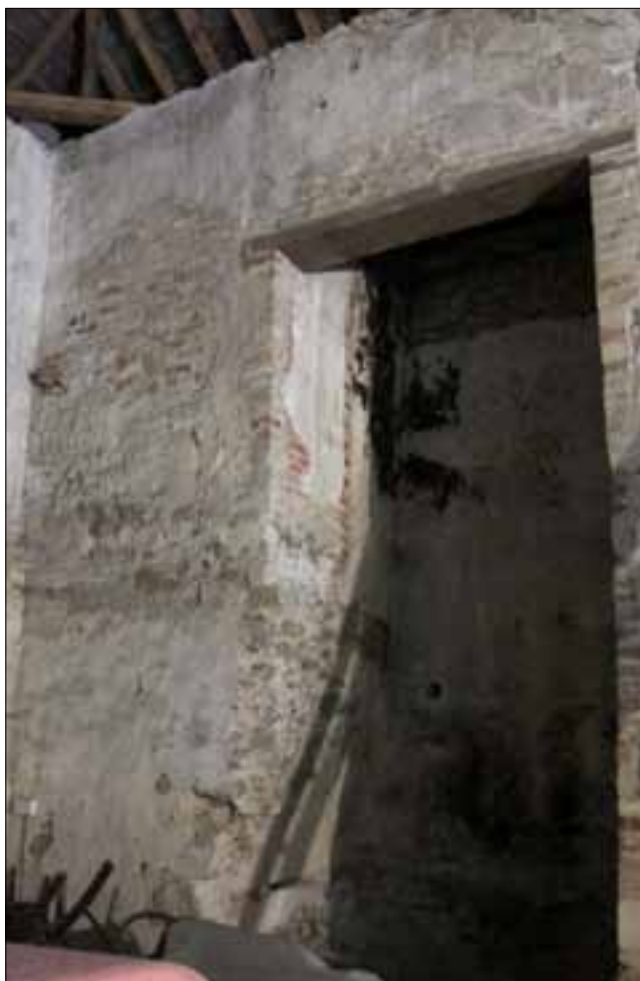
Figure 13. West wall, wing, interior.
