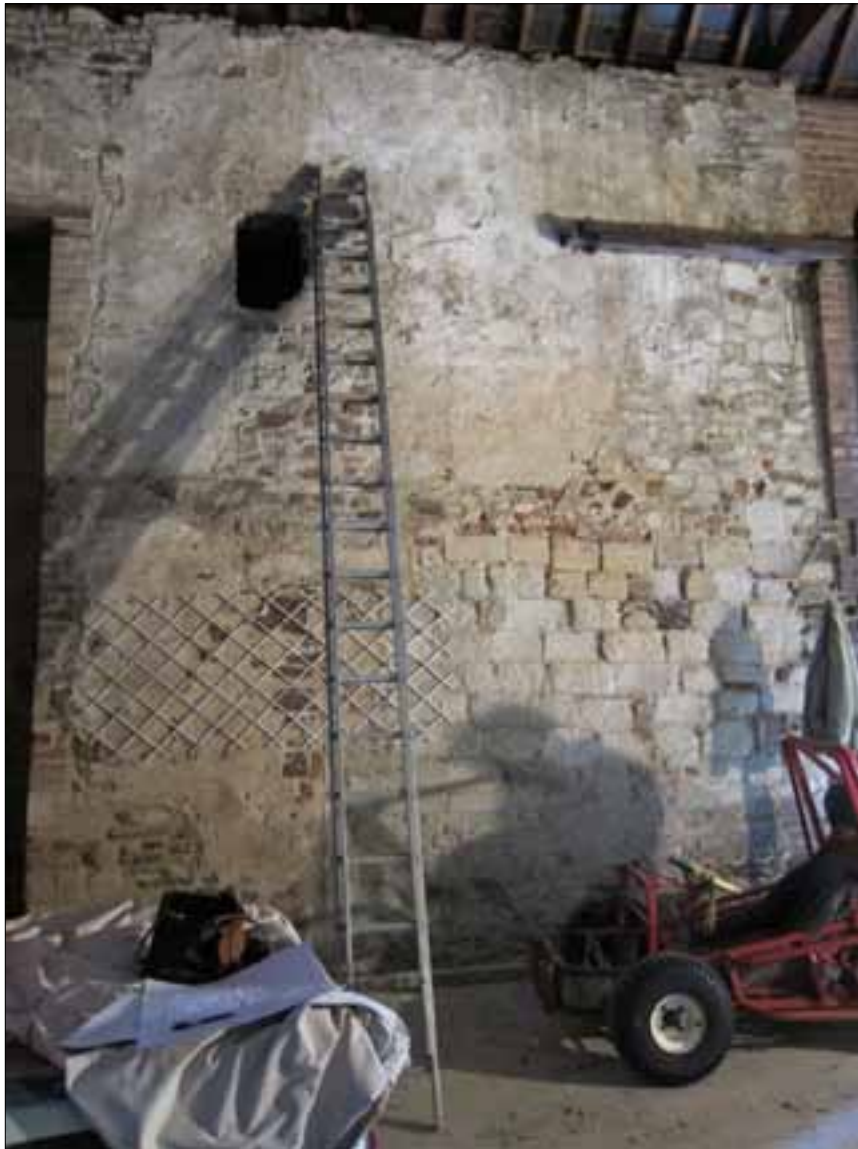
Figure 12. West wall, interior, where external features are not expressed internally.
