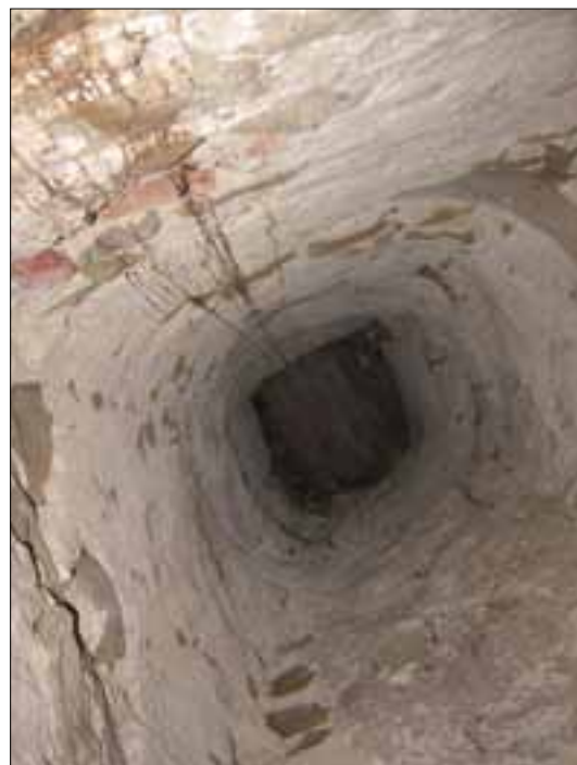
Figure 14. Probable garderobe chute in wall thickness of wing.
