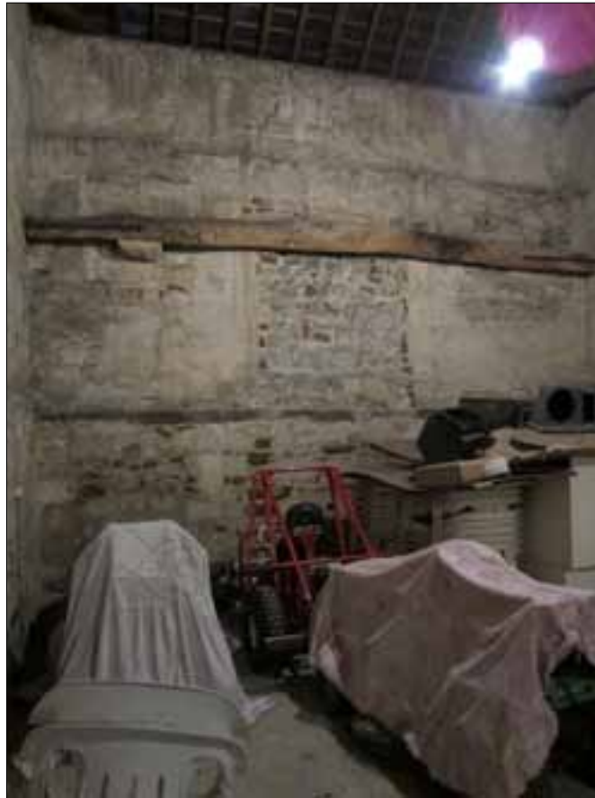
Figure 3. North wall, interior, showing evidence of earlier openings.
