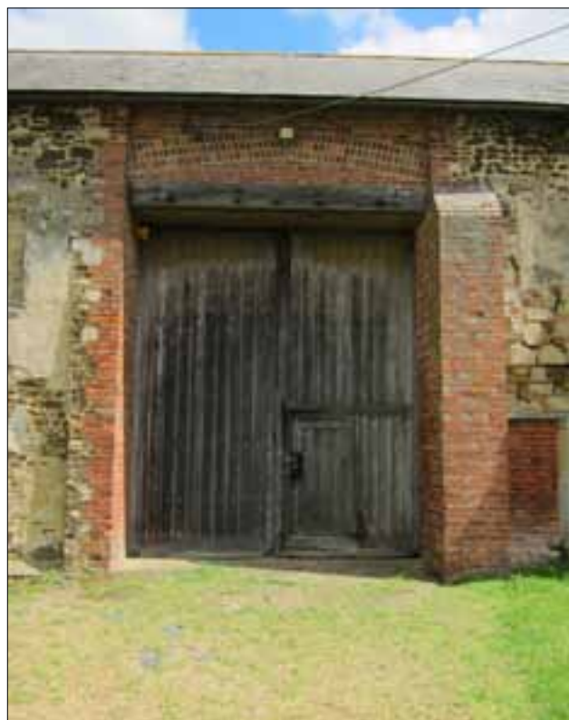
Figure 10. Taking-in door, west façade.
