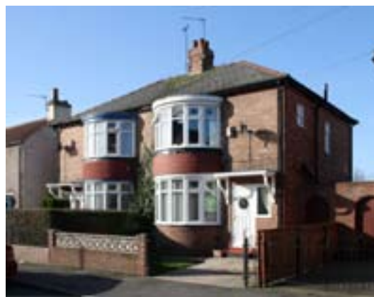
Figure 37 Nos 20-22 Cobden Street an example of inter-war development (P5924020)
