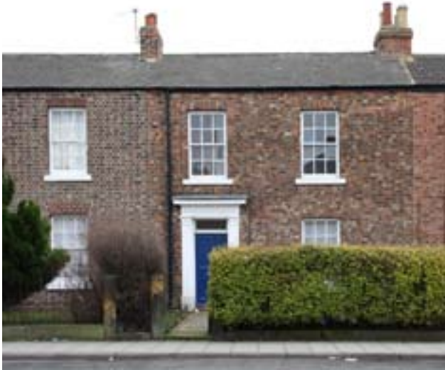
Figure 71 No. 142 Yarm Road, one of the two listed buildings in the estate. (P5924040)
