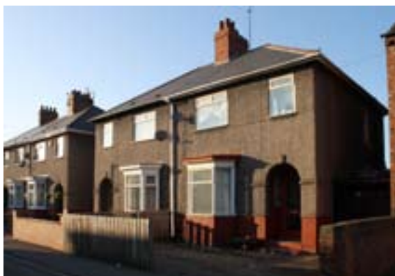
Figure 36 Nos 7-9 Pease Street, an example of inter-war development (P5924019)
