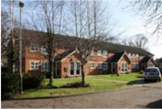
Figure 63 The recent development at Cobden Court with 'picturesque' detailing (P5924037)
