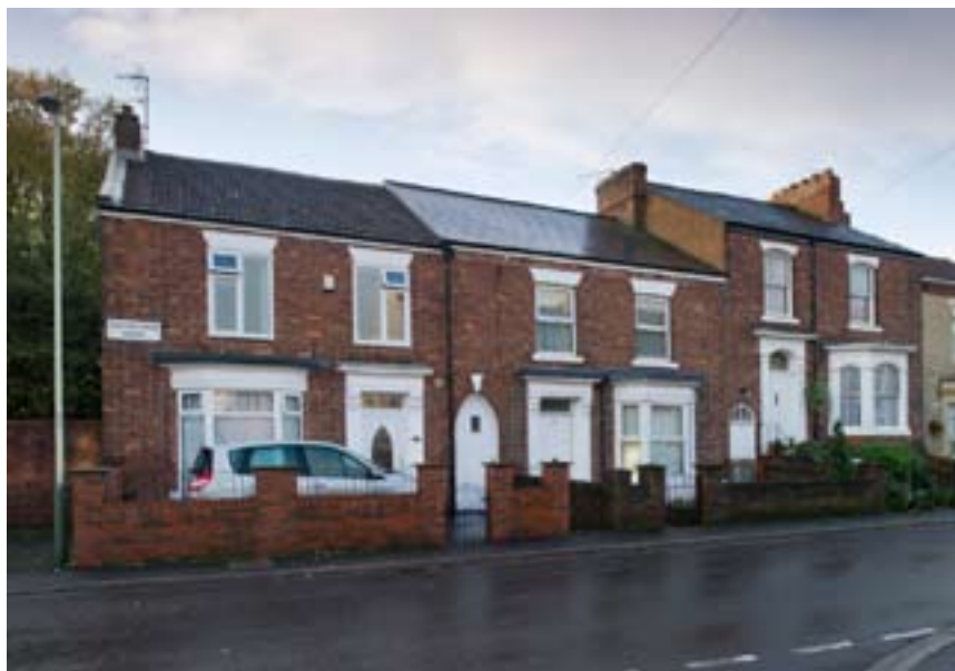
Figure 64 Nos 86-120 Eastbourne Road (DPI43806)
