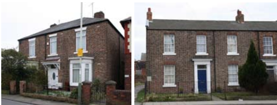
Figures 23 (left) No. 156 Eastbourne Road; an example of detached house of the 1860s or 1870s, later subdivided into two properties (P5924008) and 24 (right) No. 154 Yarm Road, built between 1851 and 1854 (listed Grade II) (DPI43799)
