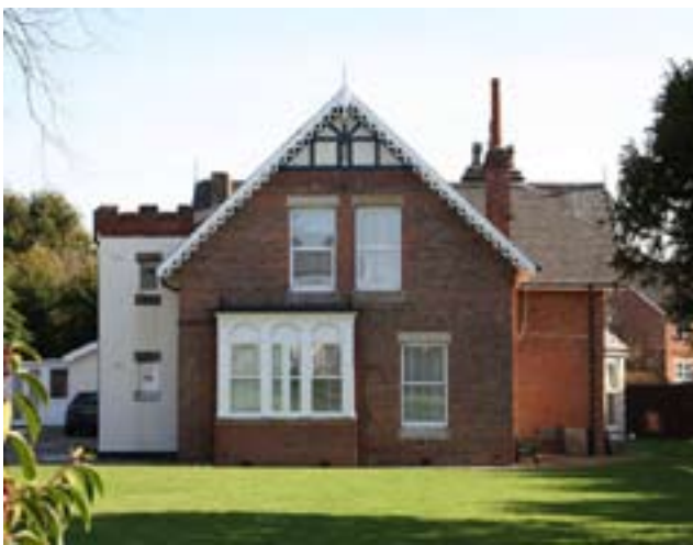
Figure 29 No. 79 Cobden Street, the best preserved example of a back-plot, more rustic style of house (P5924013)
