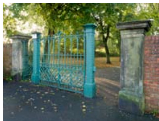
Figure 55 Eastbourne Park entrance (DPI43808)
