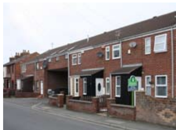
Figure 17 Nos 139-149 Eastbourne Road are post-war replacements for an extremely modest group of four late-19th century houses (P5924007)
