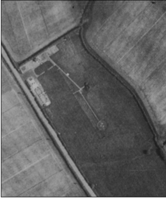
Fig 20: A radar directed searchlight battery near Meaux Abbey Farm. NMR RAF/106G/LA/212 4152 13-APR-1945 English Heritage (NMR) RAF Photography.
