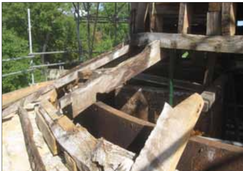
Fig 24 One of the principal rafters to the 'skirt', notched over the rim of the early 20th-century water tank.
