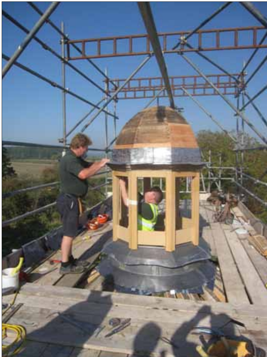
Fig 27 Reinstatement of the lantern and cupola
