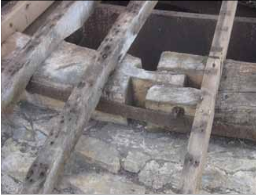
Fig 25 Joint to the wallplate, with dovetailed bridle, and failed forelock bolt fixing. The outer iron strap has been to provide restraint, after the original joint pulled apart.
