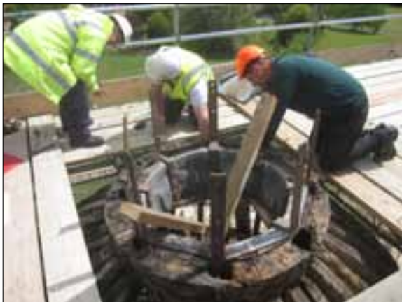
Fig 9 The two ring-beams after removal of the lantern. Note the iron straps which supported the eight posts of the lantern. These are applied over the internal lead flashing, which provided protection to the timber before the lantern was glazed.
