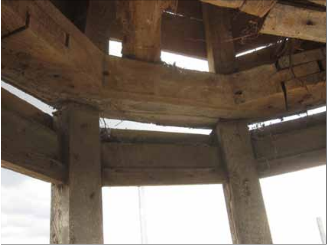
Fig 7 The base of the cupola, with octagonal base plate.
