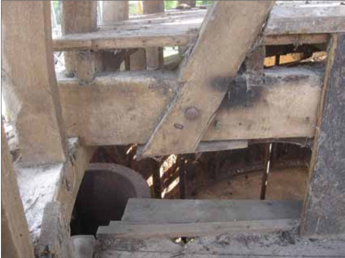
Fig 21 Detail of the joint to dome principal rafter and tie-beam, with lap dovetail, forelock bolt and large-head nail.
