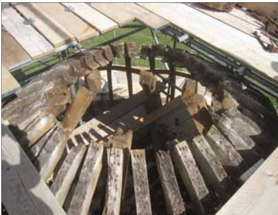
Fig 14 The tops of the main dome ribs, after removal of the ring-beams. The tops of the four straight principal rafters can also be seen.
