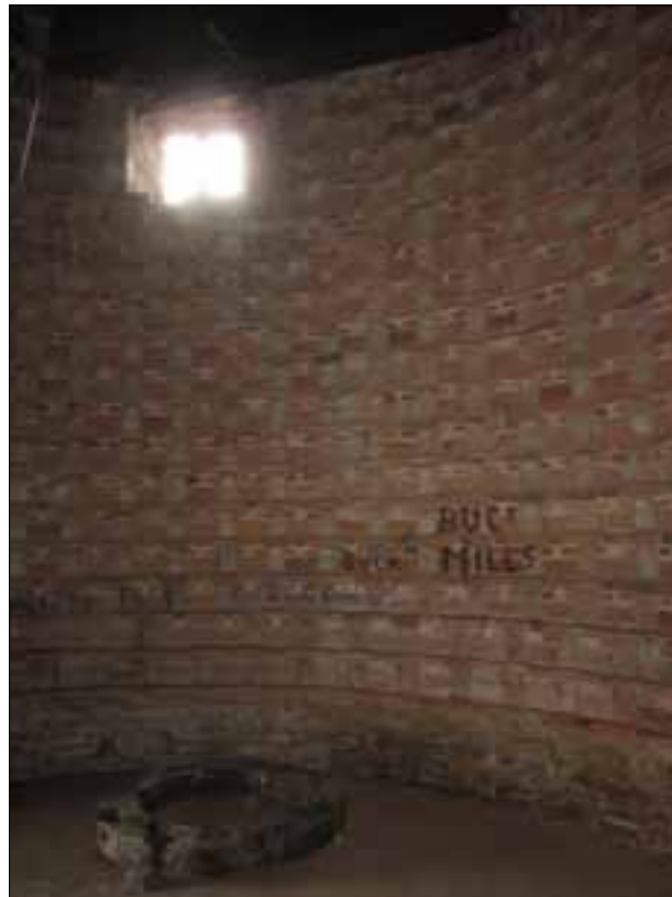
Fig 4 The interior of the Dovecote, with bricked-up nesting boxes.
