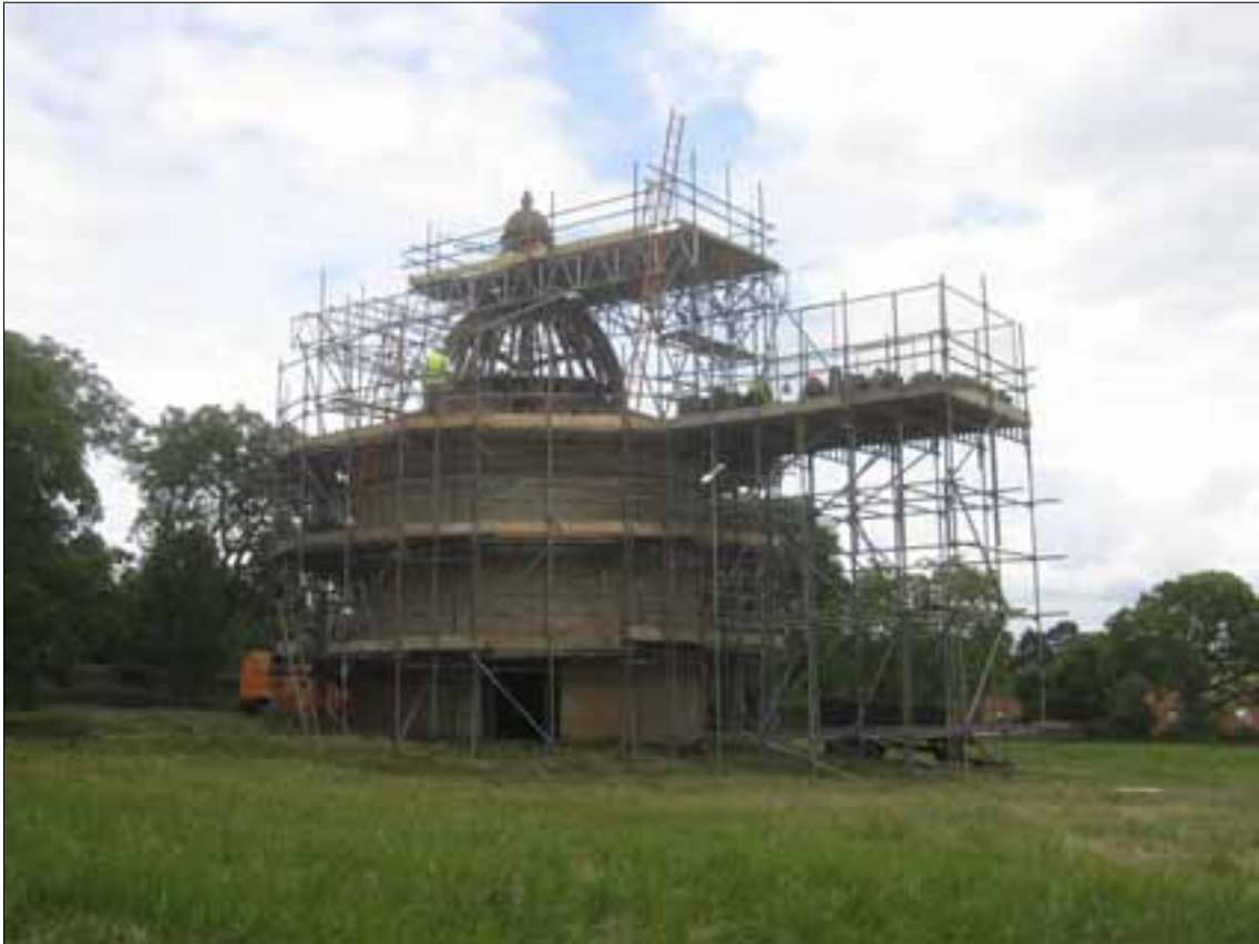
Fig 2 Works in progress, with roof covering stripped, June 2011.
