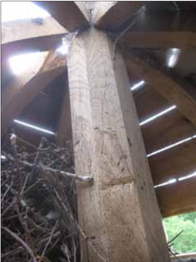
Fig 7 The base of the cupola, with octagonal base plate.
