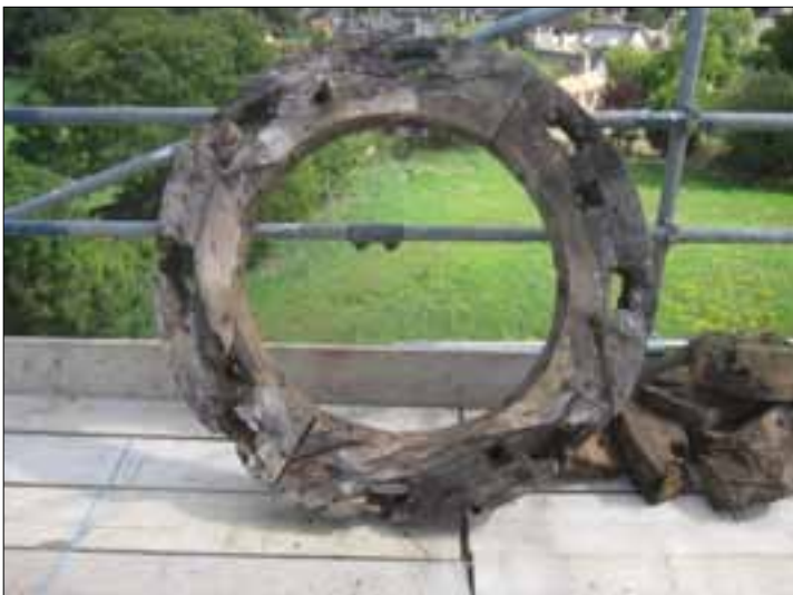
Fig 12 The upper ring-beam, formed in four sections. Note the eight decayed mortices for the Glover posts, and the four holes for forelock bolts, with square countersinking.
