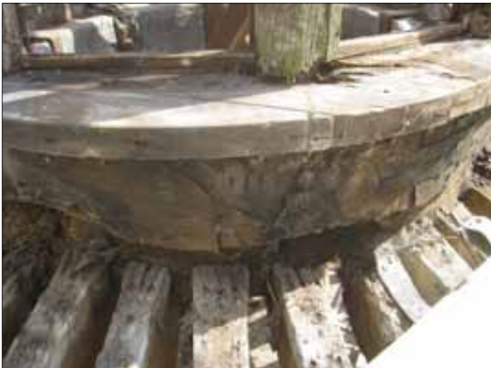
Fig 11 Detail of the upper ring-beam, with early 20th-century applied softwood cill, carpenter's mark 'IIII' and oak peg which fixed the tenon of the original Glover post.
