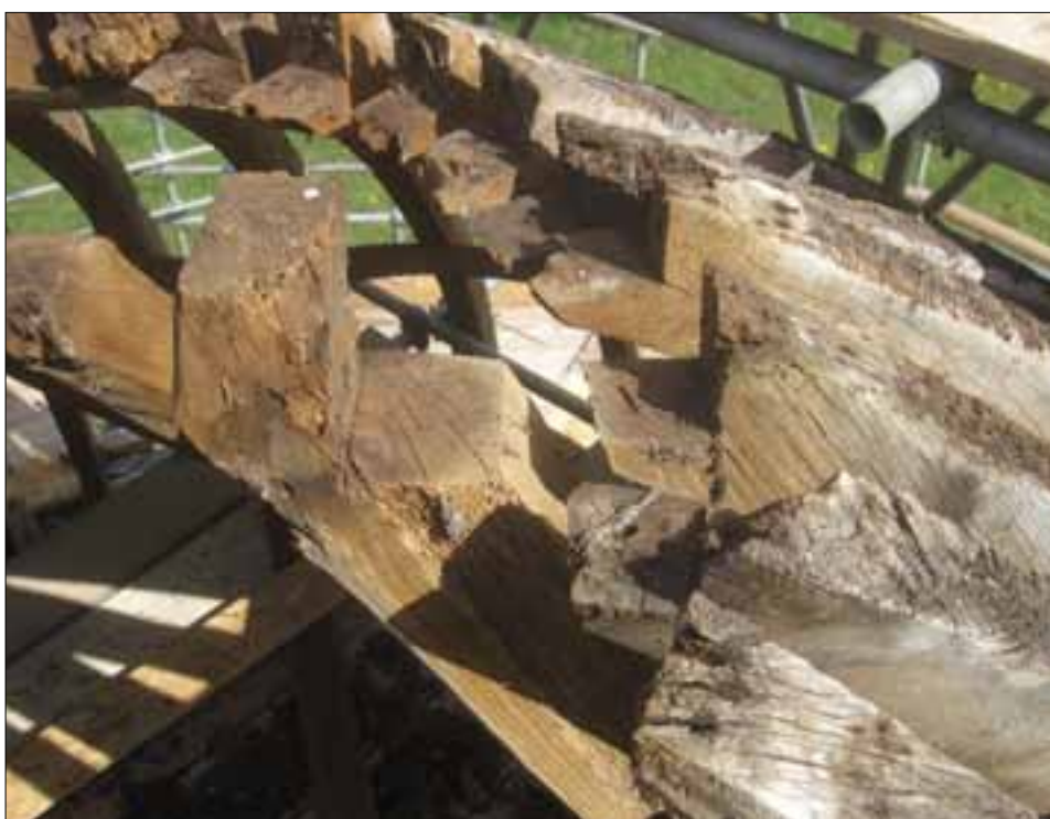
Fig 15 Detail of the birds-mouth joint to the ribs and principal rafters, which fitted against the underside of the lower ring-beam.
