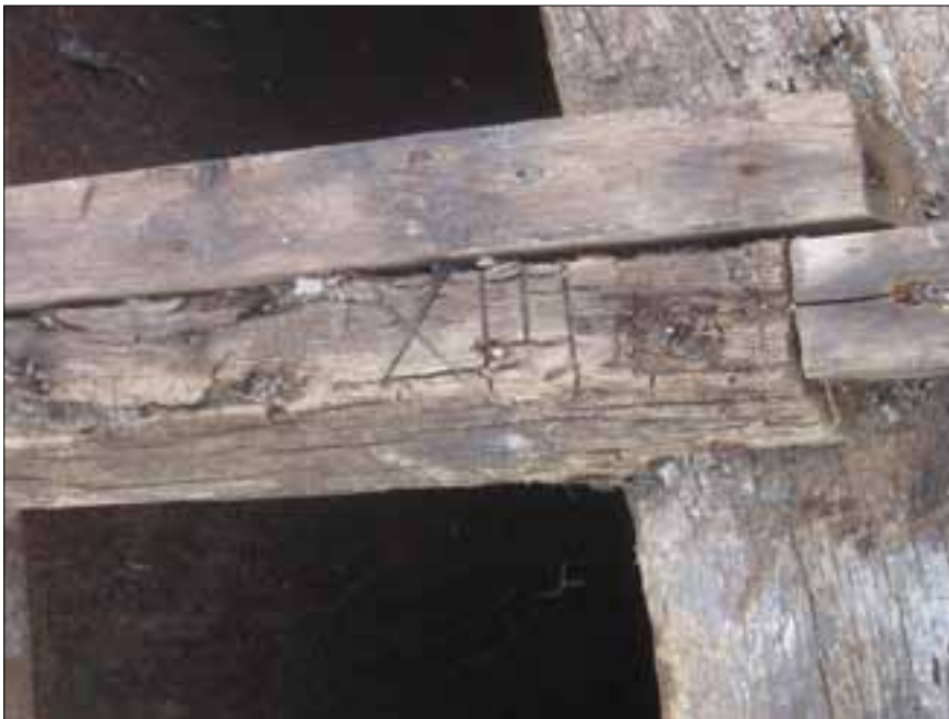
Fig 26 The foot of one of the 'skirt' principal rafters, with carpenter's mark 'XIII'.
