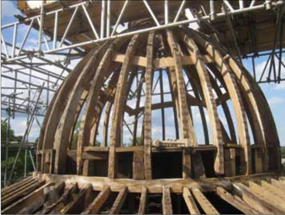
Fig 18 The ribs of the main dome are supported on the dome base plate, which is in turn supported by the lower 'skirt' structure. Some of the straight principal rafters to the dome can also be seen, as well as joist ends of the inserted floor.
