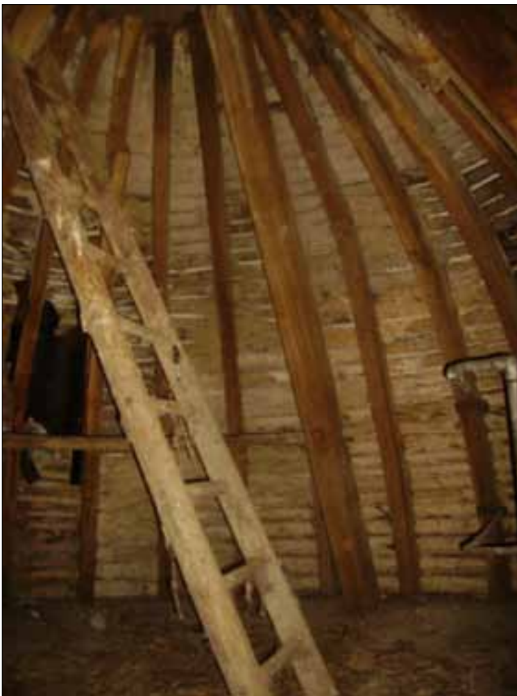
Fig 17 The interior of the main dome before roof stripping. As well as the curved ribs, one of the straight principal rafters is visible.
