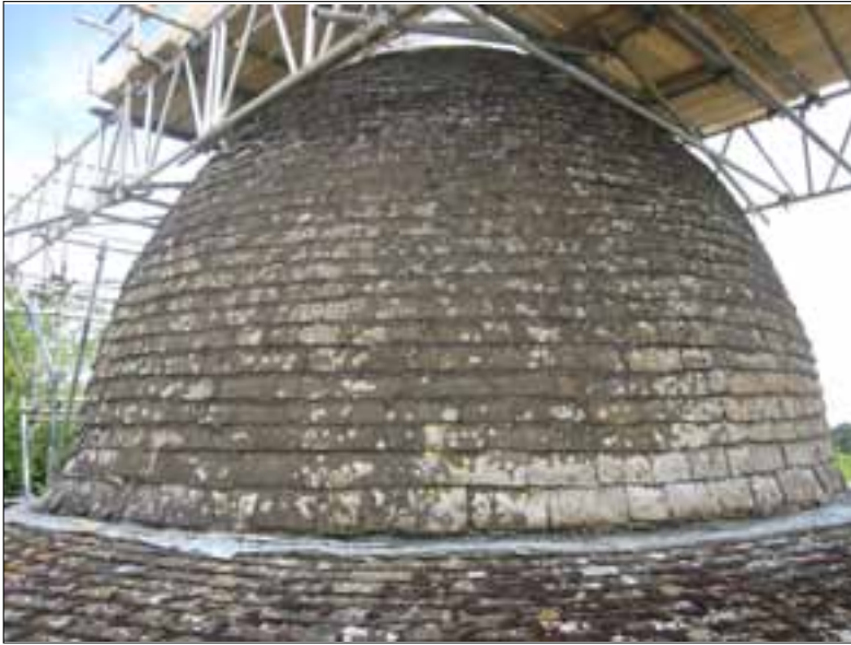
Fig 16 The main dome with Collyweston slate covering.
