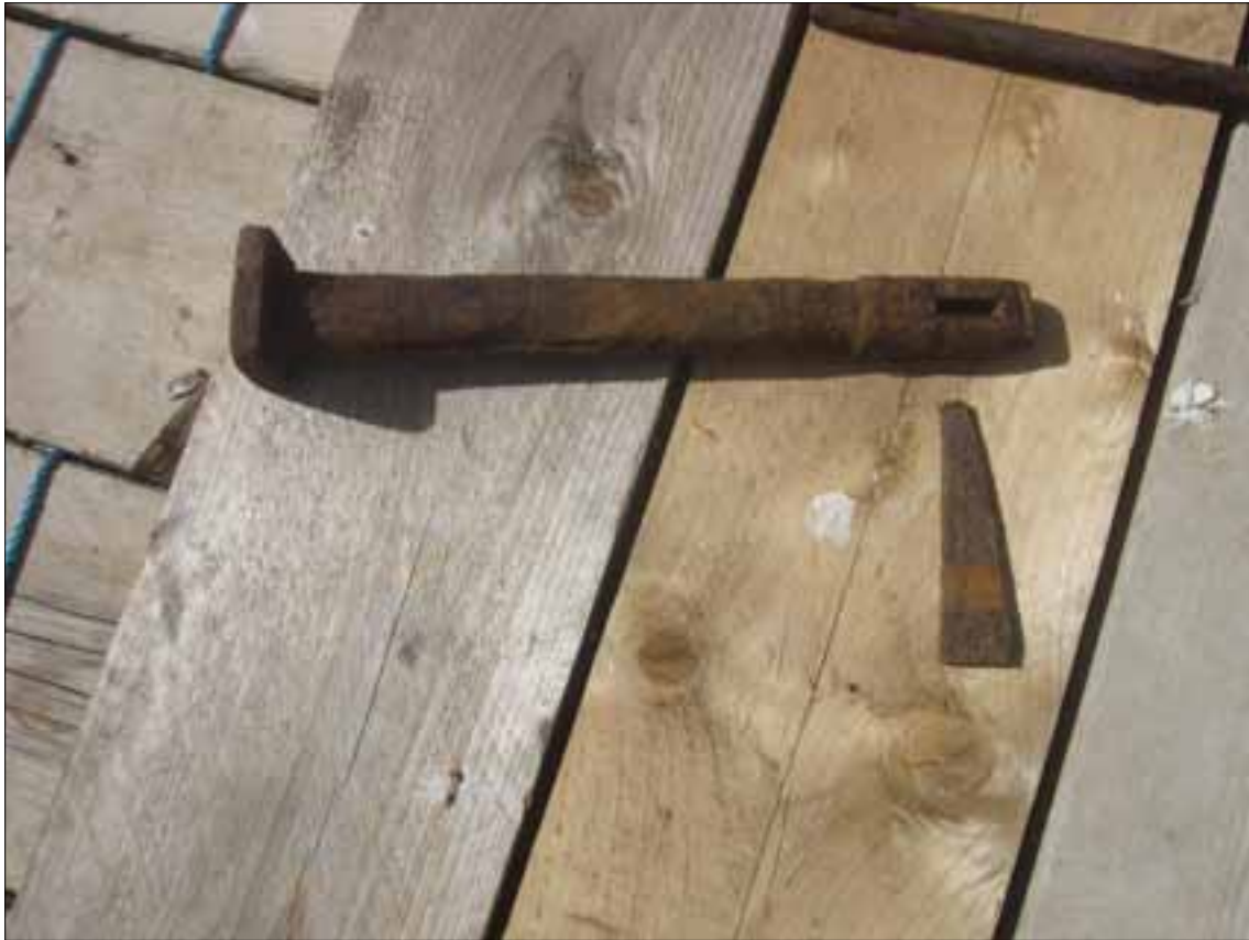
Fig 13 One of the large forelock bolts which were used to fix the upper ring-beam to the lower ring-beam. Driving the thin tapered wedge into the slot tightens up the bolt fixing. The forelock bolts are of various sizes, this being the largest.
