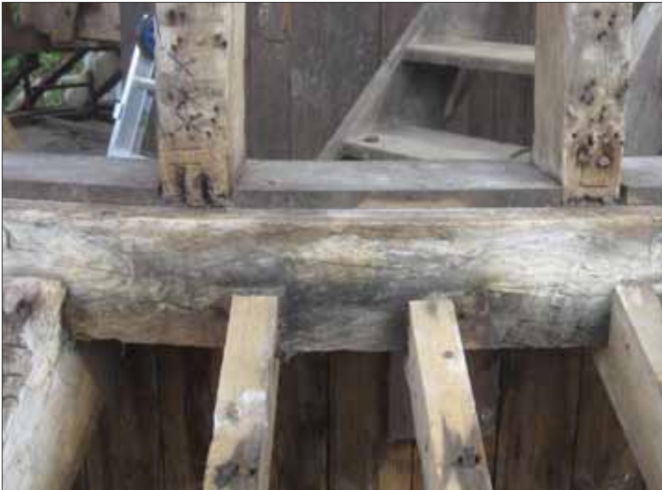
Fig 19 Detail of the dome base plate, with the first and last dome ribs – marked 'I' and 'XXXII'.
