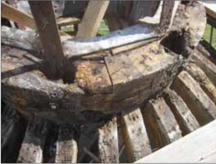
Fig 10 Detail of the upper ring-beam, with pegged, open-tenoned joints and decayed mortices for the original Glover posts.
