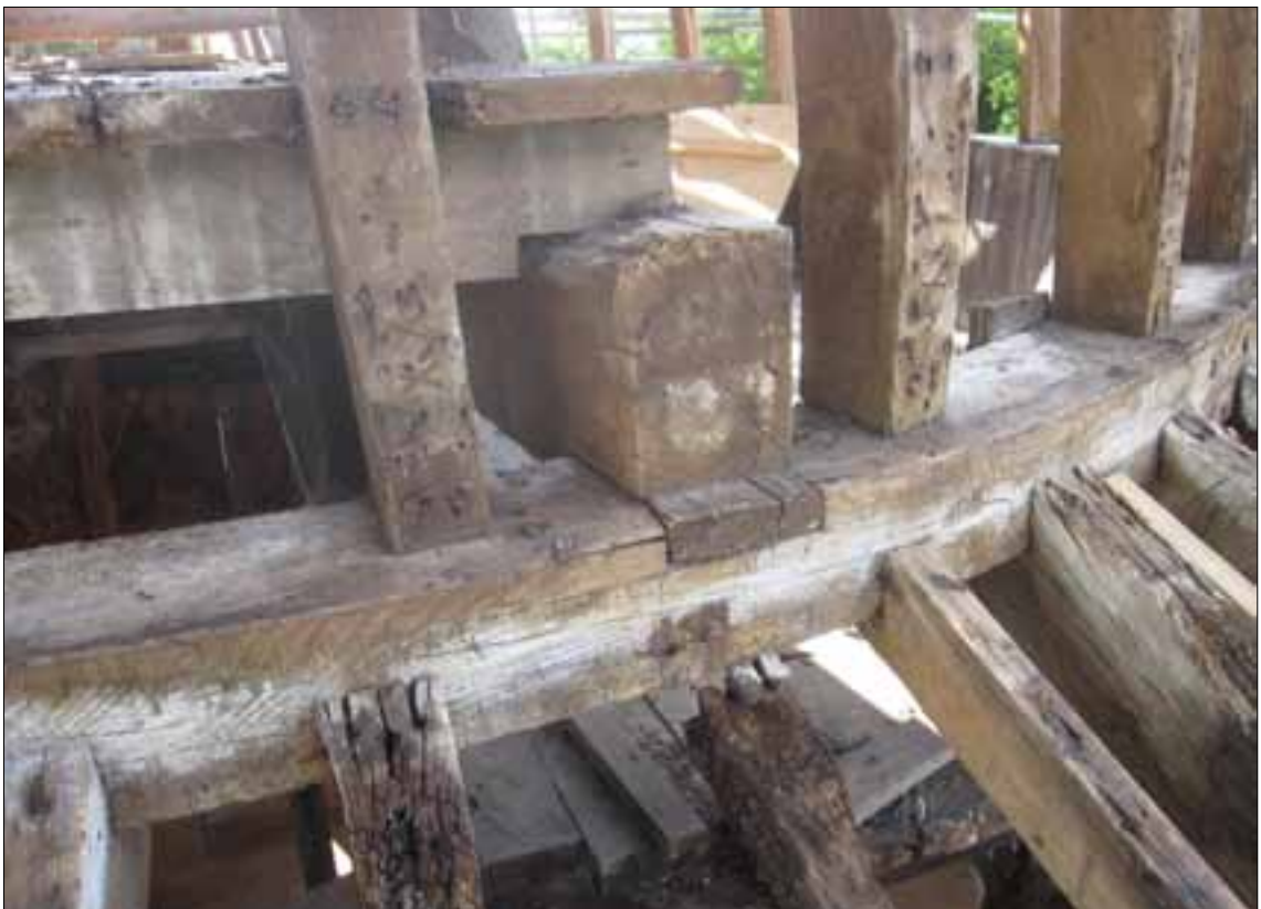
Fig 22 Detail of the dome tie-beam end, with dovetail-lap seating onto the dome base plate.
