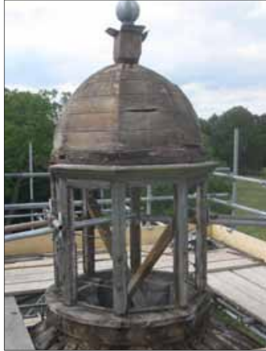
Fig 6 Lantern and cupola after roof stripping. The cupola retains its original boards, but the finial is of 20th-century date.
