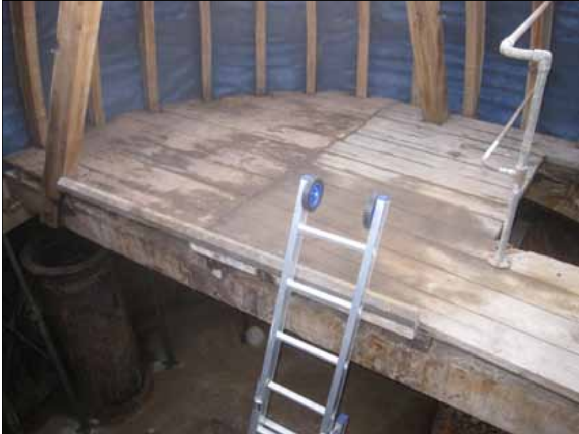
Fig 20 Lower part of a dome principal rafter and the tie-beam – partly covered by the water tank floor.
