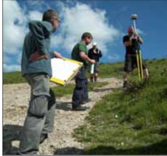
Figure 65: Stage 2 of the marking-out process. Marked nodes were joined by tape measure and line sprayed with bio-degradable, water-based paint. The marking-out team (top to bottom); Jon Horgan (OS – with GPS); John Hayes (Dorset Countryside Ranger Service); Stewart Ainsworth (English Heritage); Roger Lewis (OS); Peter Addison (English Heritage). Photograph courtesy of Chris Bird.
