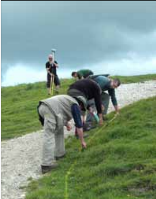
Figure 65: Stage 2 of the marking-out process. Marked nodes were joined by tape measure and line sprayed with bio-degradable, water-based paint. The marking-out team (top to bottom); Jon Horgan (OS – with GPS); John Hayes (Dorset Countryside Ranger Service); Stewart Ainsworth (English Heritage); Roger Lewis (OS); Peter Addison (English Heritage). Photograph courtesy of Chris Bird.
