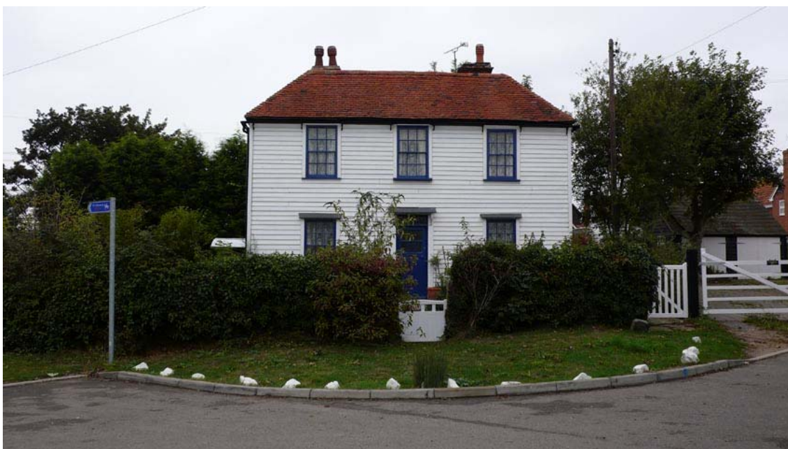
Figure 64 Whitehouse Farm, Chapel Road, Grain; an example of a house with weatherboarding.
