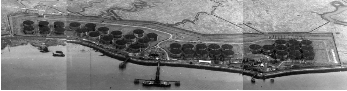
Figure 5 Admiralty fuel oil station on the Isle of Grain in 1950 (composite detail of RAF 540/393 PO20-23 30-Jul-1950 English Heritage RAF Photography).
