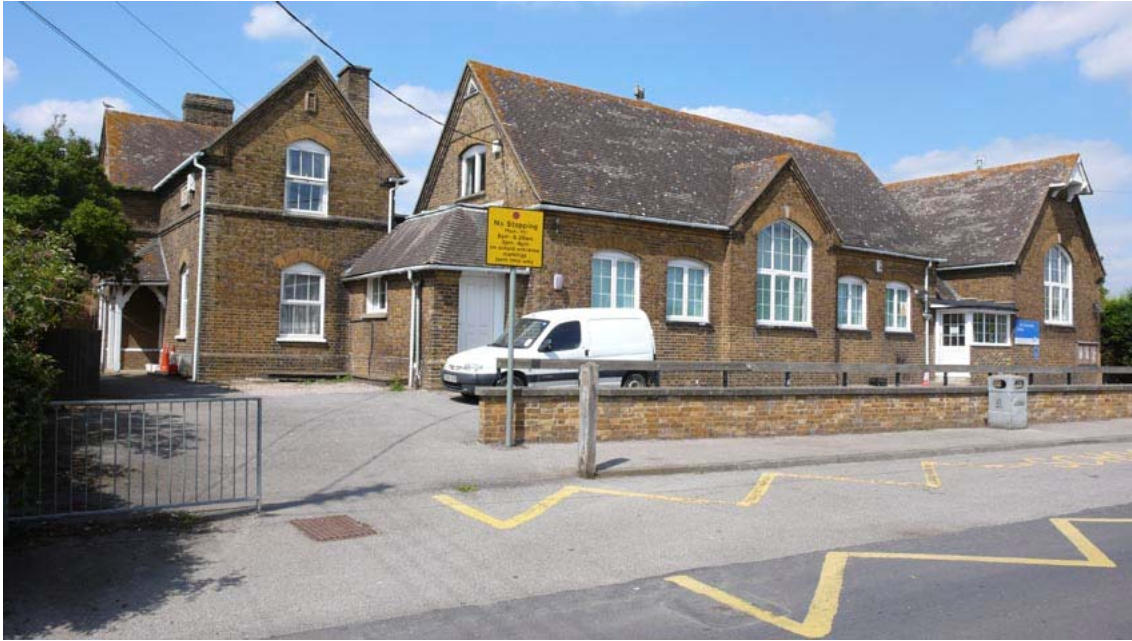
Figure 62 Stoke Community School, Allhallows Road, Lower Stoke. One of the two schools built in the peninsula by the local education board in the wake of the 1870s Education Act. P1090154 © English Heritage.
