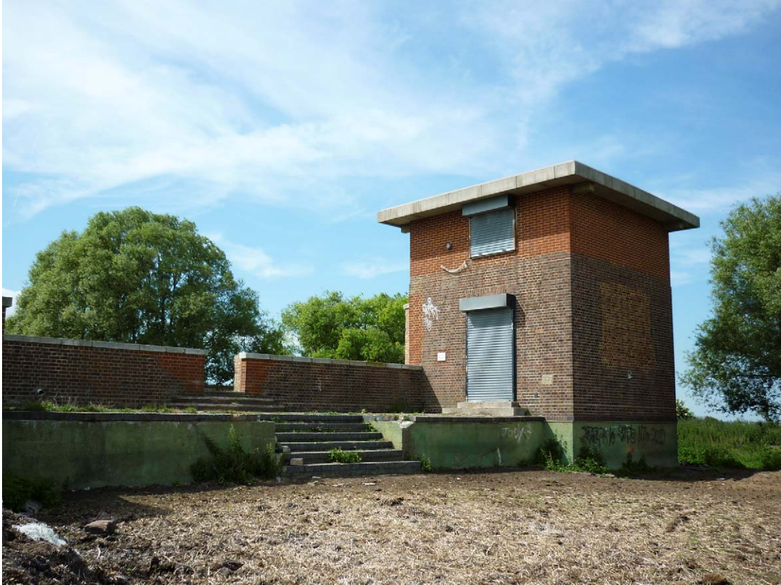
Figure 14 The surviving remains of Cooling Radio Station. The main apparatus building was demolished to basement level but the lower portion of the generator room at the north-eastern corner of the building remains intact. © English Heritage.
