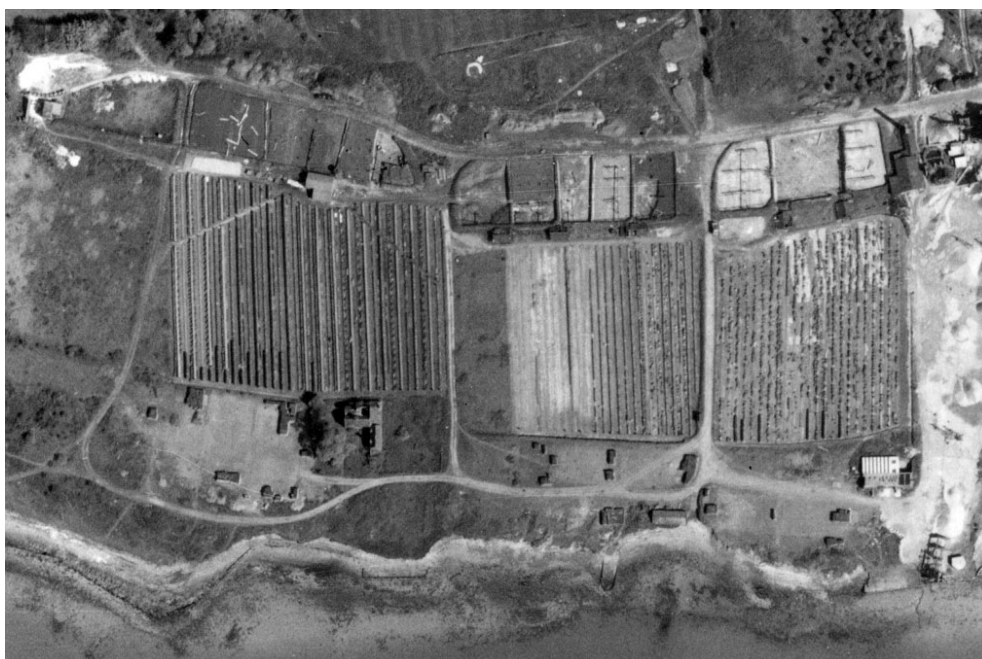
Figure 20 The brickworks at Hoo St. Werburgh. The washbacks where the clay settled are at the top of the photograph; some are partly dug out. The moulding sheds are below the washbacks. The straight and narrow rows across the middle are evidence of drying bricks. RAF 106G/UK/1444 3132 1-May-1946 English Heritage RAF Photography.
