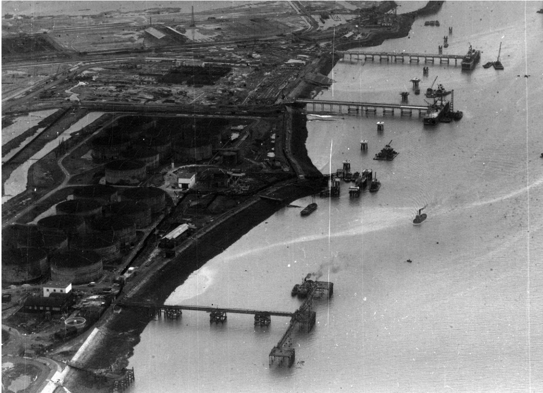
Figure 12 BP refinery jetties on the Isle of Grain in 1953. The tanks on the left were formerly part of the Admiralty fuel oil station. Floodwater can also be seen amongst some of the buildings. RAF 540/1017 I 18 5-Feb-1953 English Heritage RAF Photography.
