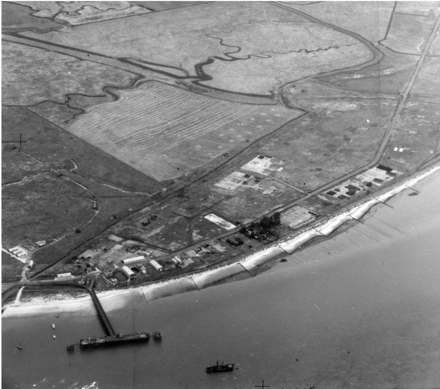
Figure 49 The remains of the site of the RNAS on Grain in 1950. RAF 540/393 PO29 30-JUL-1950 English Heritage RAF Photography.
