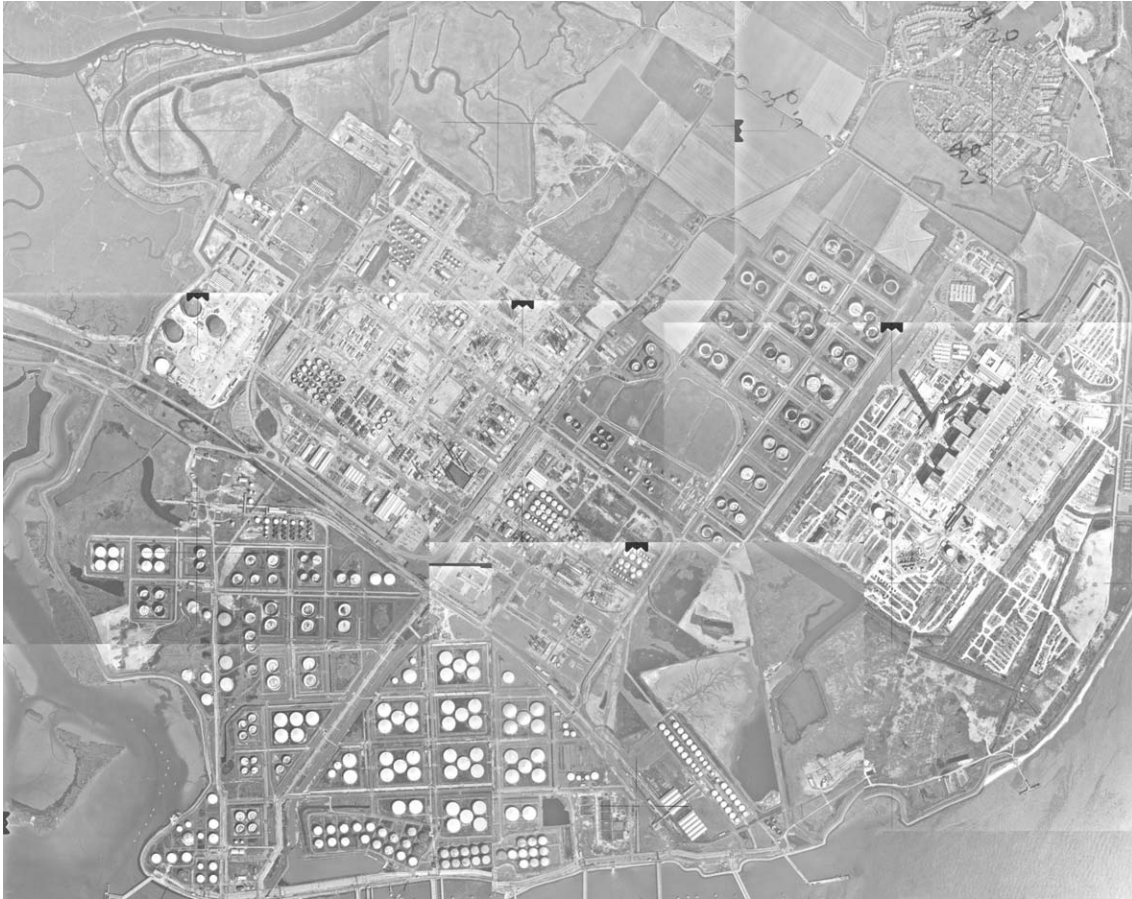
Figure 11 Grain refinery and power station in August 1978. Composite of OS/78123 67, 70, 72; OS/78125 224, 226,260, 262, 264 17/18-Aug-1978 © Crown copyright. Ordnance Survey.
