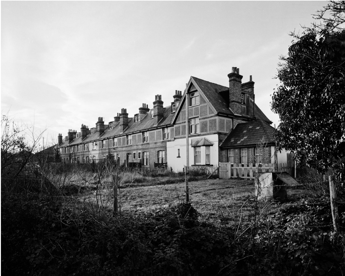
Figure 65 Nos 1-10 Coastguard Cottages, Chapel Road, Grain. AA98/07957 © English Heritage.
