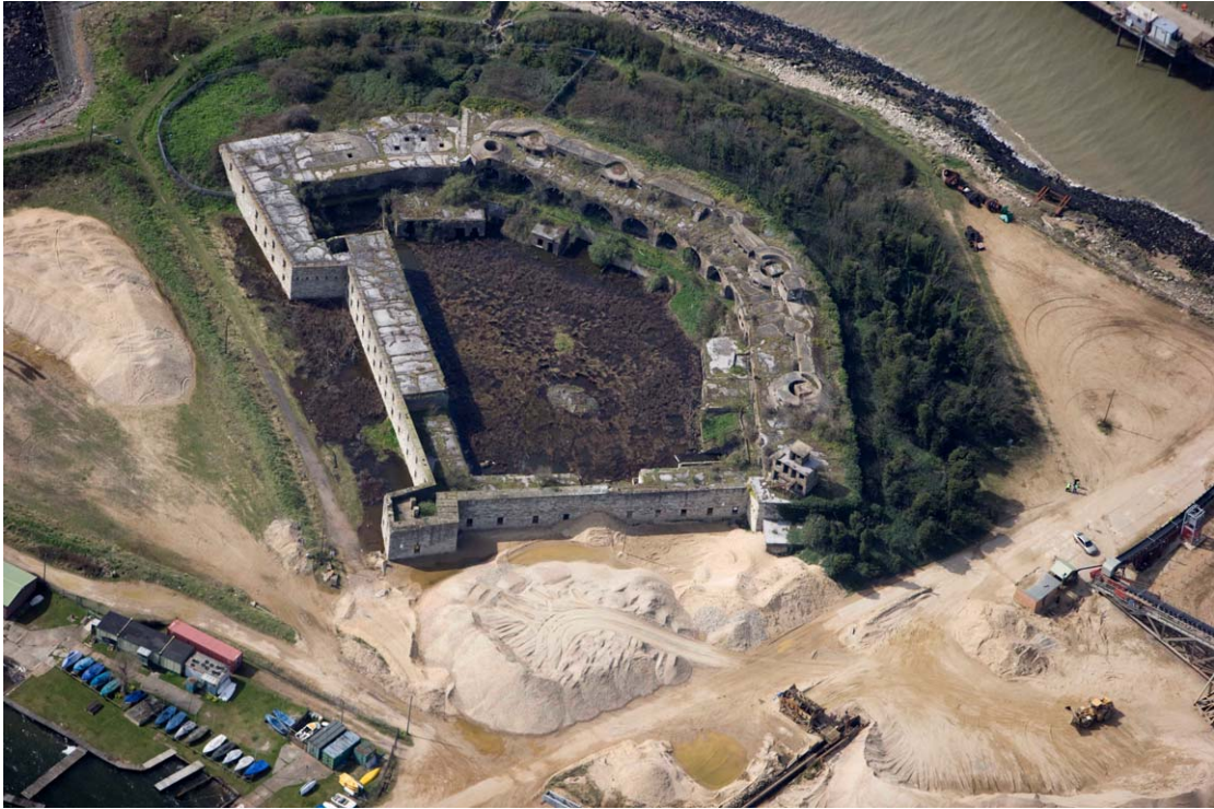
Figure 41 Aerial view of the flooded remains of Cliffe Fort surrounded by heaps of aggregates. 26604/008 6-Apr-2010 © English Heritage.
