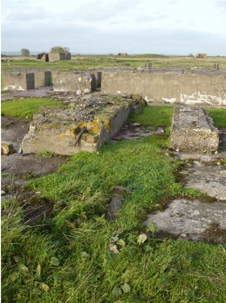
Figure 18 The concrete remains of machine beds at the Cliffe Explosives Works. Despite few buildings surviving beyond floor slabs and machine beds the layout of the factory can still be clearly understood. © English Heritage.
