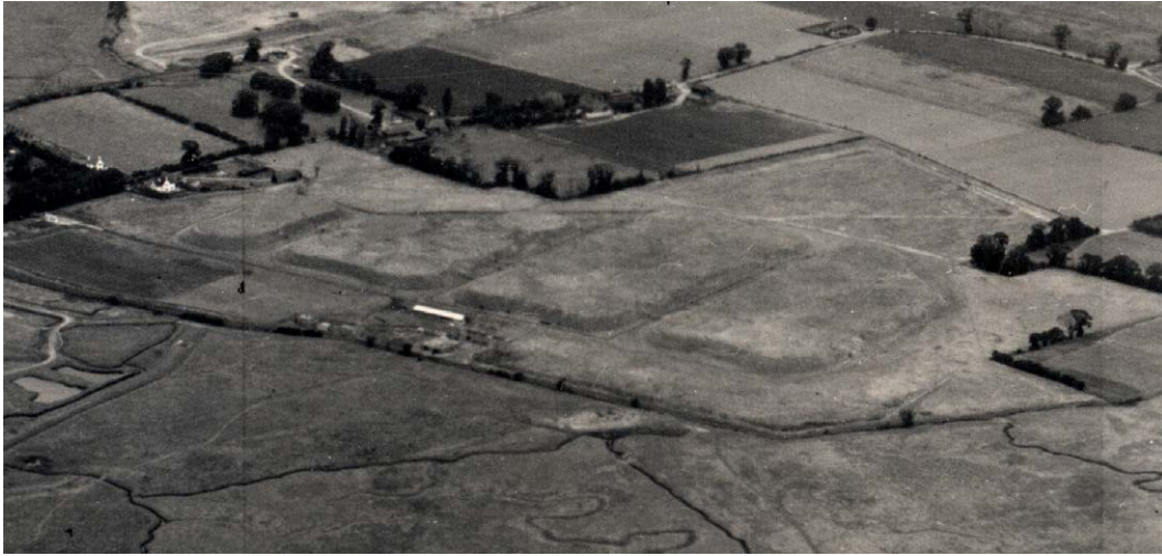
Figure 10 Buried oil tanks on Grain built during the Second World War. They were later incorporated into the BP refinery built there. RAF 540/393 PO-28 30-Jul-1950 English Heritage RAF Photography.
