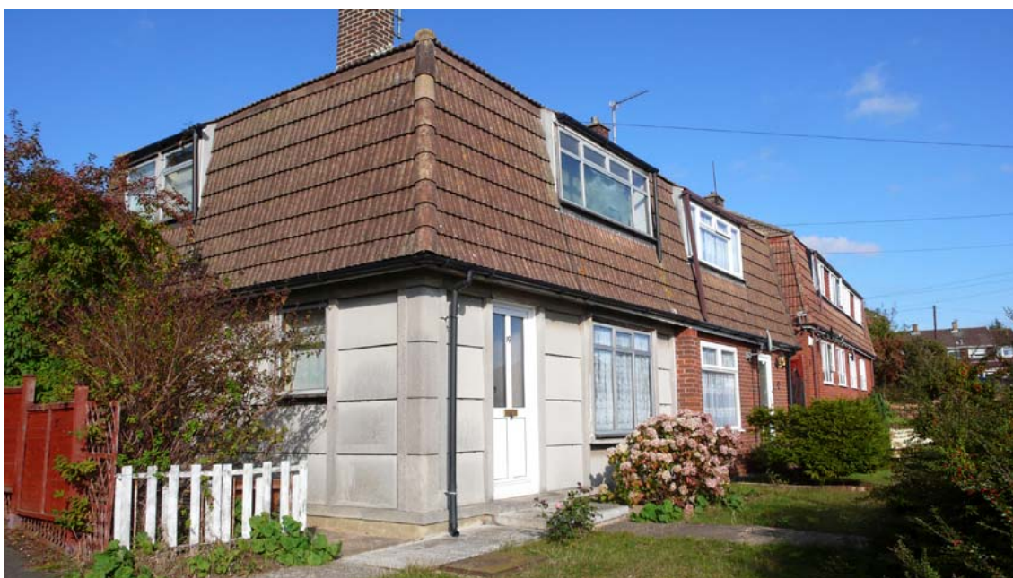
Figure 55 Example of surviving unfaced Cornish Unit Type I pre-cast concrete house in Hoo St. Werburgh. The use of these types of pre-cast building system reflects the need to respond to housing demands quickly and cheaply (P1090914) © English Heritage.
