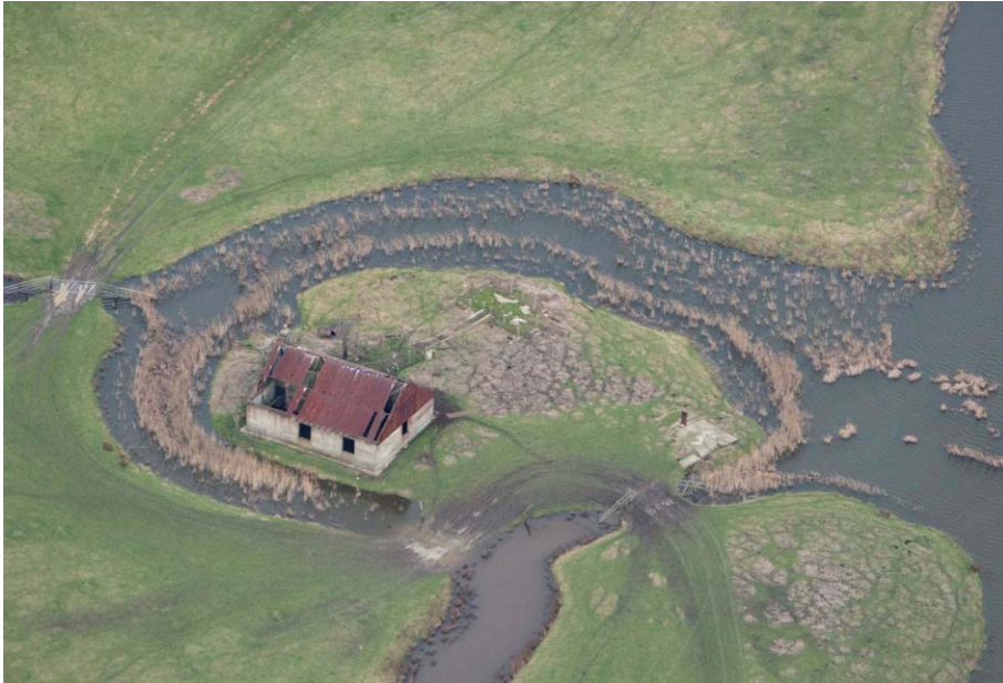
Figure 82 Modern but derelict building next to Cliffe Fleet. This site has had buildings on it since at least the late 17th century and is located top right in the previous figures (Figs 80 and 81). 26866/37 23-Jan-2011 © English Heritage.
