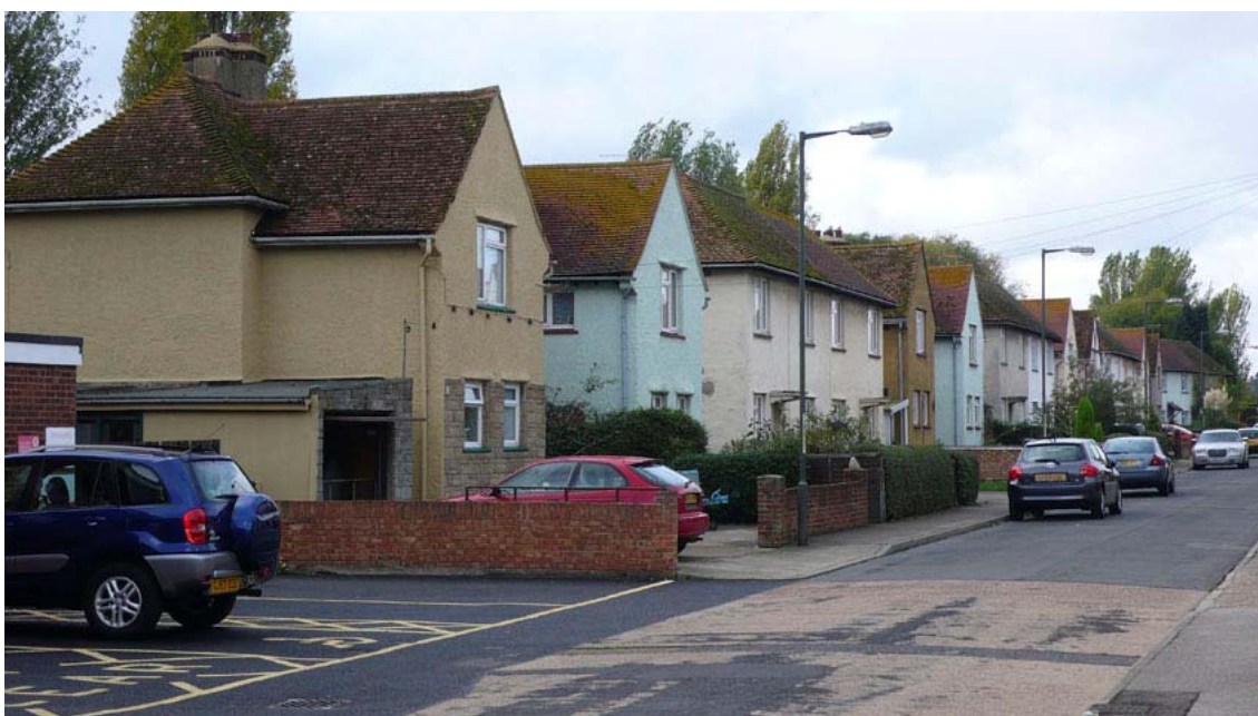
Figure 53 The first generation of local authority housing on Hoo was built in the 1920s and includes these houses in St. Werburgh Crescent, Hoo St. Werburgh (P1090842) © English Heritage.
