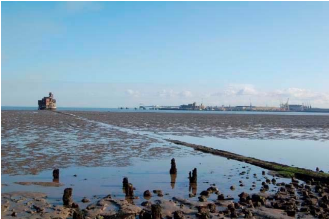
Figure 29 Grain Tower at low tide with Sheerness in the background. Note the line of the hard to the fort exposed in the mud and the stumps of piles from a late 19th century jetty. © English Heritage 2009.
