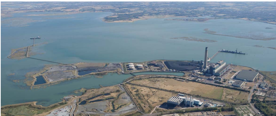
Figure 3 Kingsnorth power station. Detail of 26477/01 | 8-Sep-2009 © English Heritage.
