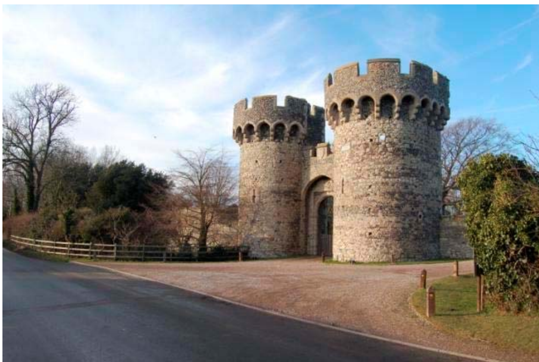
Figure 27 Cooling Castle gatehouse from the road. © English Heritage 2009.
