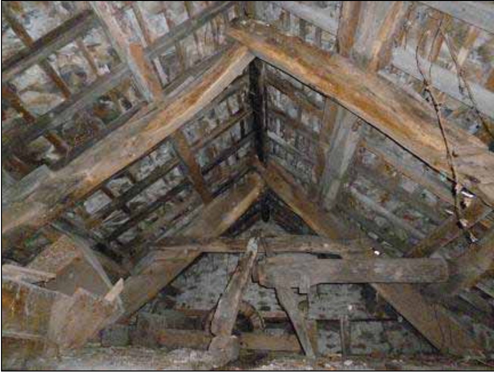
Figure 5: Linnels Mill; roof of the main building (photograph Alison Arnold)
