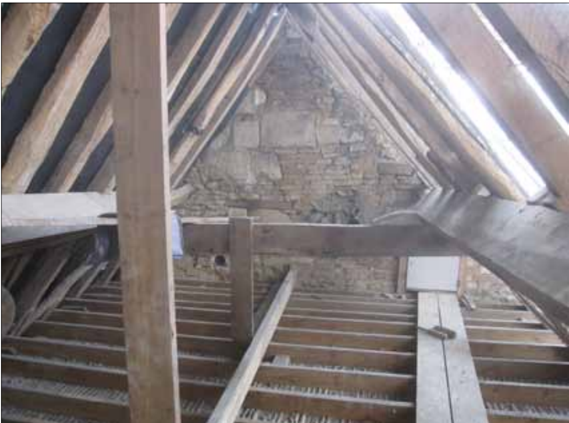
Fig 5.19 West section of roof, looking towards west gable (Nick Hill).
