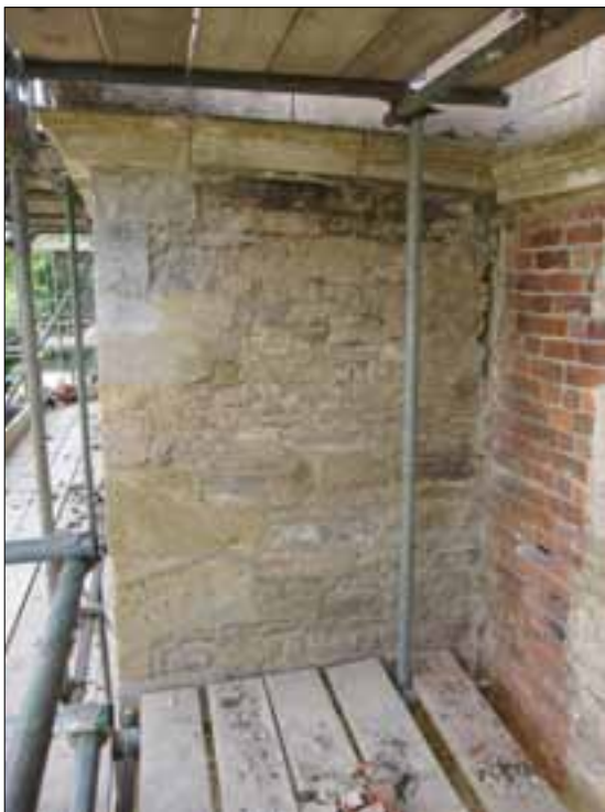
Fig 2.2 Junction of garderobe block (left) and north wall of the north range (right) (Nick Hill).
