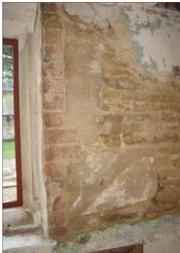
Fig 4.10 West jamb of west window to the former eastern opening, with 18th or 19th-century brickwork cut into the original jamb (Nick Hill).
