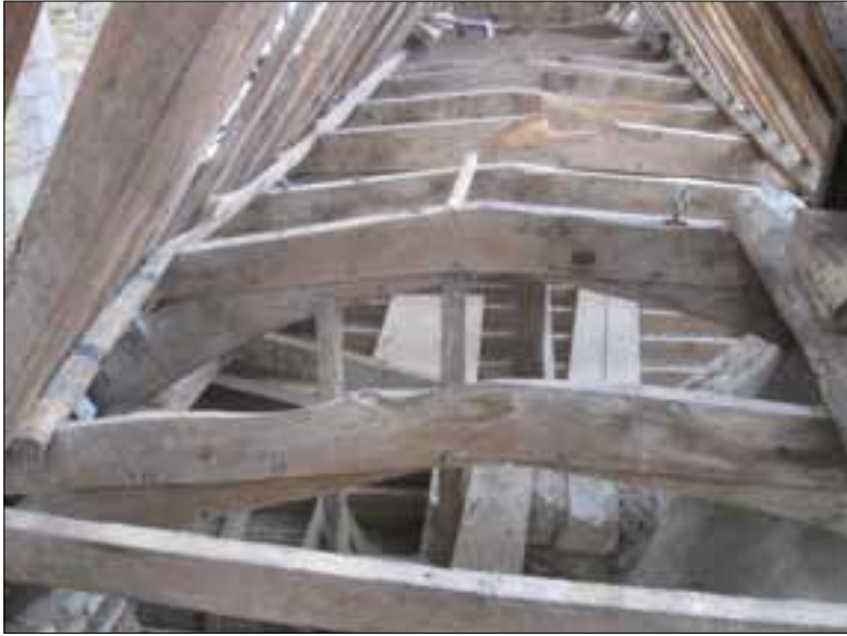
Fig 5.4 East section of roof H2.11, looking west (Nick Hill).
