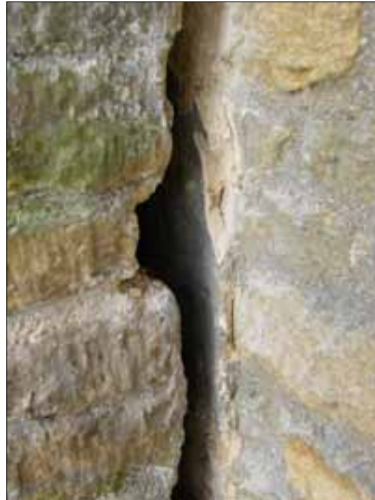
Fig 1.2 Plaster finish to rubble masonry of gatehouse, trapped by addition of Library block. An ashlar joint pressed into the plaster face is visible (Nick Hill).
