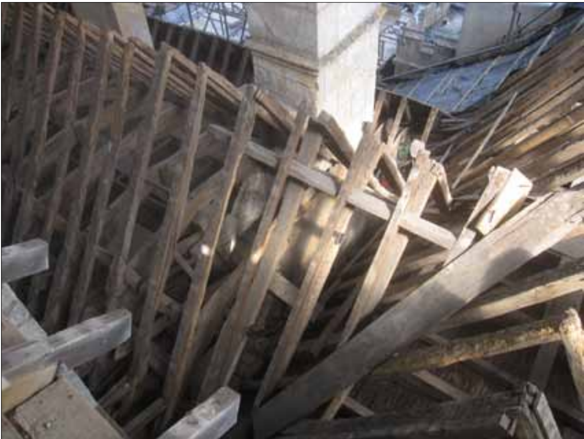
Fig 5.3 East end of roof H2.11, abutting parlour block (Nick Hill).
