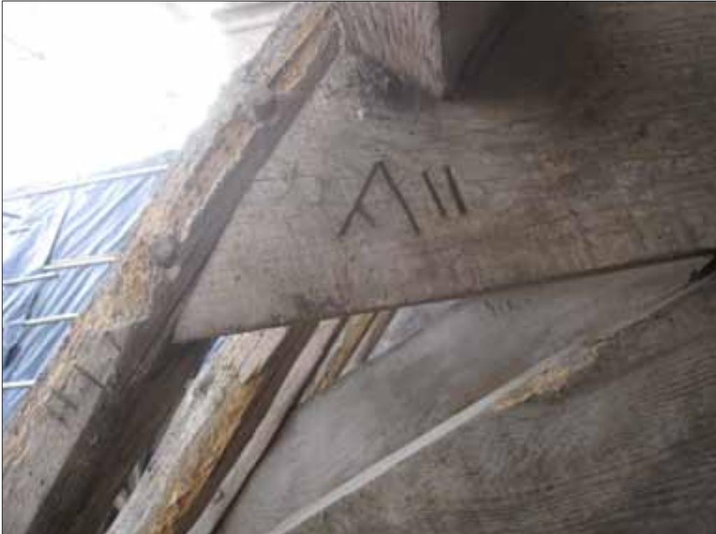
Fig 5.11 Carpenter's mark to truss T6: VII with a tag (Nick Hill).
