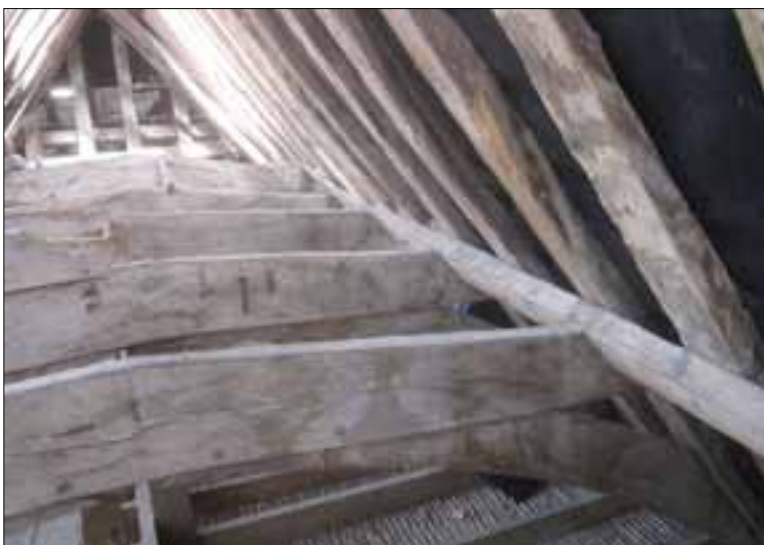
Fig 5.6 East section of roof H2.11, looking east (Nick Hill).
