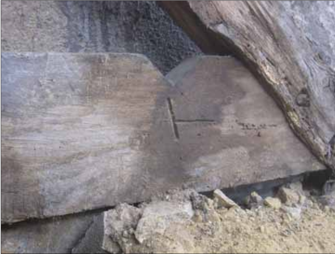
Fig 5.13 Carpenter's mark to truss T2, north end (Nick Hill).
