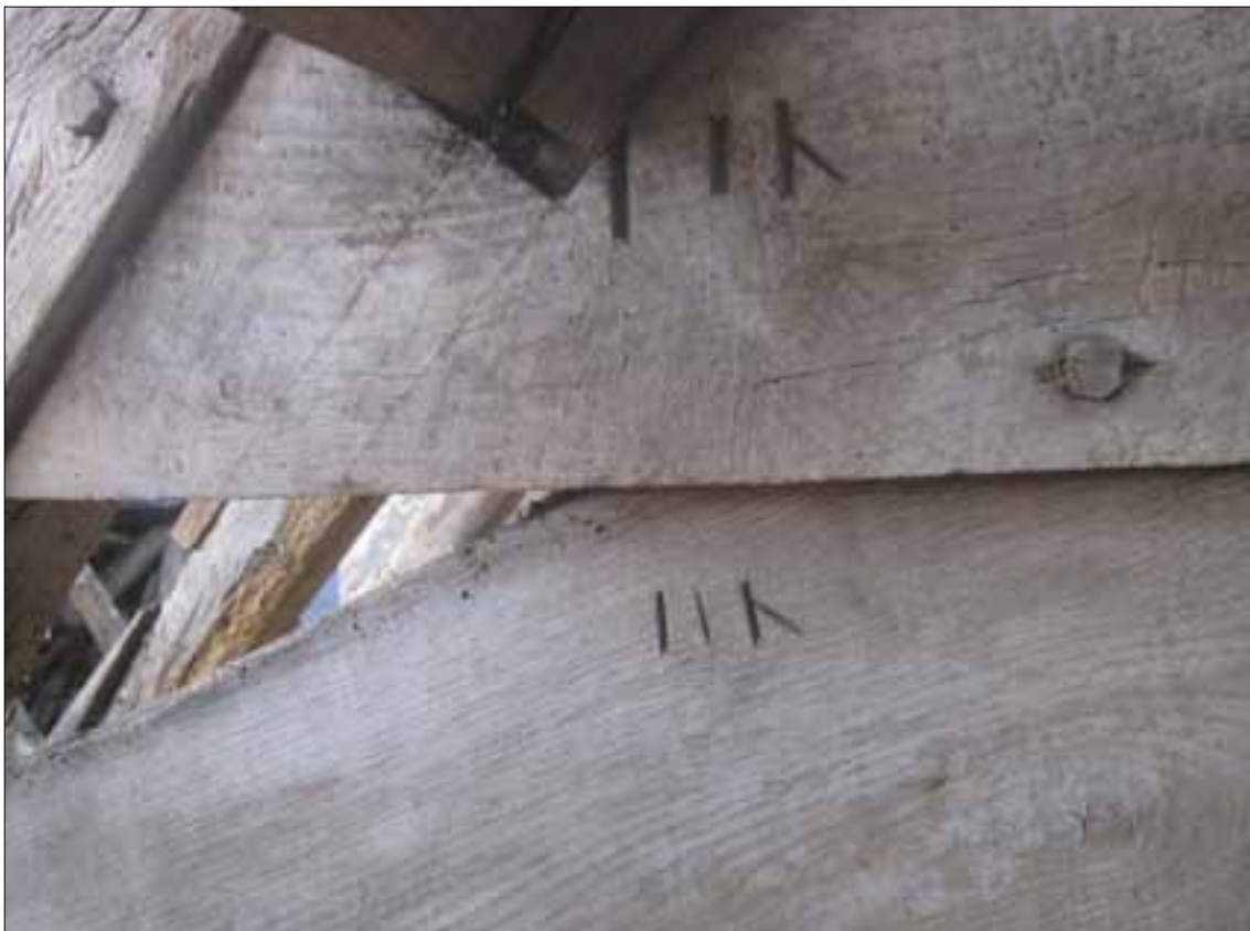
Fig 5.10 Carpenter's mark to truss T5: III with a tag (Nick Hill).
