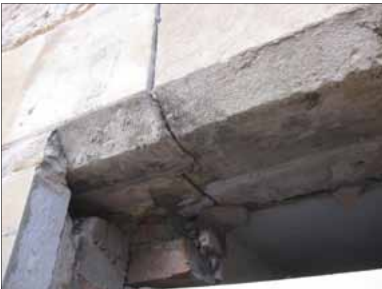
Fig 4.5 Joggled joint to lintel blocks, visible on soffit (Nick Hill).
