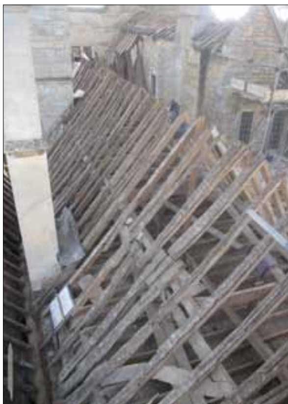
Fig 5.1 View over roof of H2.11 from the west (Nick Hill).
