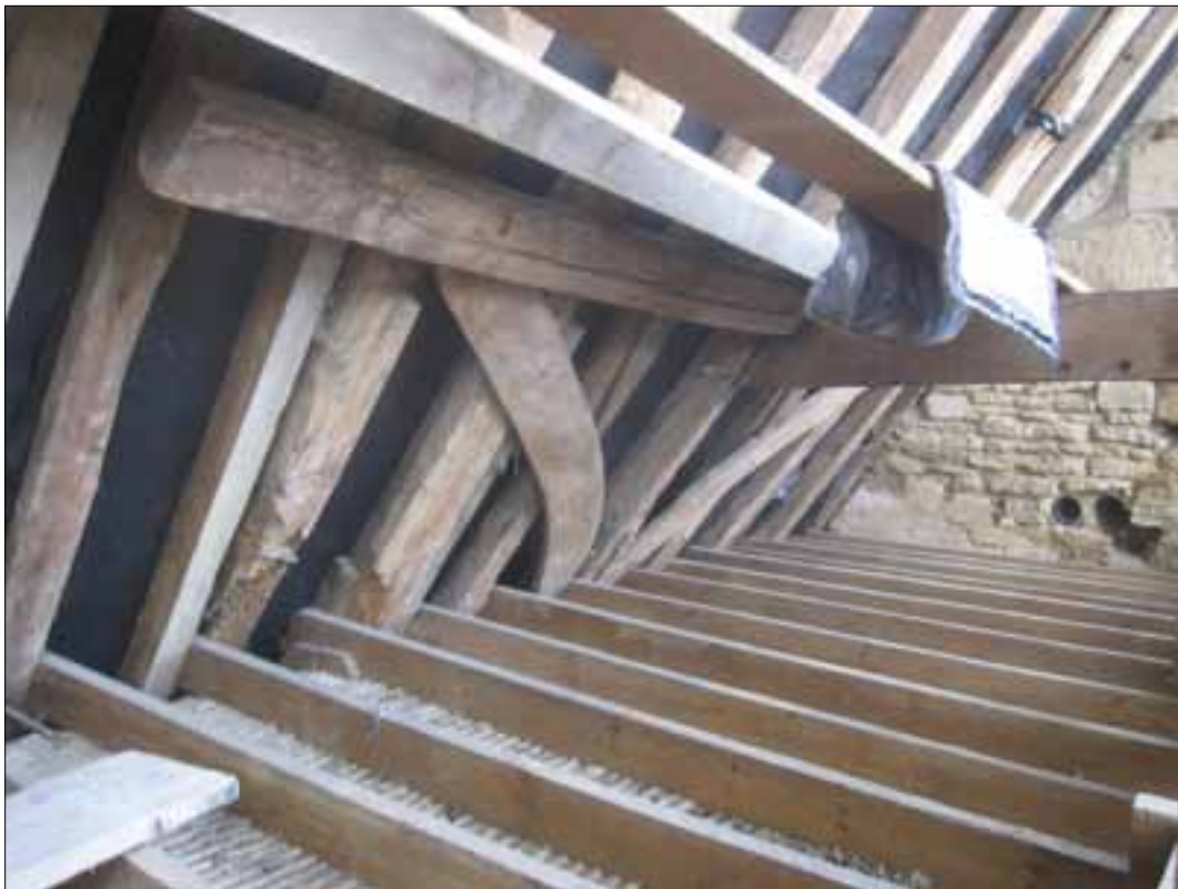
Fig 5.17 West section of roof H2.11, looking west (Nick Hill).
