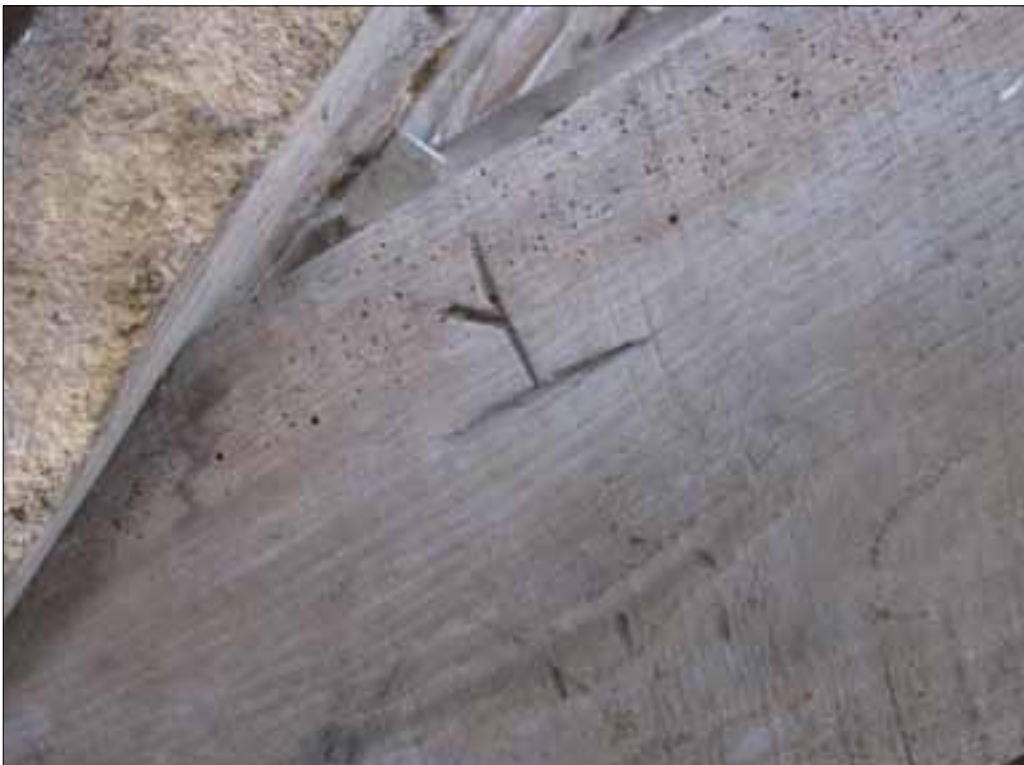
Fig 5.12 Carpenter's mark to truss T2, south end (Nick Hill).
