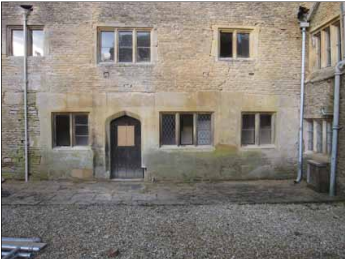
Fig 4.8 Row of seven ashlar blocks to east, with later infill of doorway and three windows (Nick Hill)..
