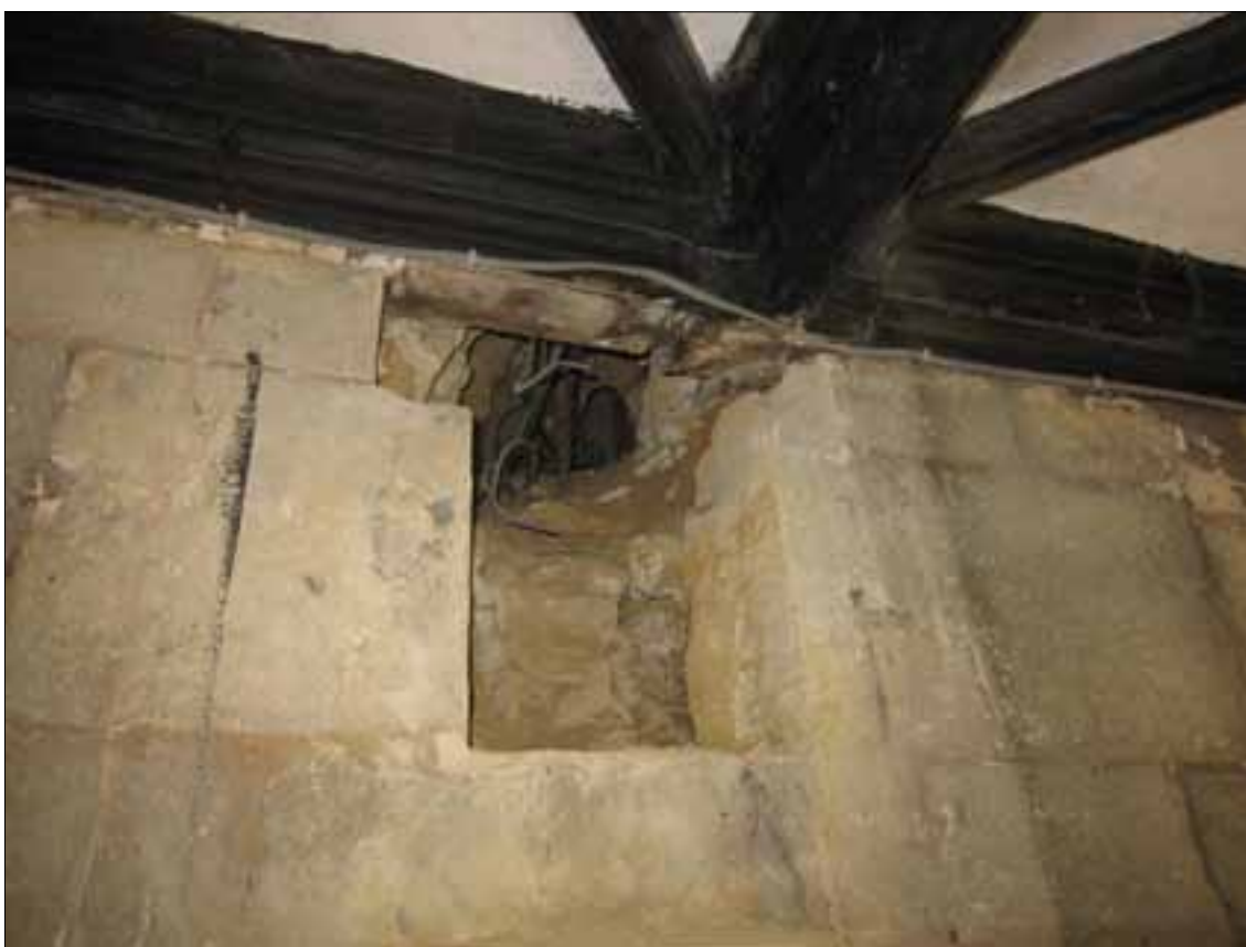
Fig 3.1 East face of Gatehouse entry, with stone ashlar lining (Nick Hill).
