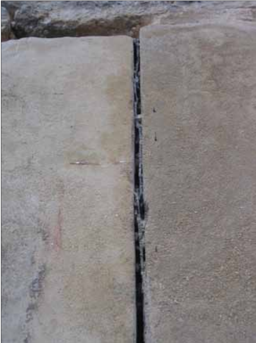
Fig 4.6 Ashlar joint filled with lead, poured in when molten (Nick Hill).
