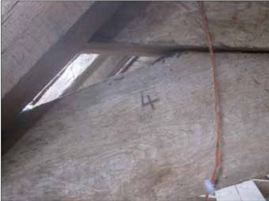
Fig 5.15 Carpenter's mark to truss T8, north end (Nick Hill).
