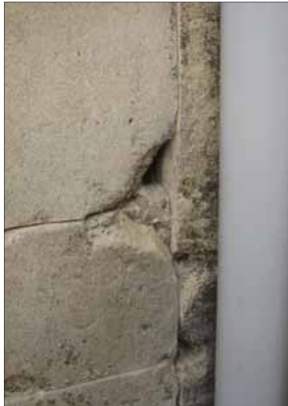
Fig 4.9 East jamb of former eastern opening, with square reveal (Nick Hill).
