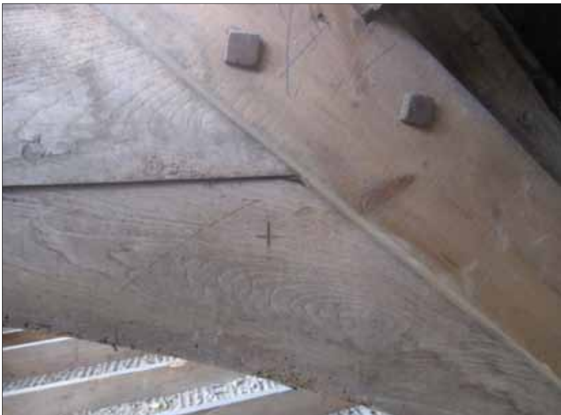
Fig 5.14 Carpenter's mark to truss T8, south end (Nick Hill).
