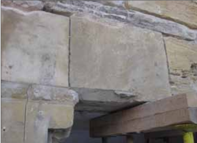
Fig 4.3 Lintel block with chamfer (Nick Hill).
