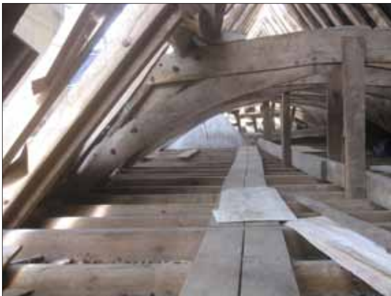
Fig 5.5 East section of roof H2.11, looking east (Nick Hill).
