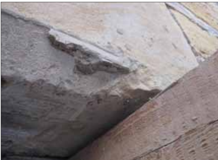
Fig 4.4 Detail of chamfer, with remains of mitred return to jamb (Nick Hill).
