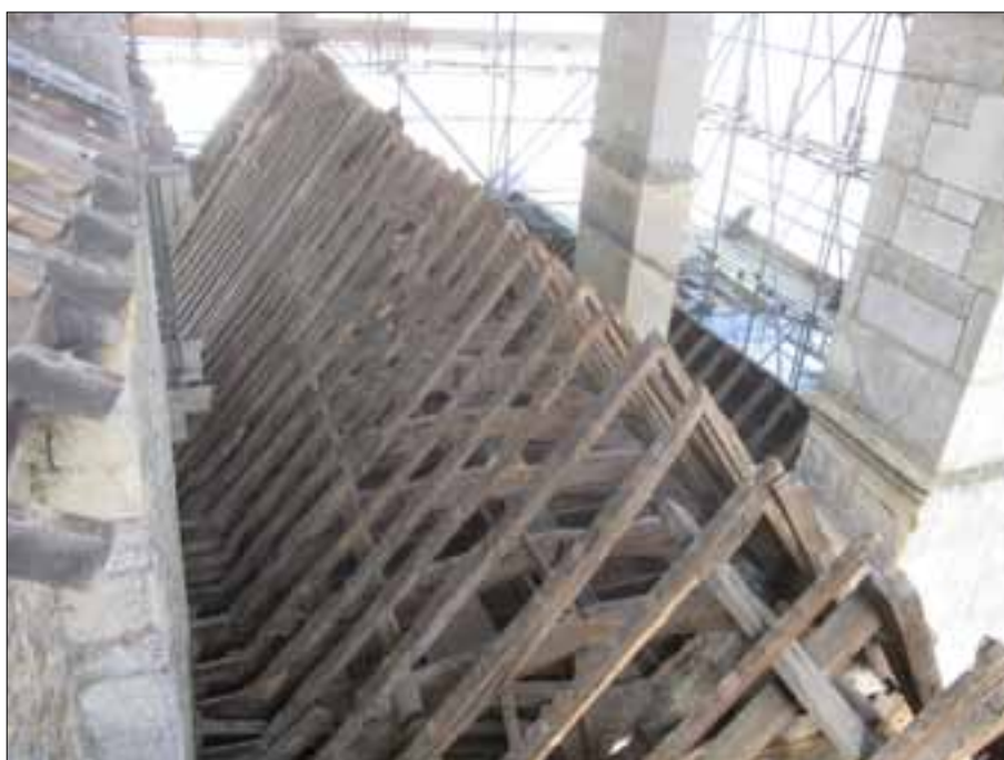
Fig 5.2 View over roof of H2.11 from the east (Nick Hill).
