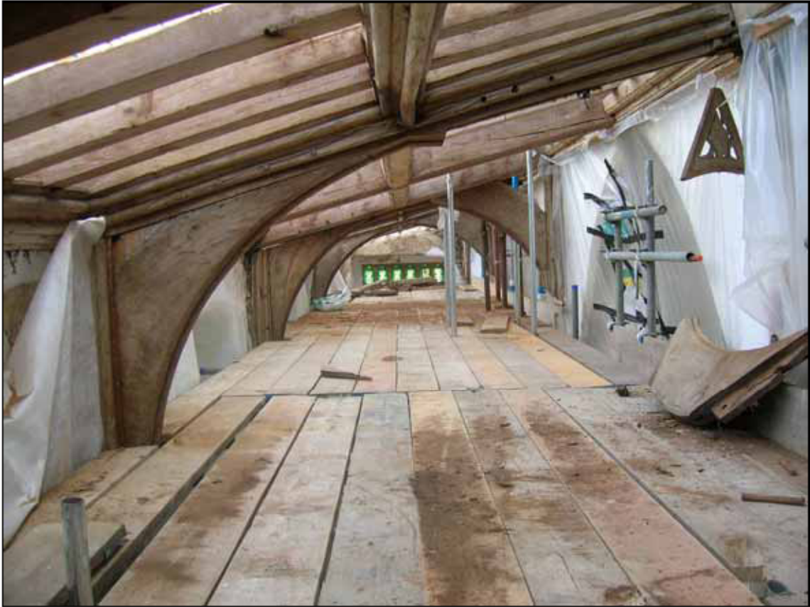
Figure 4: North aisle roof, photograph taken looking east (Robert Howard)
