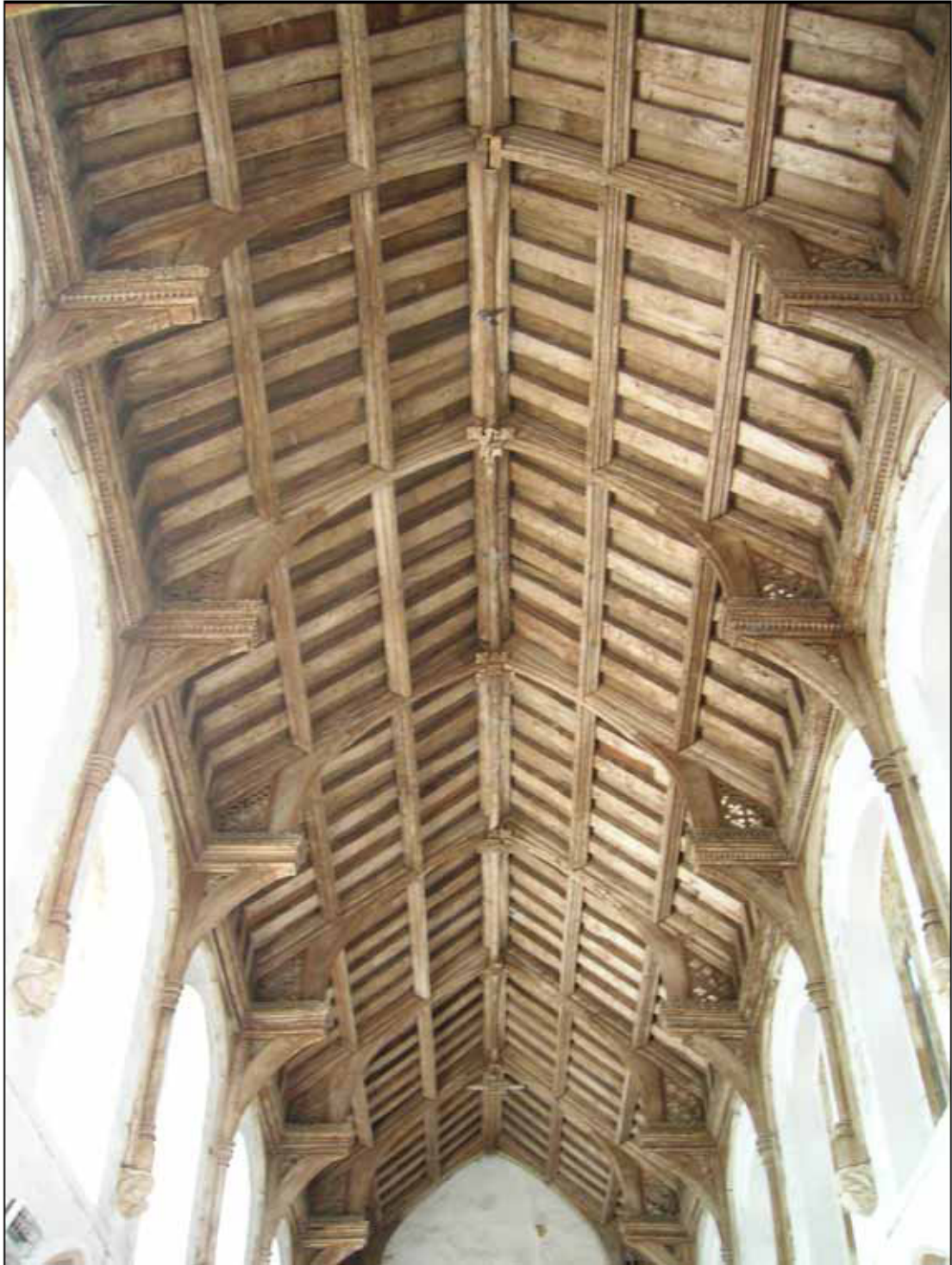
Figure 5: Nave roof, photograph taken looking west (Robert Howard)
