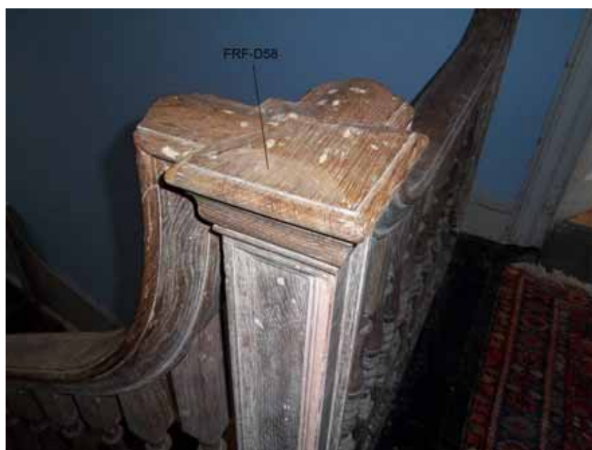
Figure 28: Photograph of first-floor newel post cap, showing the location of sample FRF-D58 in the Connecting range (RobertHoward)
