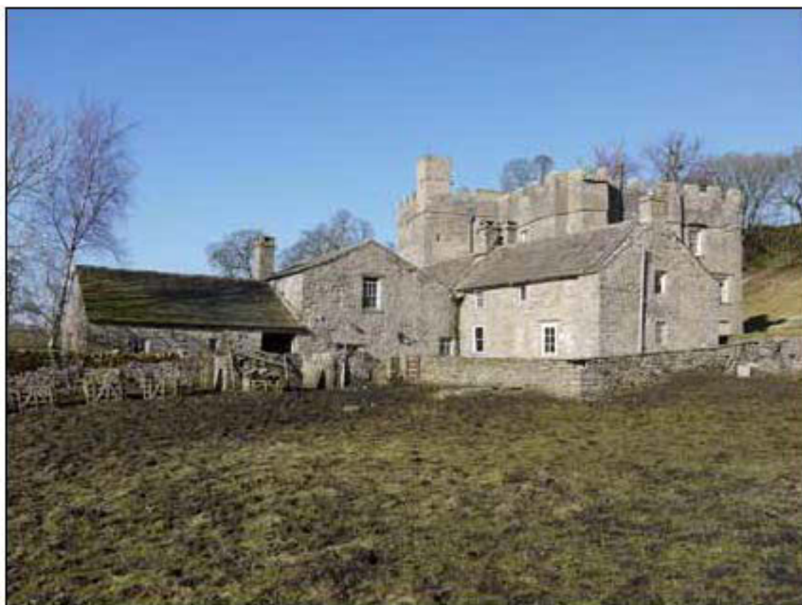
Figure B. The service range viewed from the east (photograph: Lucy Jessop, English Heritage).
