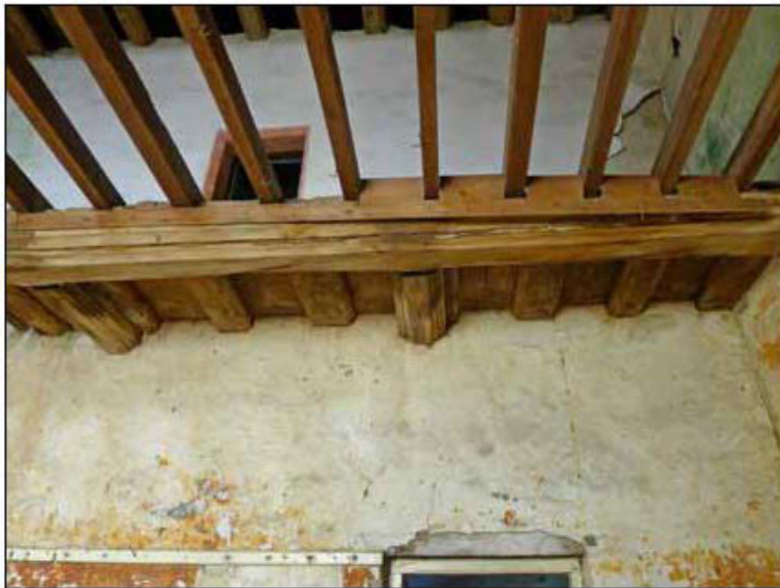
Figure 6. The medieval flooring technique employed in the high-end tower: boards resting in rebates along the joist and beams (photograph: Lucy Jessop, English Heritage).
