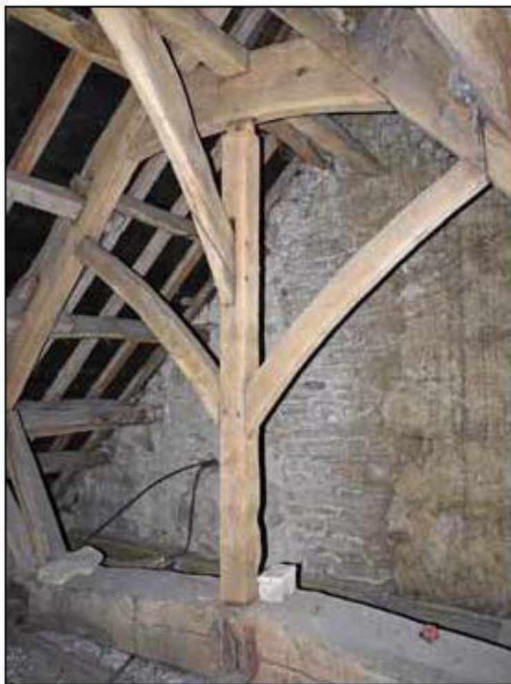
Figure 5. The hall's roof structure with inserted flue behind. (photograph: Adam Menuge, English Heritage).
