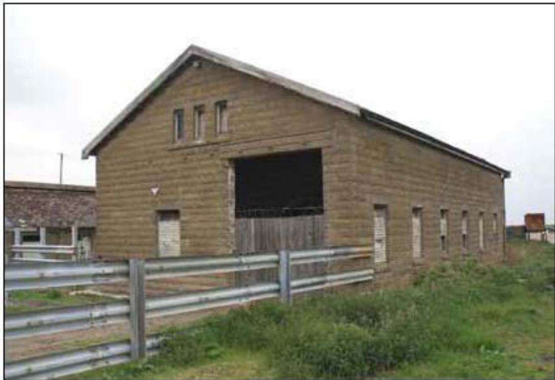
Figure 35. Main workshop building from the east.
