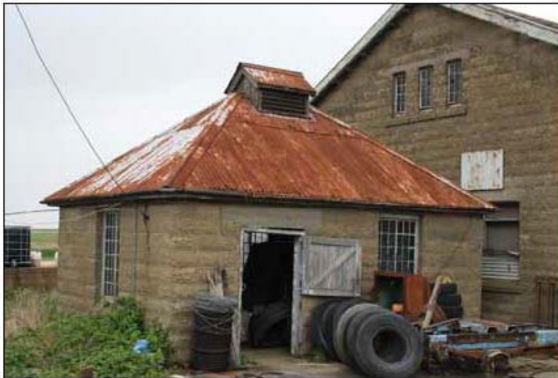
Figure 37. Forge, next to main workshop, from the west.
