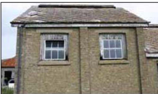
Figure 40. Detail of the taller part of later building, from the south-west or road side. The door is on the other side, facing the main workshop building.
