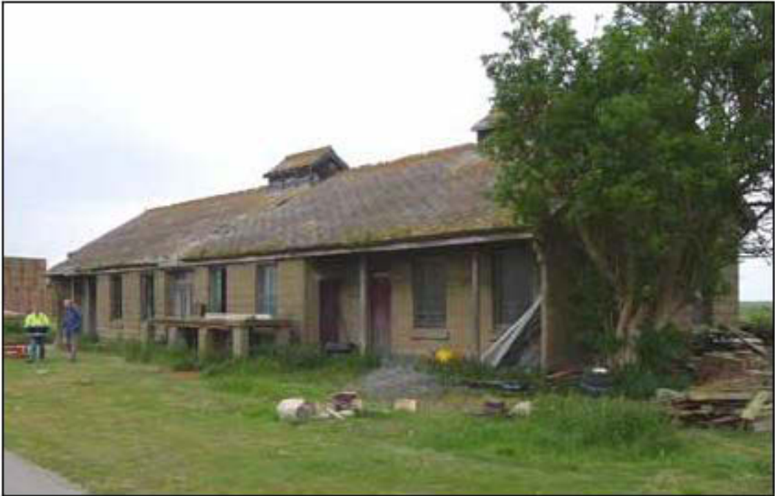
Figure 29. Powerhouse from the south.
