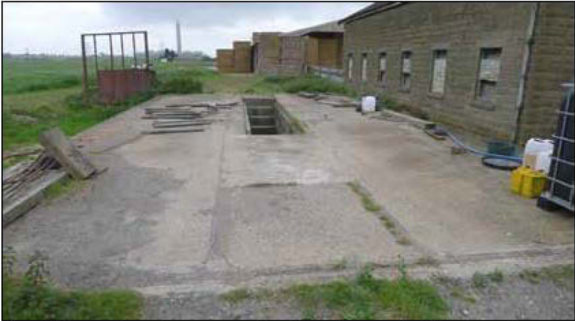
Figure 38. Concrete base with inspection pit, formerly a railway engine shed, from the north-west.
