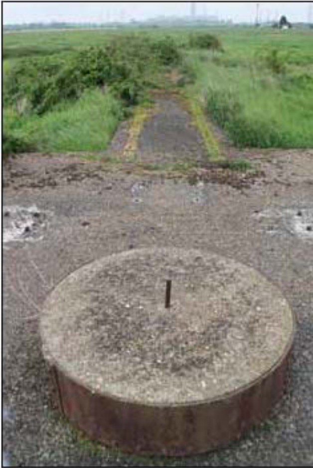
Figure 47. Looking southeast along arm of inner and shorter velocity screen mast base.
