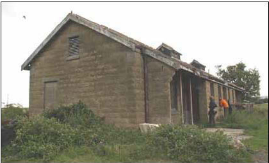
Figure 30. Powerhouse from the north-west.
