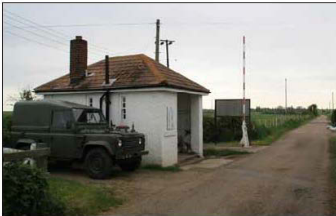
Figure 26. Guardhouse and barrier from the west.
