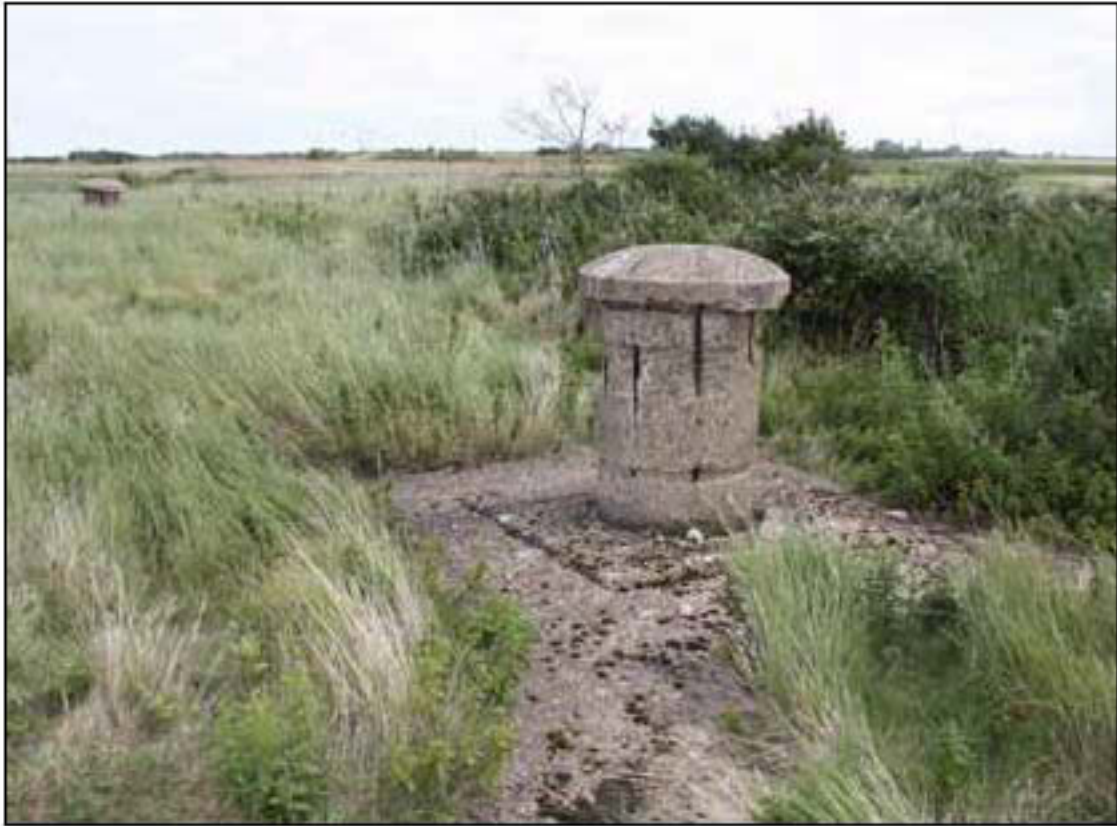
Figure S6. Ballards for tethering, looking east.
