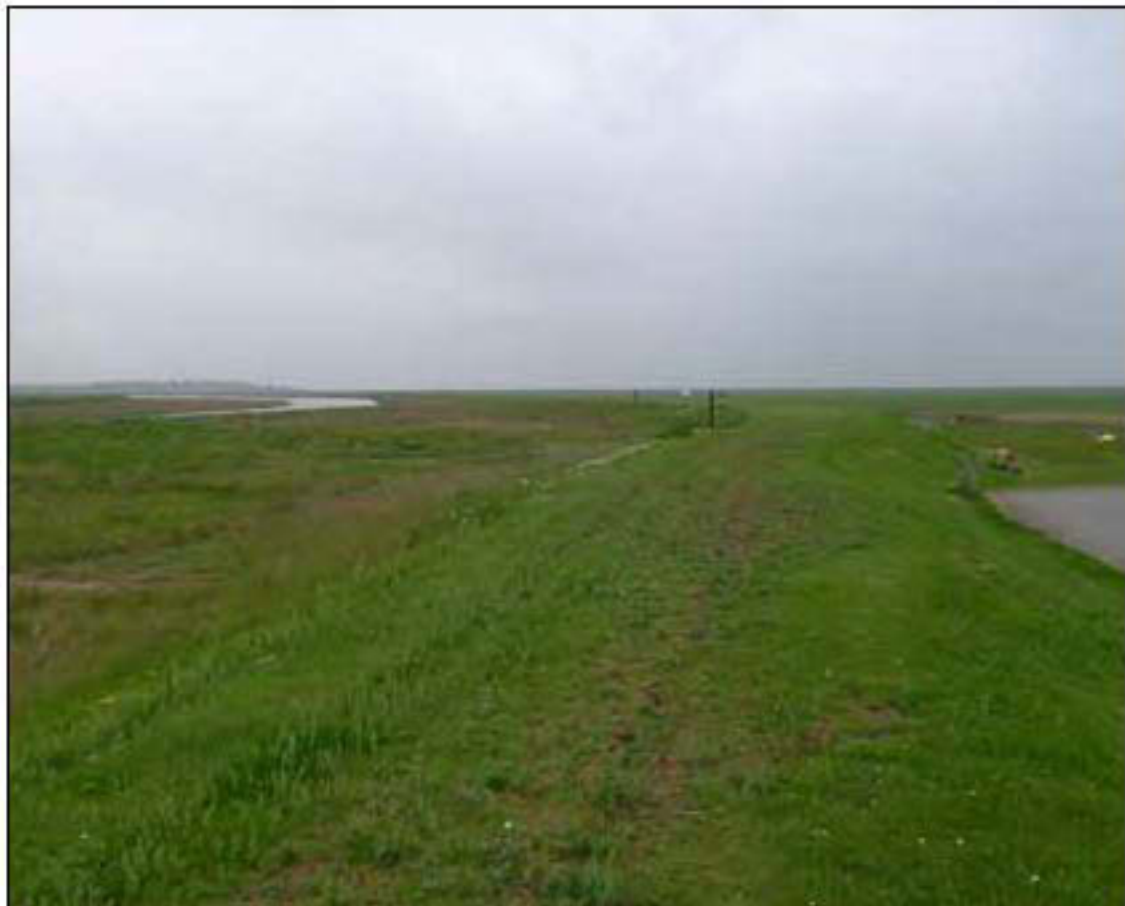
Figure 5B. Floodbank, looking northwest, from top of bank level with gantry path.
