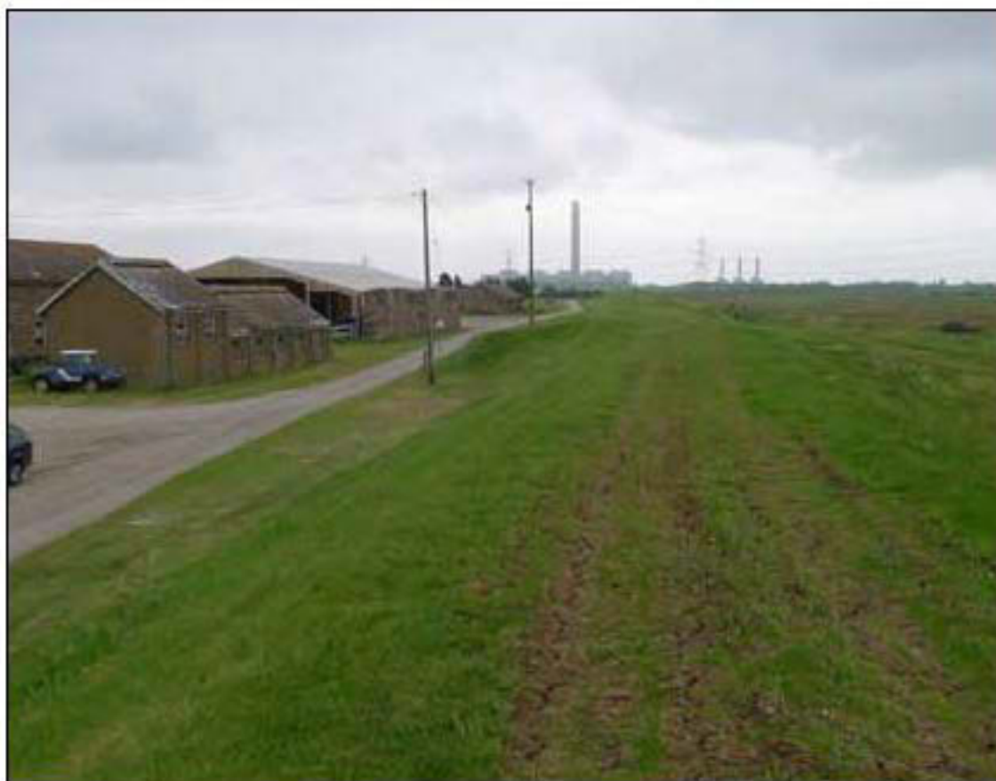
Figure 57. Floodbank, looking south-east, from top of bank level with gantry path.
