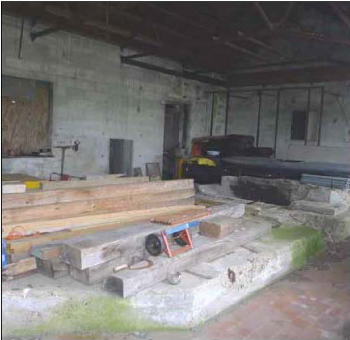
Figure 31. Interior of powerhouse.
