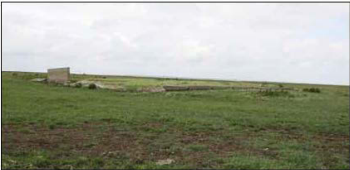
Figure 54. Rosecourt Barn from the east.
