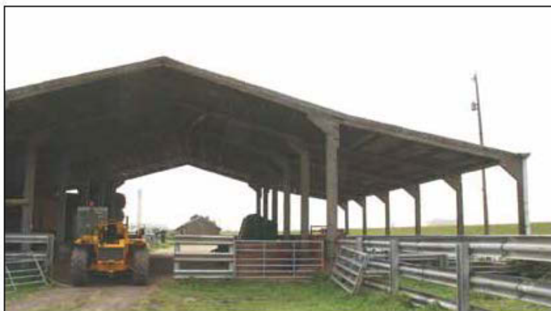
Figure 59. Recently constructed agricultural shelter, framing the powerhouse, taken from the north-west.
