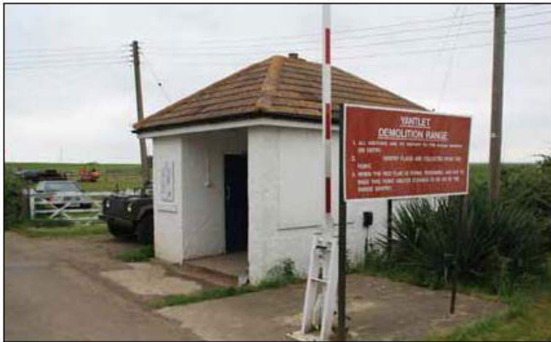
Figure 24. Guardhouse and barrier from the southeast.
