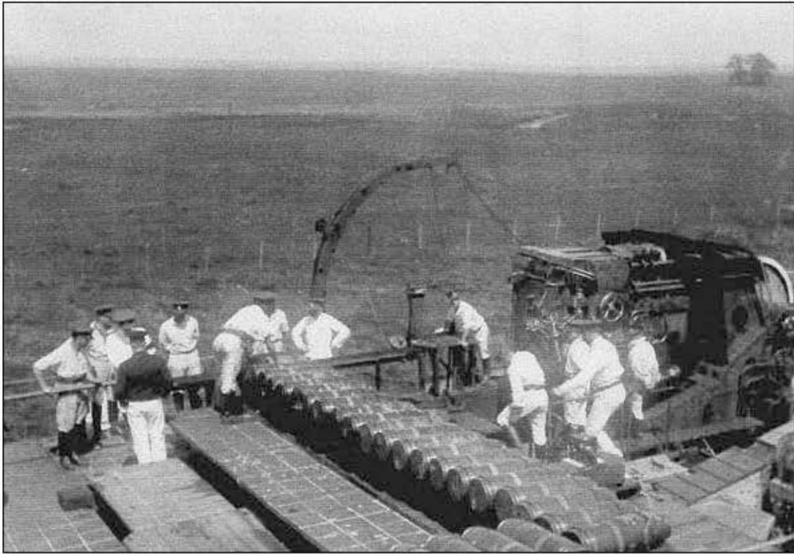
Figure 67. Loading of gun with weighted (non-explosive) shells during a 'Rapid' (fire) trial of a naval 12in breach-loading gun, looking north, 1933-38, © The Shoeburyness Military Archives.
