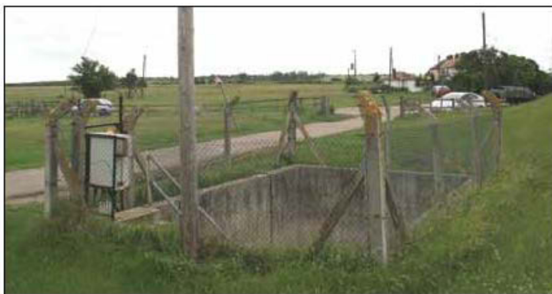
Figure 28. Concrete tank next to road, looking towards the south-east.
