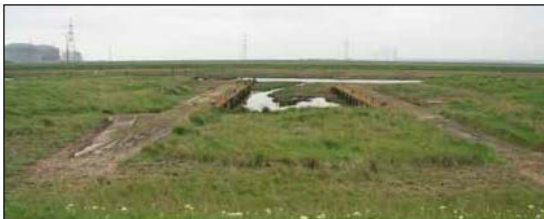
Figure 43. Dock, from bank, looking south-west.
