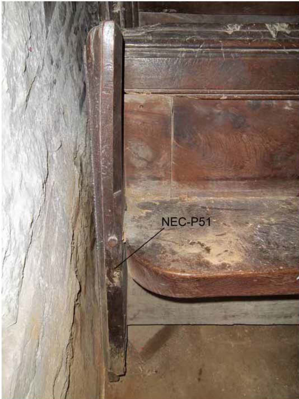
Figure 38: Photograph to show the location of sample NEC-P51 (Robert Howard)
