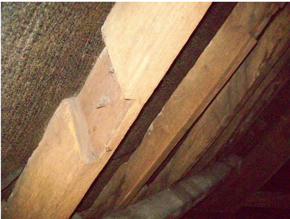
Figure 10: The roof above the Stairway, one of the reused timbers (Alison Arnold)
