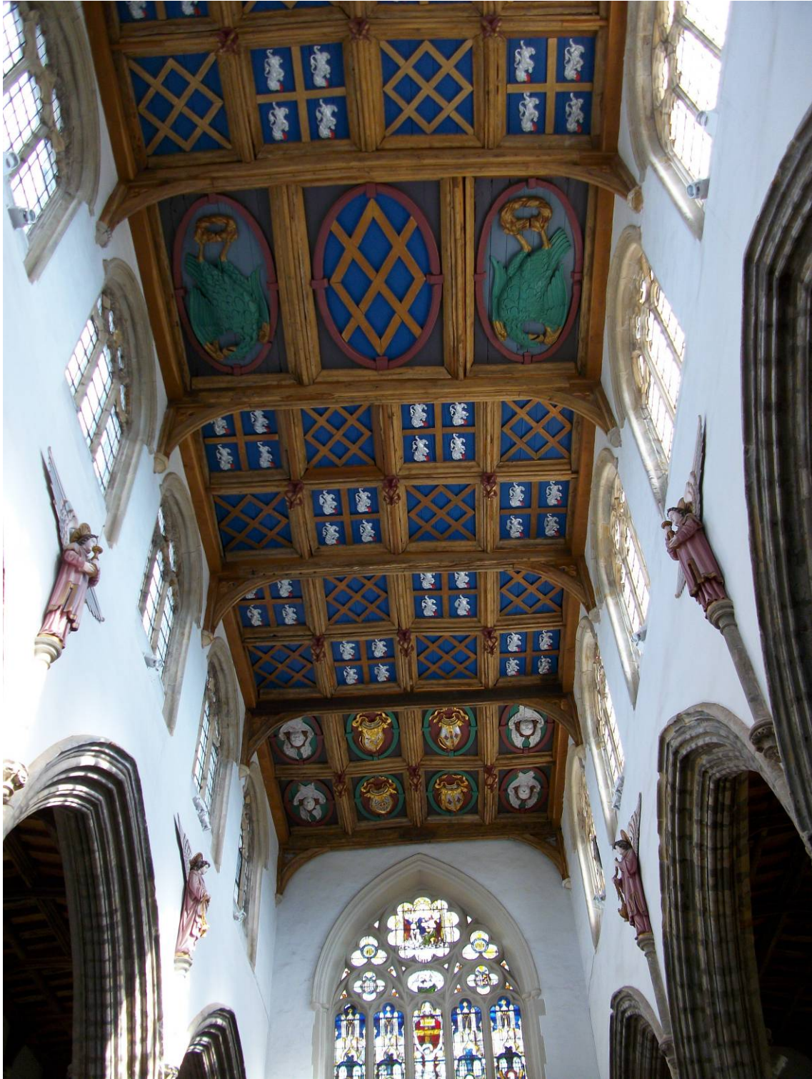
Figure 14: Chapel; nave ceiling (Alison Arnold)
