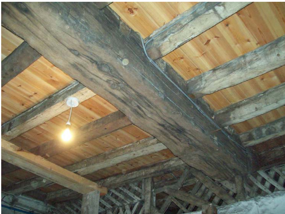
Figure 12: Gate Lodge cellar ceiling, looking south-west (Alison Arnold)
