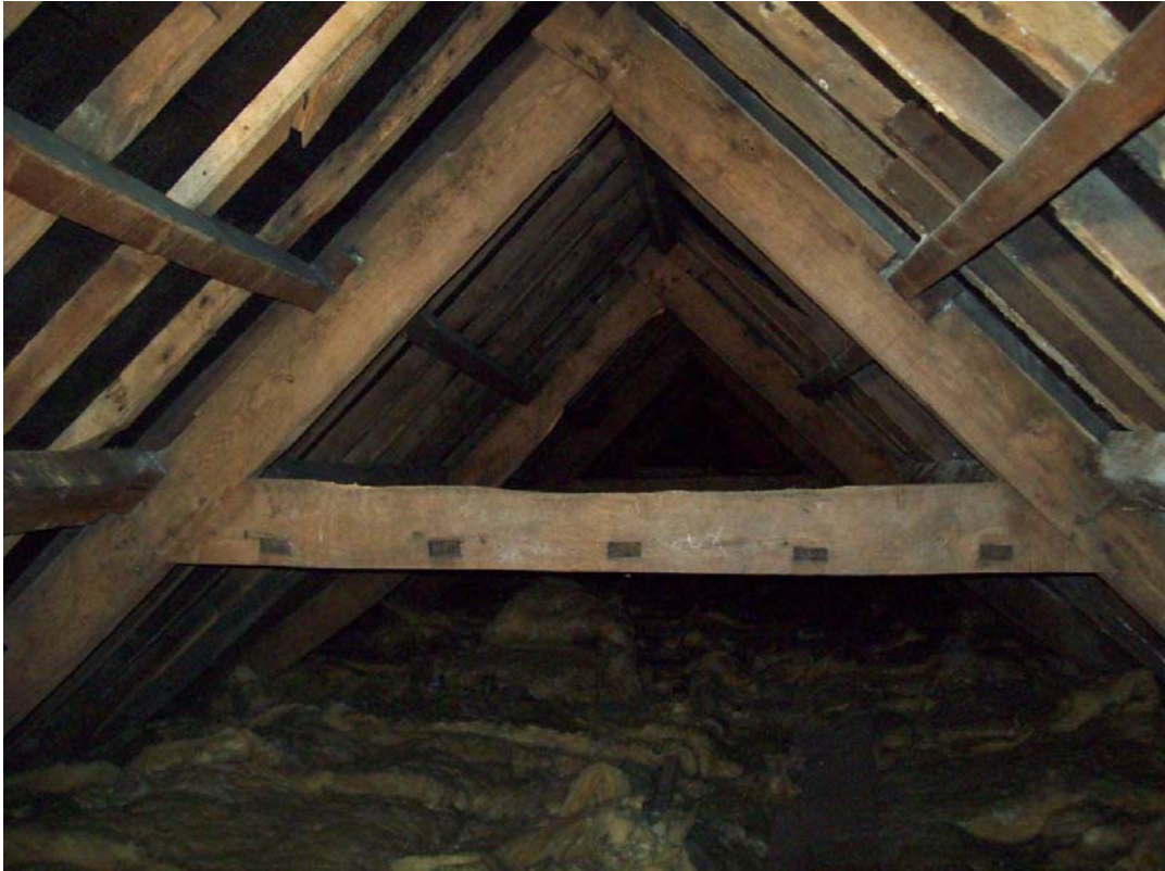
Figure 13: Scotland wing roof, looking west (Alison Arnold)
