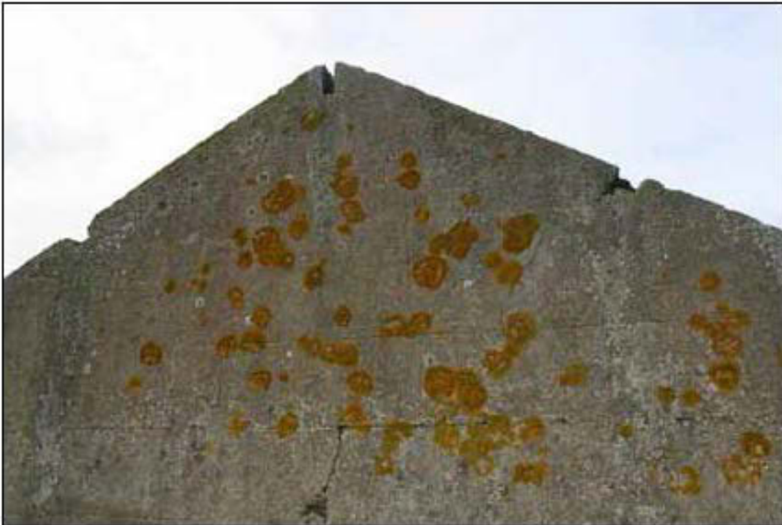
Figure 8: Gable end of a magazine showing the 'ashlar pattern' incised into the concrete render and the three slots which carried the roof purlins.
