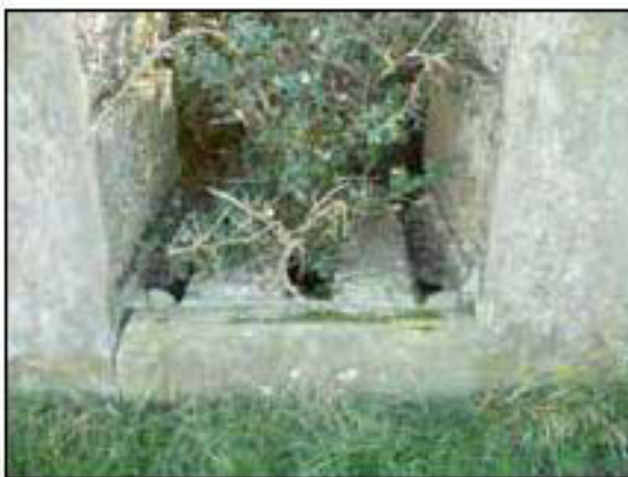
Figure 16B: Concrete floor supports within the entrance porch.
