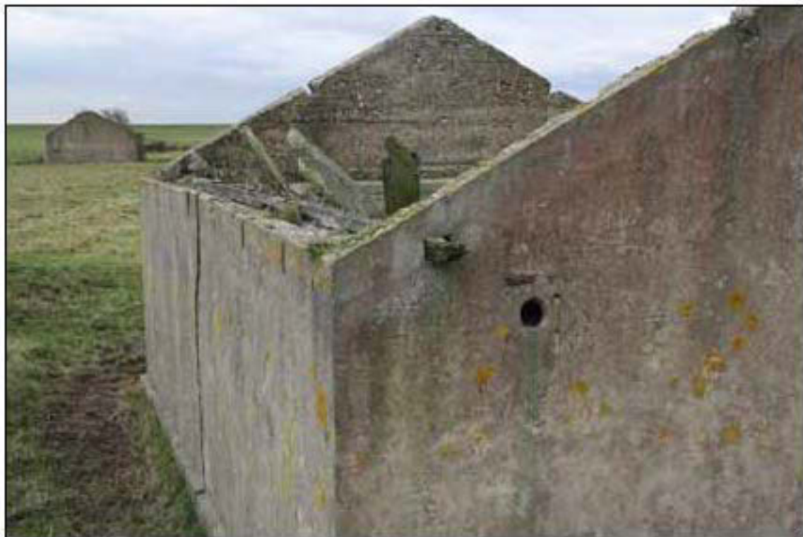
Figure 10: Surviving roof timbers in the magazine to the extreme south-east of the site indicate the position of the pole plate which protruded through both gables and carried the rafters. Evidence for some form of cover over the ventilation pipe in the east elevation is also visible
