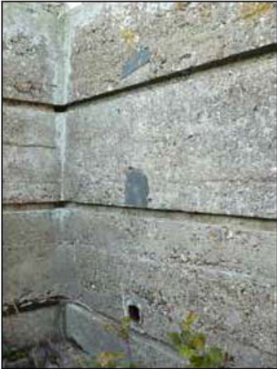
Figure 15: The internal slots which carried batons on to which wooden anti-spark 'match-lining' would have been fixed. Pieces of slate can be seen embedded in the interior face of the southern wall above a ceramic pipe. This may be related to the external concrete ventilation shaft seen on the southern elevation of some of the magazines.
