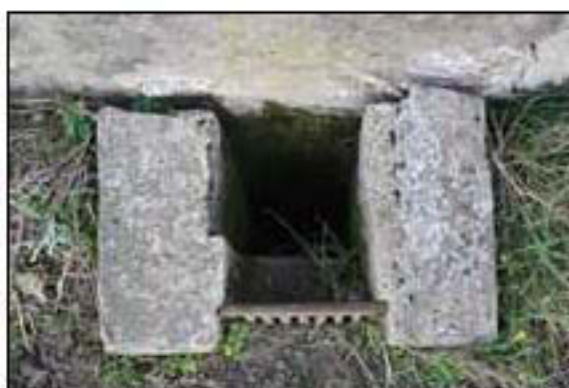
Figure 12B: A concrete ventilation shaft with the cap removed.
