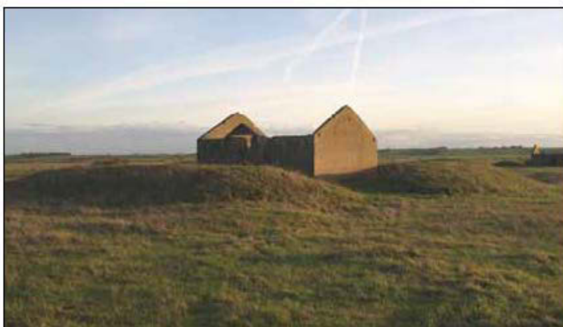
Figure 17: A surviving example of the earthwork bund which originally protected all the magazines (eastern of central two magazines).
