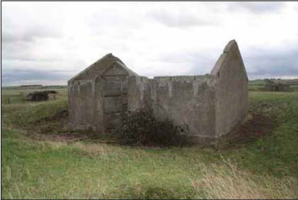
Figure 7: An example of a typical magazine building (eastern magazine in central row).
