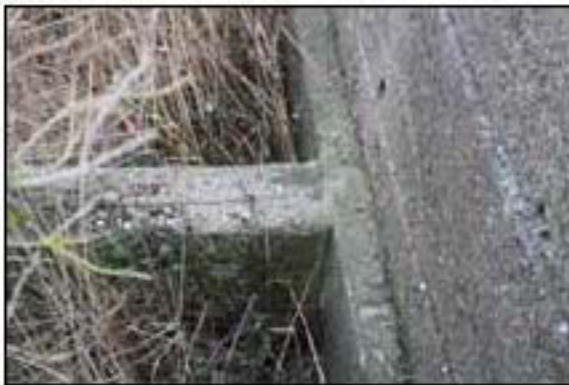
Figure 15: The internal slots which carried batons on to which wooden anti-spark 'match-lining' would have been fixed. Pieces of slate can be seen embedded in the interior face of the southern wall above a ceramic pipe. This may be related to the external concrete ventilation shaft seen on the southern elevation of some of the magazines.
