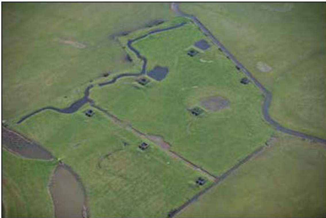
Figure 6: The magazine complex as seen from the north-west. NMR 26598/0190 6-APR-2010 English Heritage
