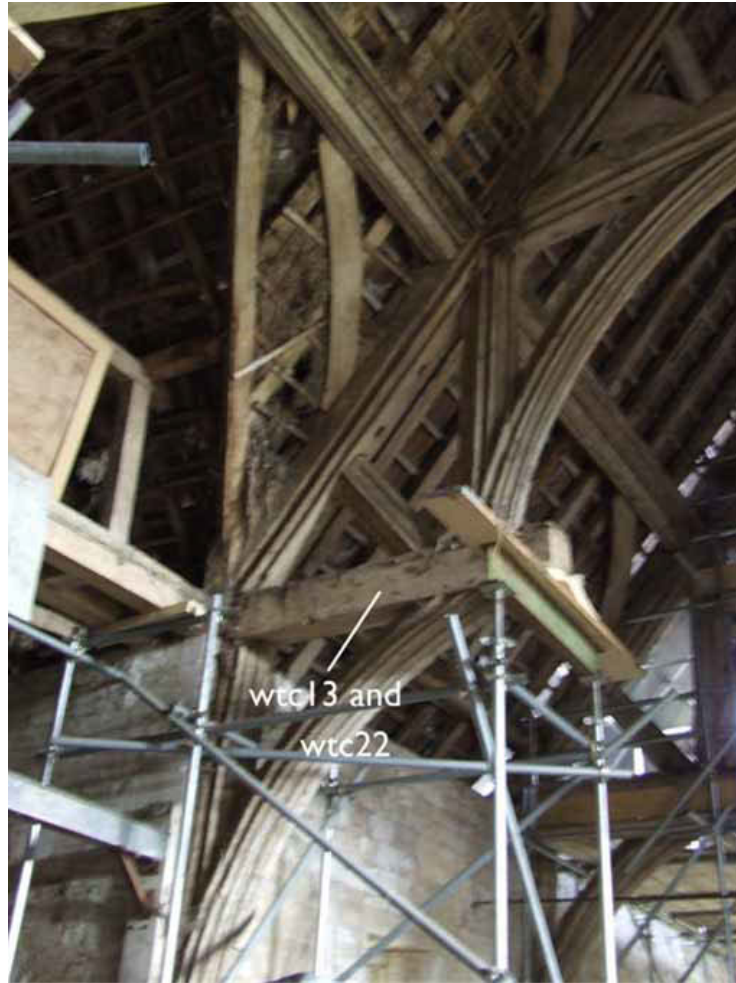
Figure 7: Photograph, looking north-east, showing the north-west side of truss 4, with the hammer beam sampled twice indicated (Martin Bridge)
