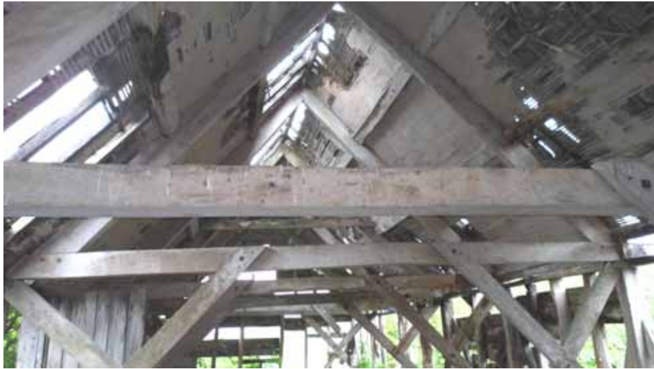
Figure 4: Main barn roof, looking north-east (Alison Arnold)
