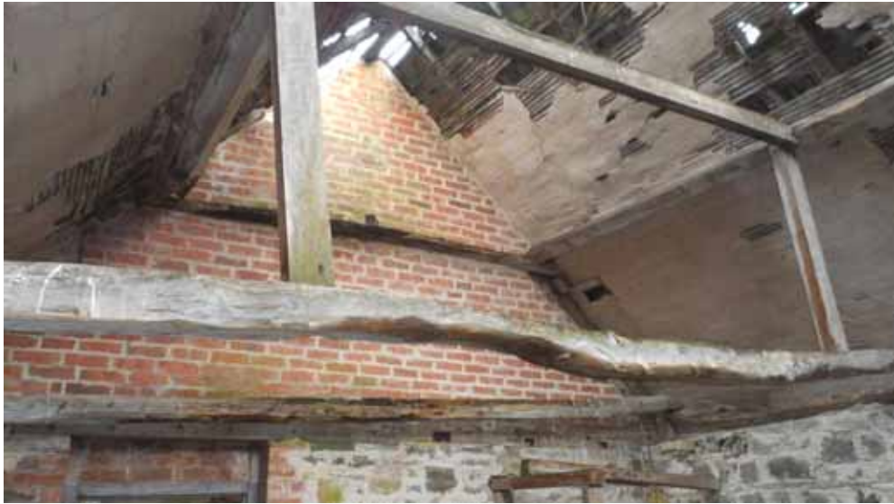
Figure 6: South extension, truss 10, from the south-west (Alison Arnold)
