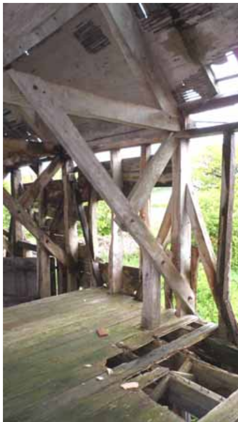
Figure 5: Main barn, later posts and bracing, from the west (Alison Arnold)
