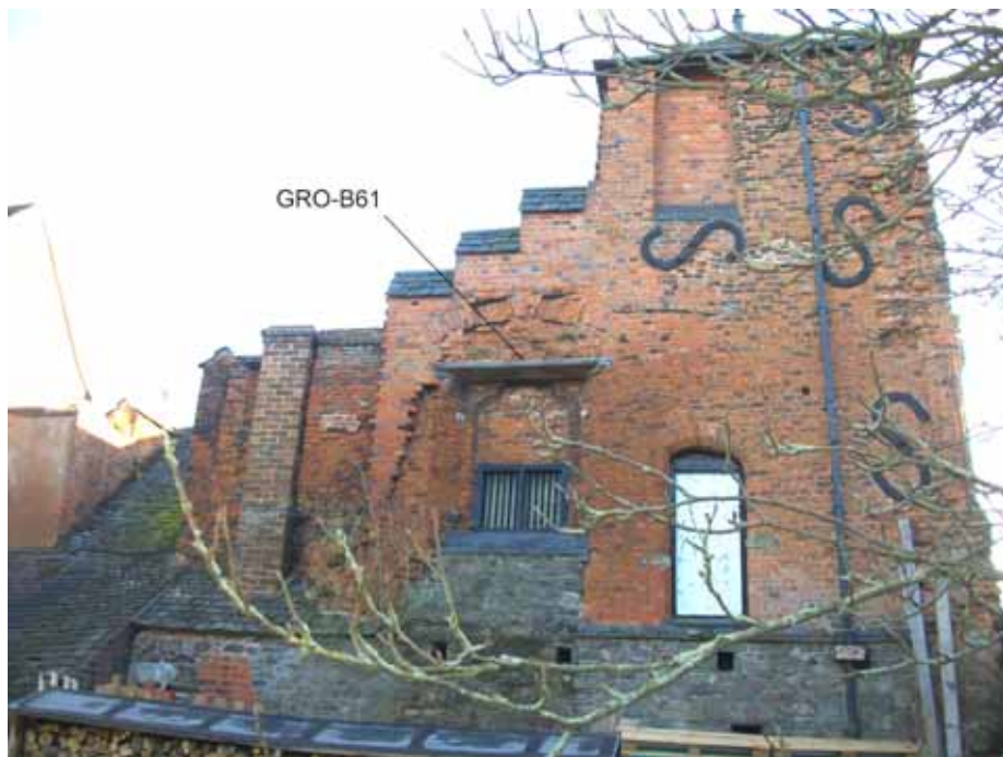
Figure 18: Remains of 'lost' range D with timber lintel (GRO-B61), photograph taken from the north-west (Alison Arnold)
