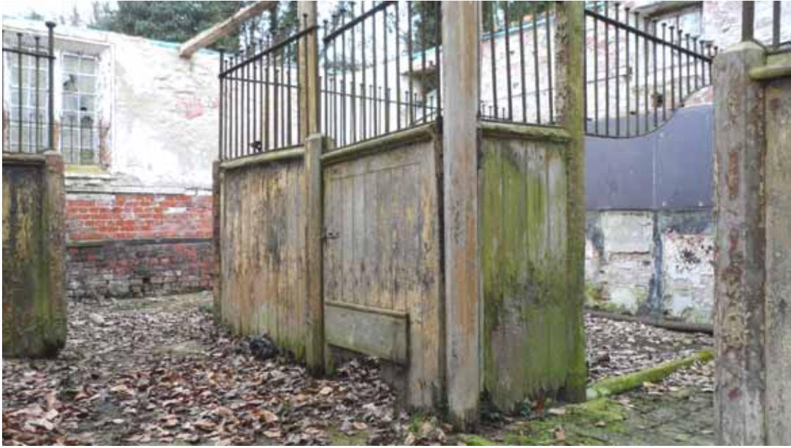
Figure 15: The stables, surviving partitioning, photograph taken from the east (Alison Arnold)
