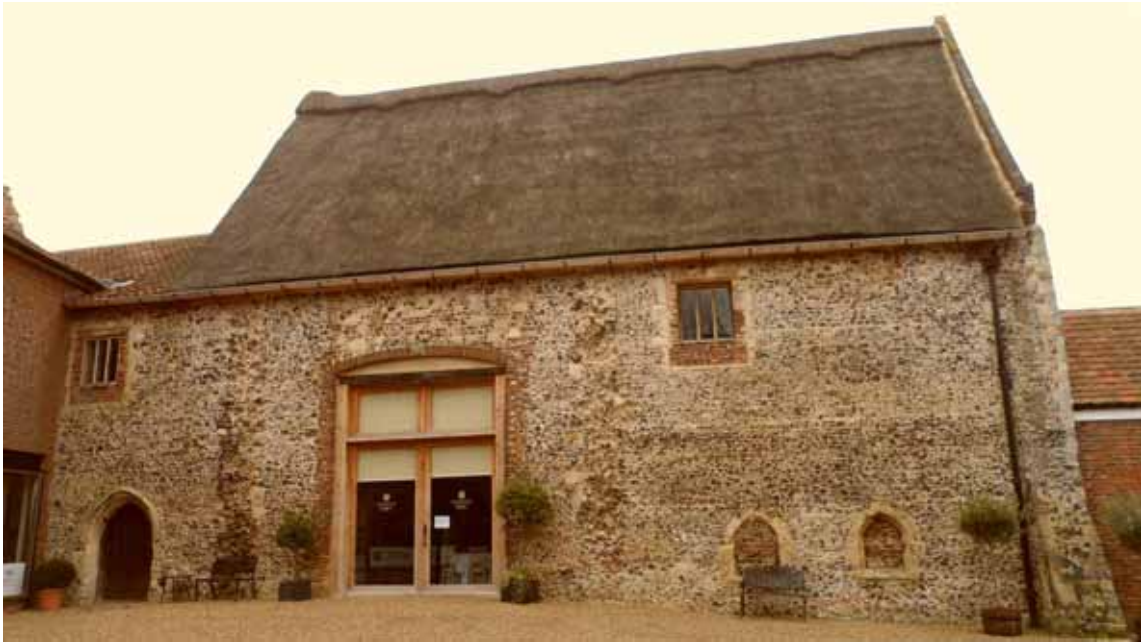
Figure 5: Former west range of the cloister, from the east (Alison Arnold)
