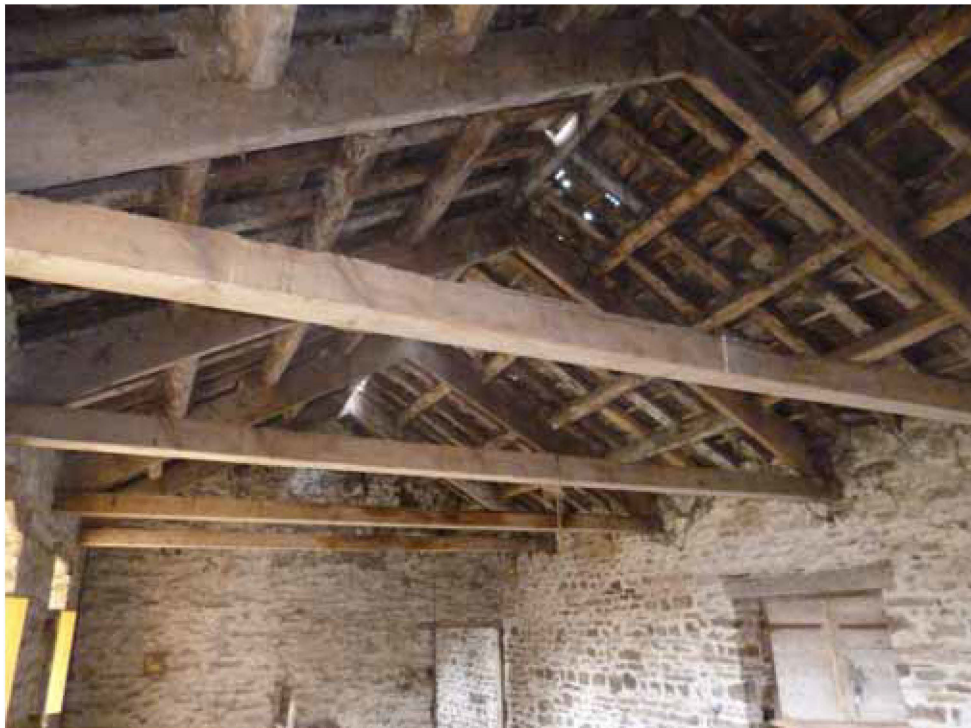
Figure 20: Stable/Coach-house range, stable roof, truss 6 in the foreground, photograph taken from the north (Robert Howard)
