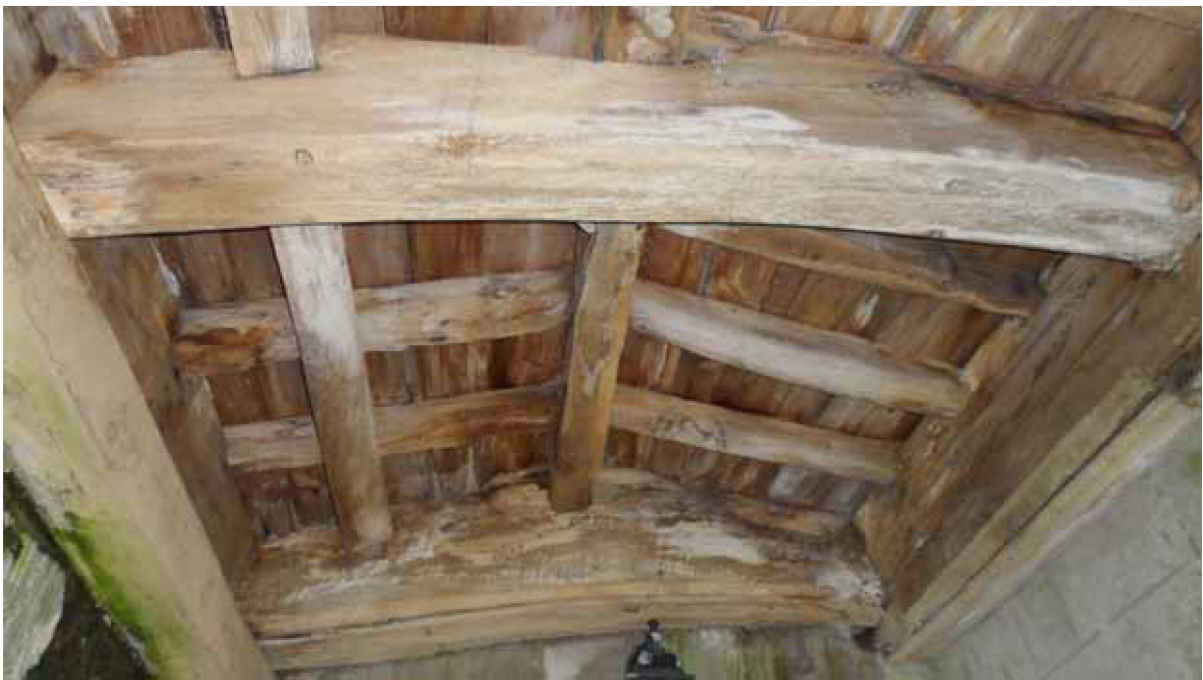
Figure 10: Porch roof, truss 2 in foreground, photograph taken from the south (Alison Arnold)
