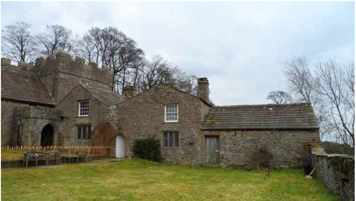
Figure 12: Service range, Kitchen to the left and cow byre to the right (Alison Arnold)
