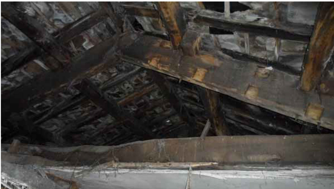
Figure 16: Service range, Tack room roof, truss 2, photograph taken from the west (Alison Arnold)
