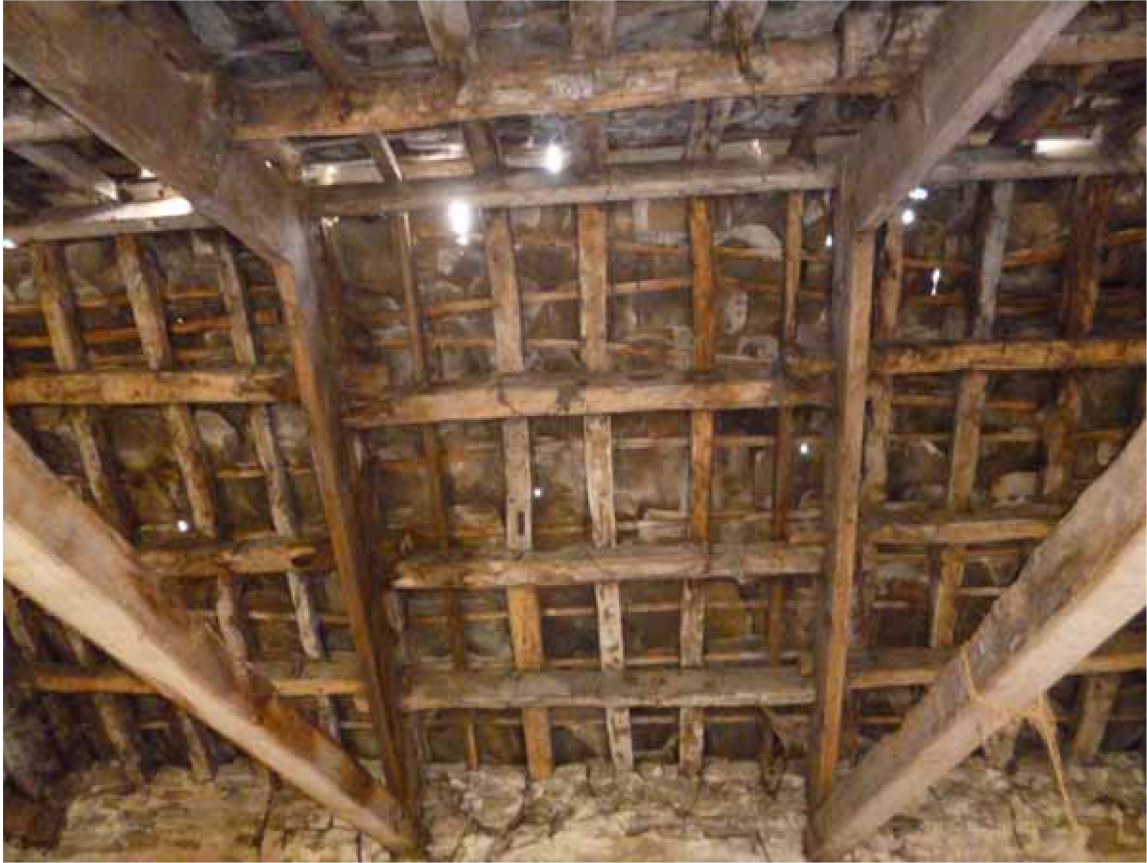
Figure 21: Stable/Coach-house range, stable roof, bay 7, photograph taken from the east (Robert Howard)
