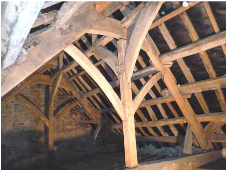
Figure 6: Hall roof, truss 2 in the foreground, photograph taken from the south-east (Robert Howard)
