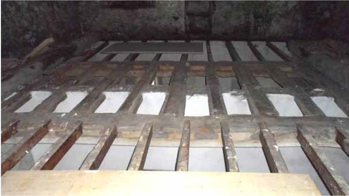
Figure 7: High-end tower, first-floor ceiling frame (from above) with main beams from the second floor lain loose by the walls (Alison Arnold)
