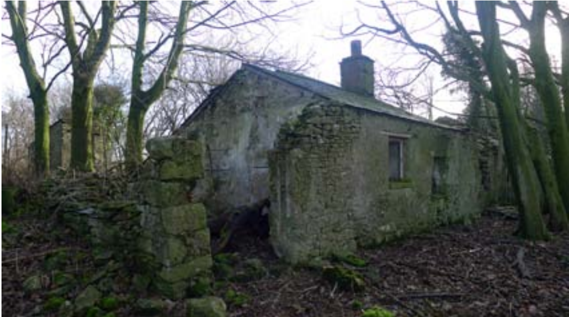
Fig 22: The ruined building (1583311) to the south of scheduled area of Dalton village, of 18th or 19th century construction, and abandoned in the first half of the 20th century. (Photograph: Dave Went).
