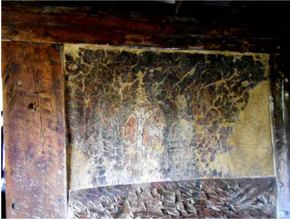
Figure 3: Painting of a saint extending onto the timber framework (Martin Bridge)
