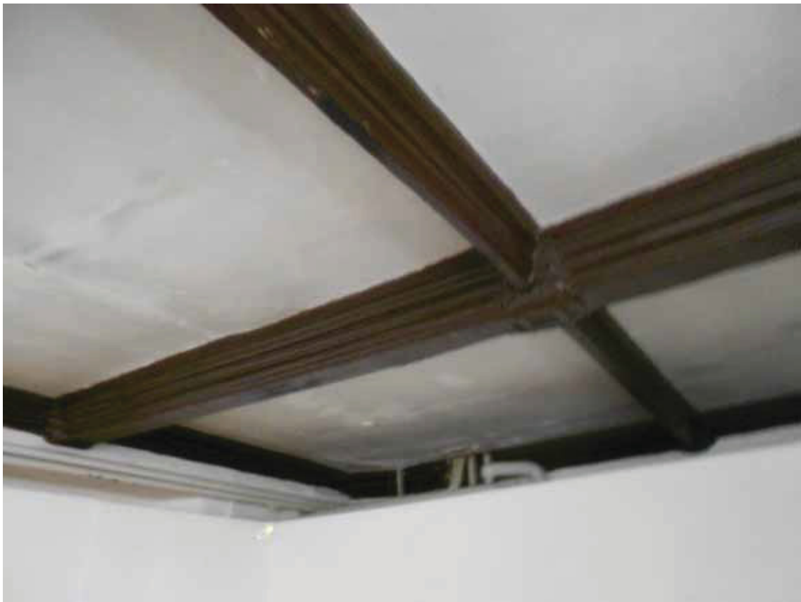
Figure 4: View of the ground-floor ceiling beams . (Photograph Martin Bridge)
