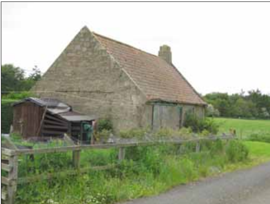
Figure 40: The smithy on the approach to Heaton Mill (© English Heritage, photograph: Clare Howard).
