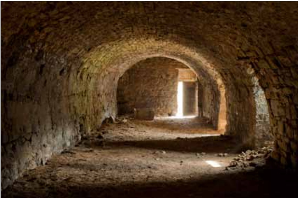
Figure 19: The tunnel-vaulted ground floor (DPI56937 © English Heritage, photograph: Alun Bull).
