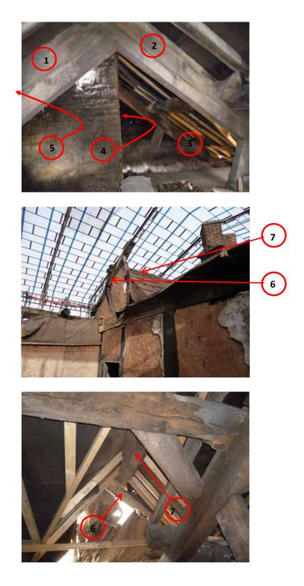
Figure 3a-c: Annotated photographs to locate sampled timbers
