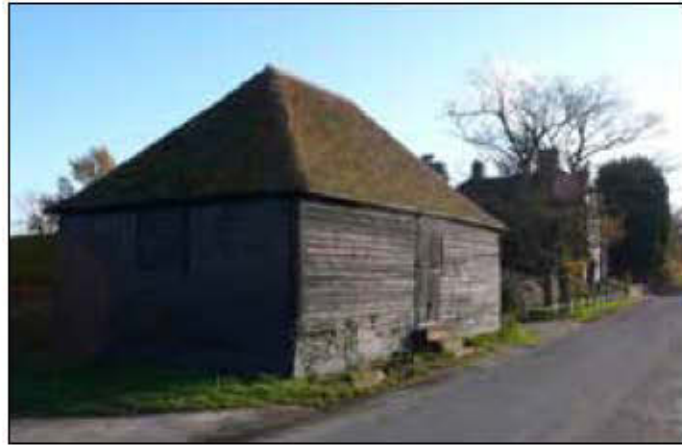
Figure 28 Court Lodge Farm barn in 2009 (P57330046)
