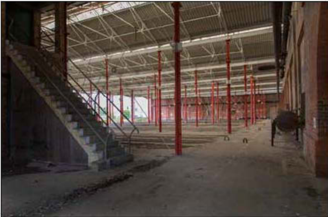
Figure 33. Interior of gunboat sheds from south, showing the stair to the upper storey of the inserted brick building (EHA DP161552)
