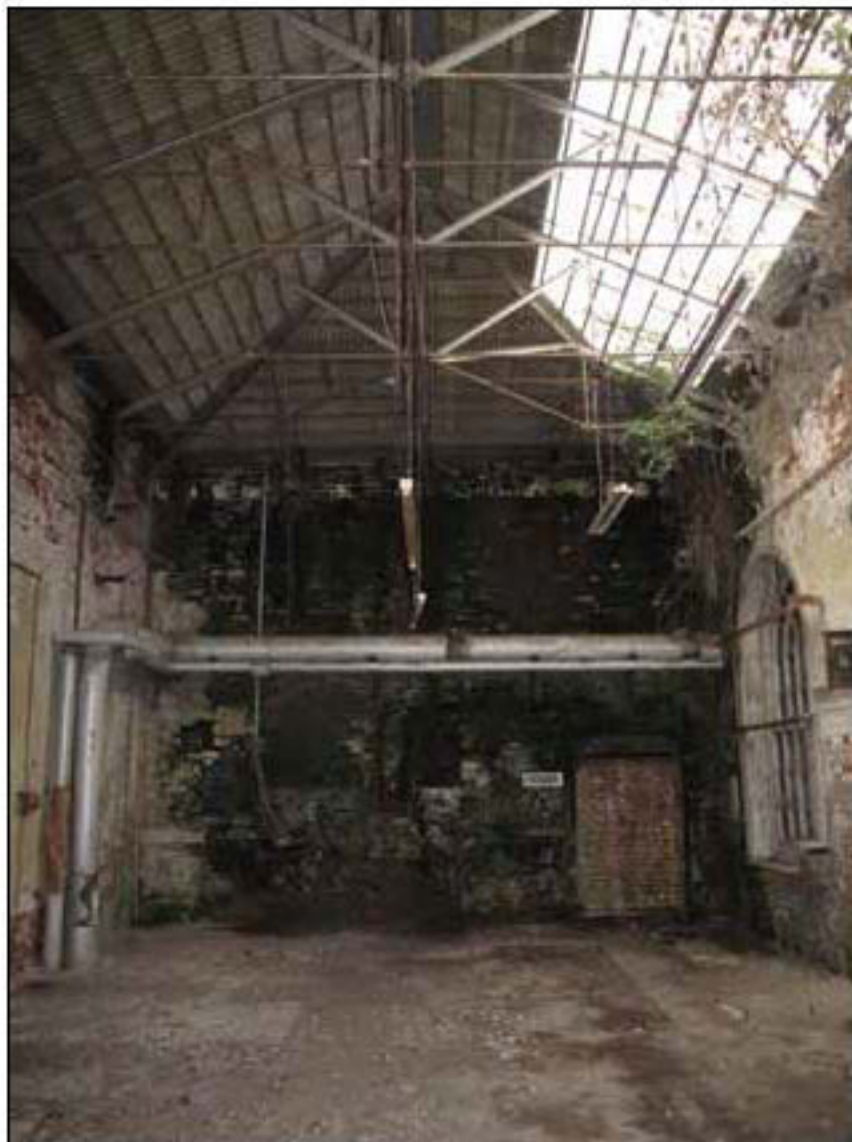
Figure 47. Interior of the engine house looking west, showing the blocked doorway to the boiler house (© English Heritage)
