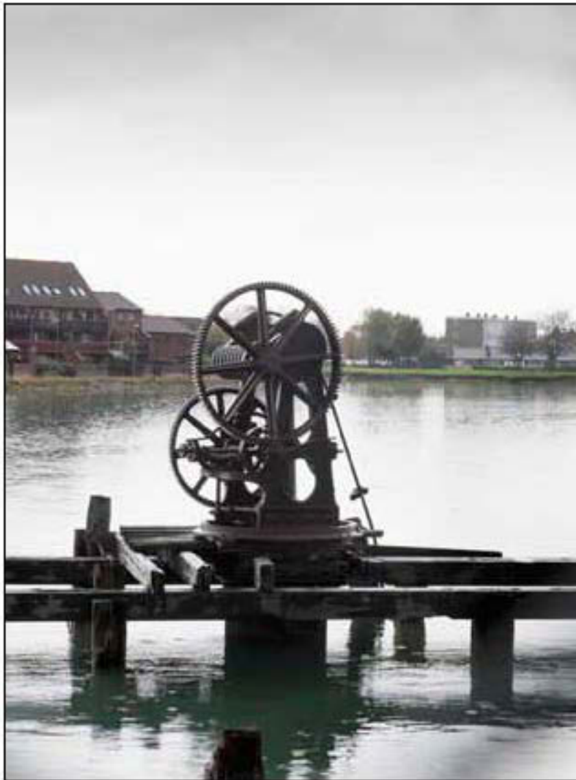
Section of timber jetty with crane (EHA DP161577)
