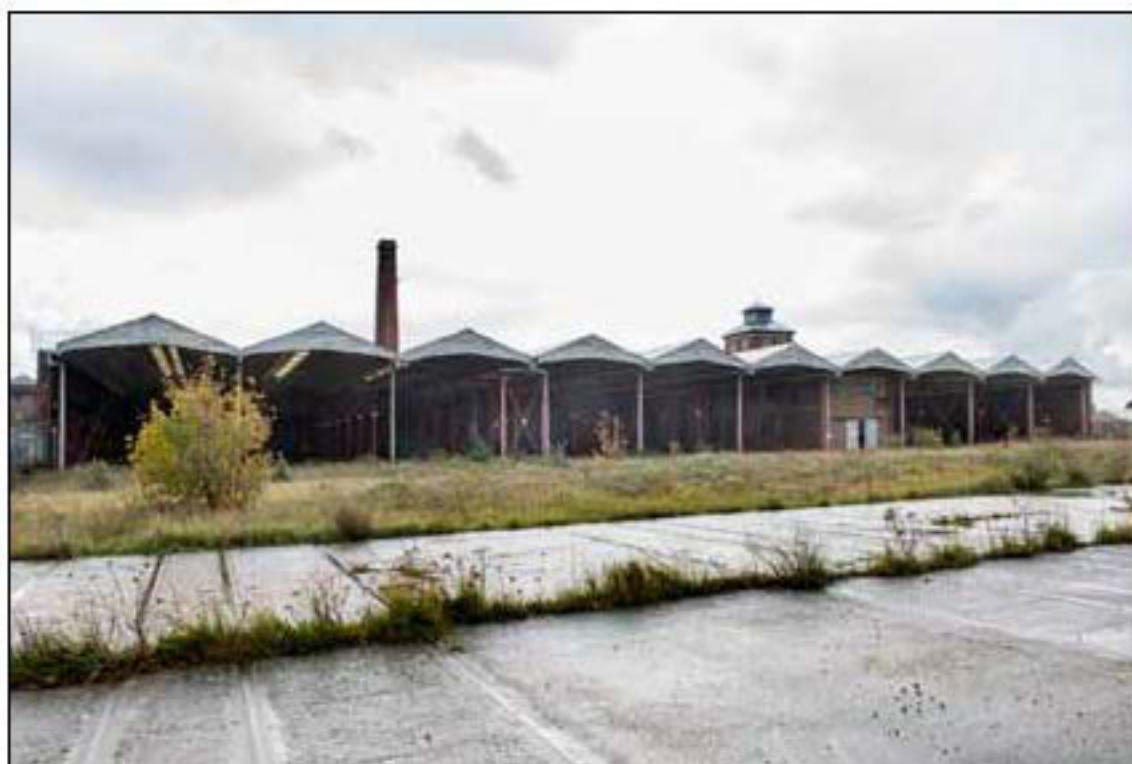
Figure 27. Gunboat sheds from the north east (EHA DP161539)
