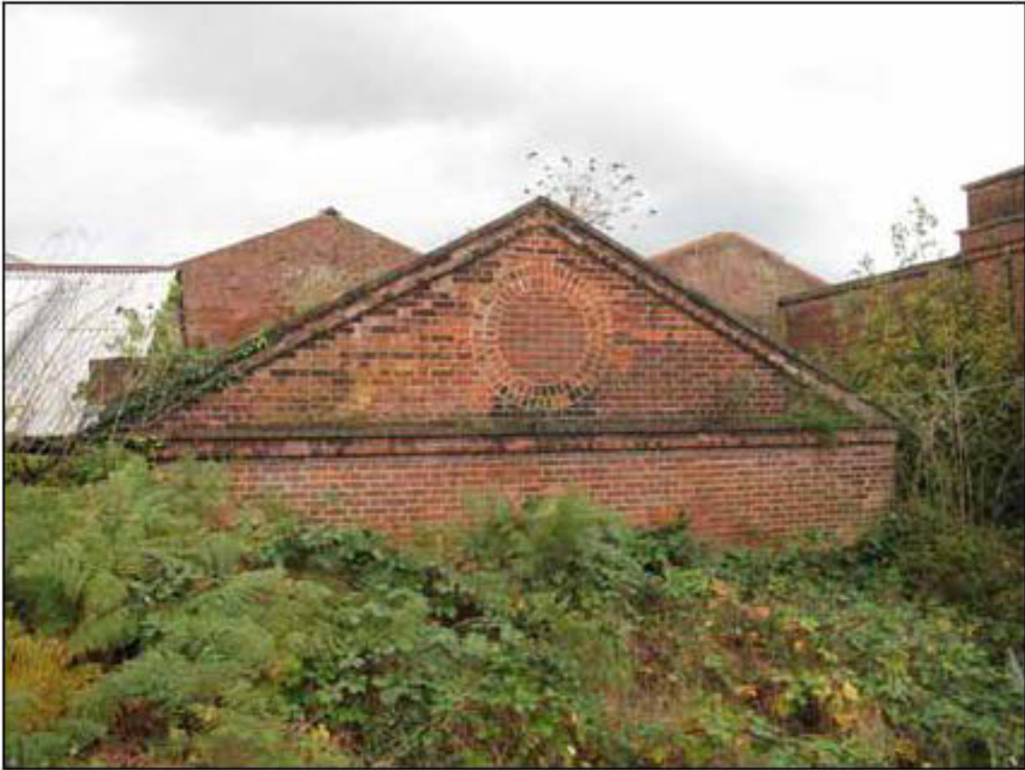
Figure 53. South elevation of the eastern maintenance shed (© English Heritage)
