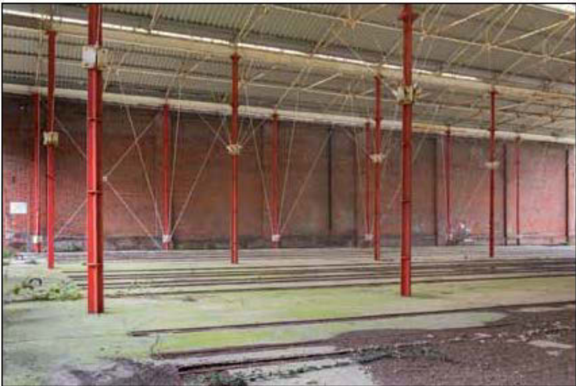
Figure 40. Rails visible in shed interior (EHA DP161551)
