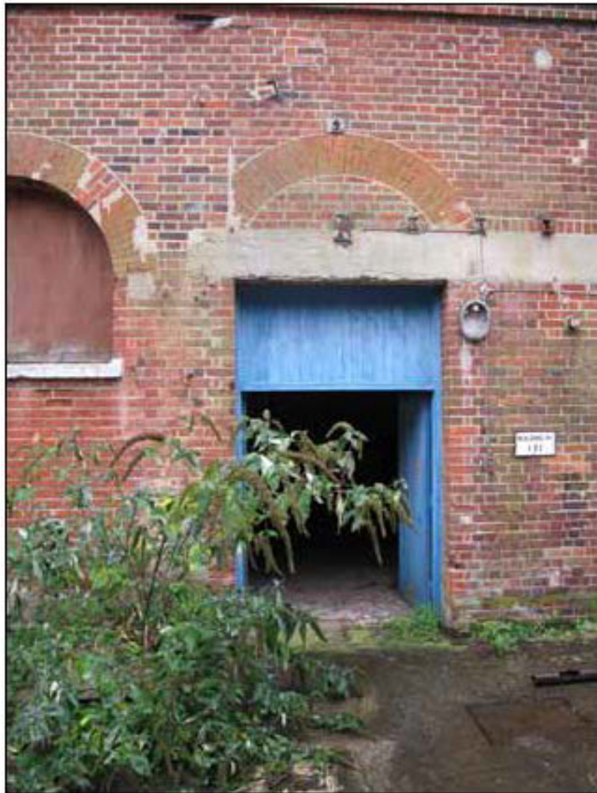
Figure 45. North elevation of the boiler house showing the inserted doorway (© English Heritage)
