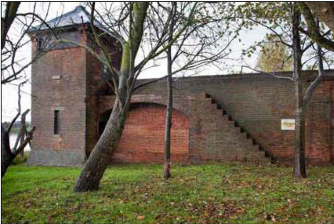
Figure 54. Southeast corner of the boundary wall, with sentry house (EHA DP161575)
