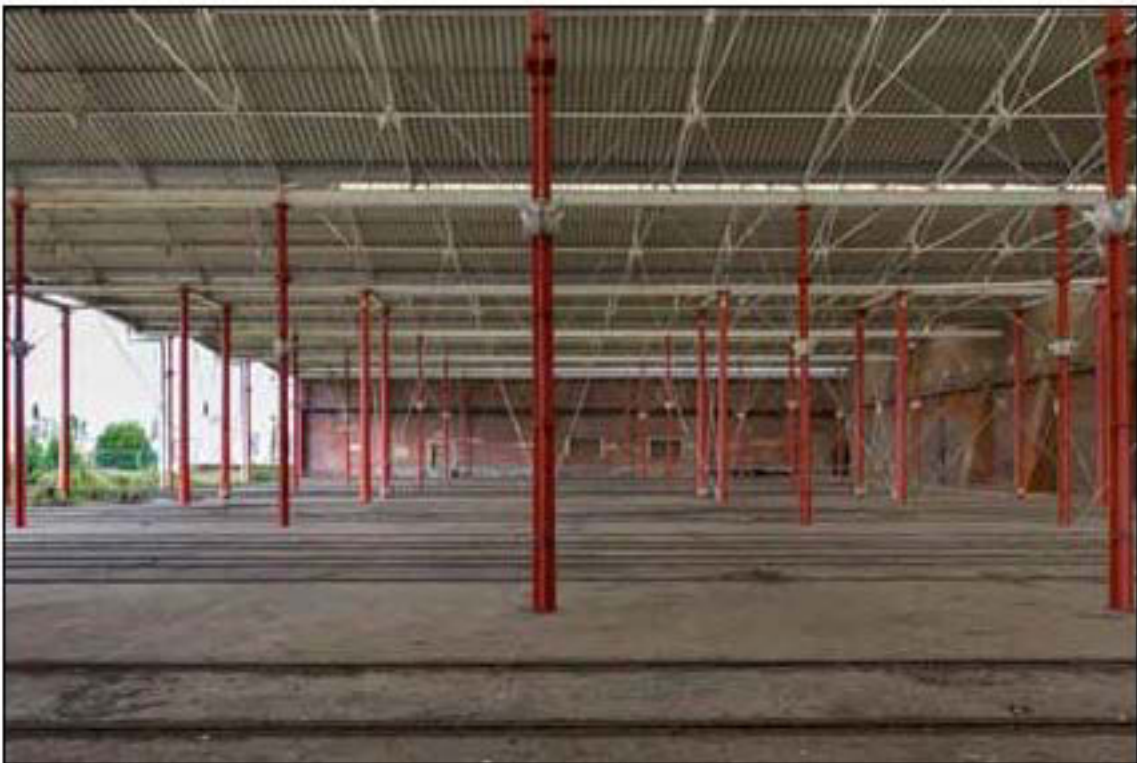
Figure 31. Gunboat sheds interior from south west (EHA DP161548)
