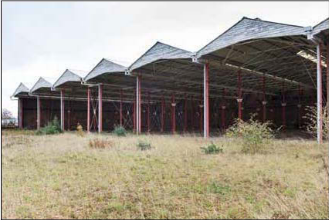
Figure 30. North face of gunboat sheds (EHA DP161536)
