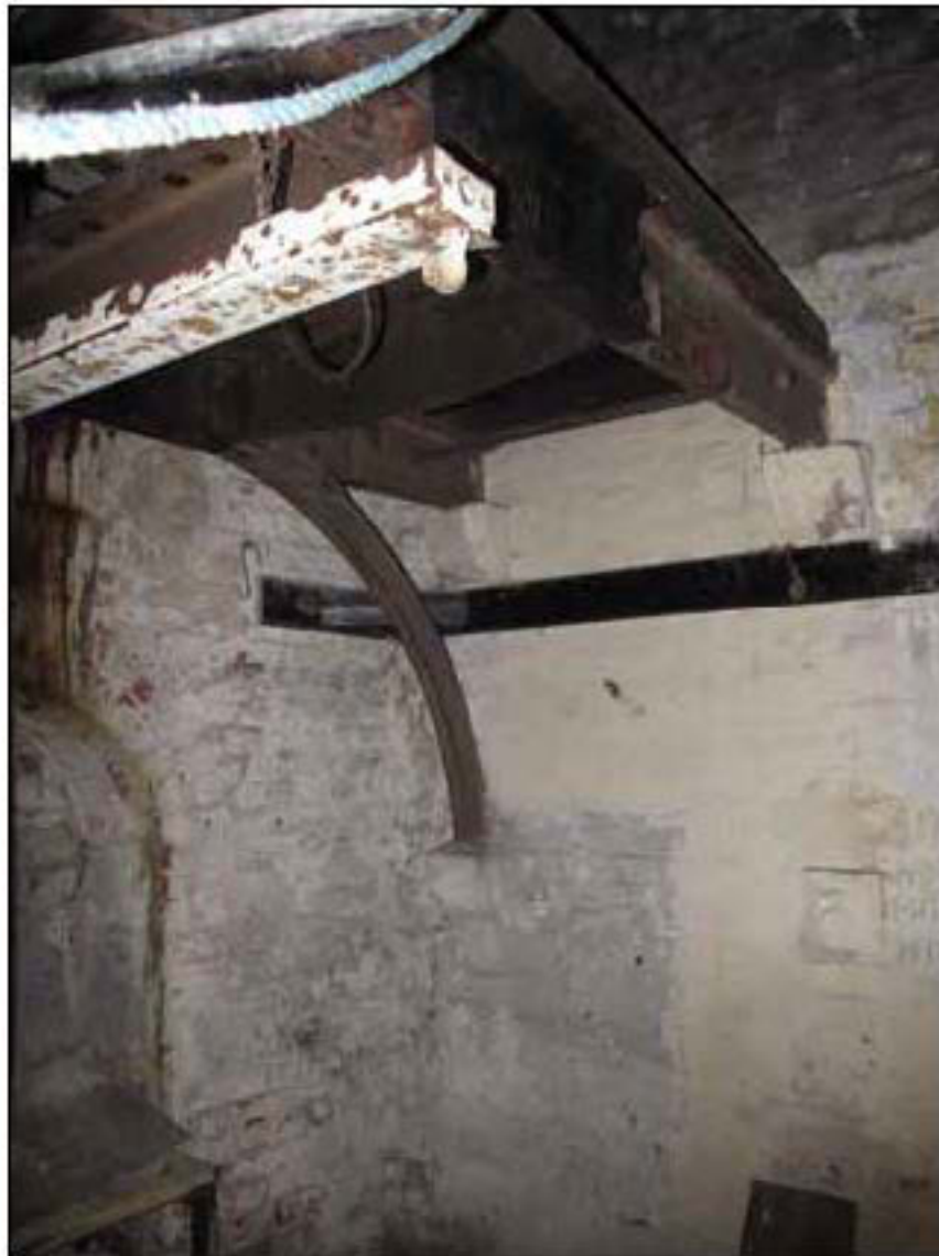
Figure 52. Interior of rebuilt well house showing part of winch mechanism (© English Heritage)
