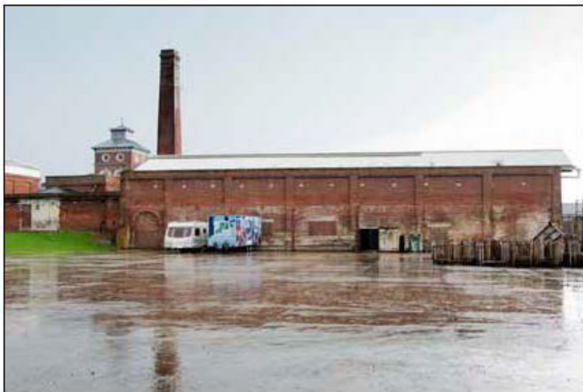
Figure 28. Gunboat sheds from the east (EHA DP161542)
