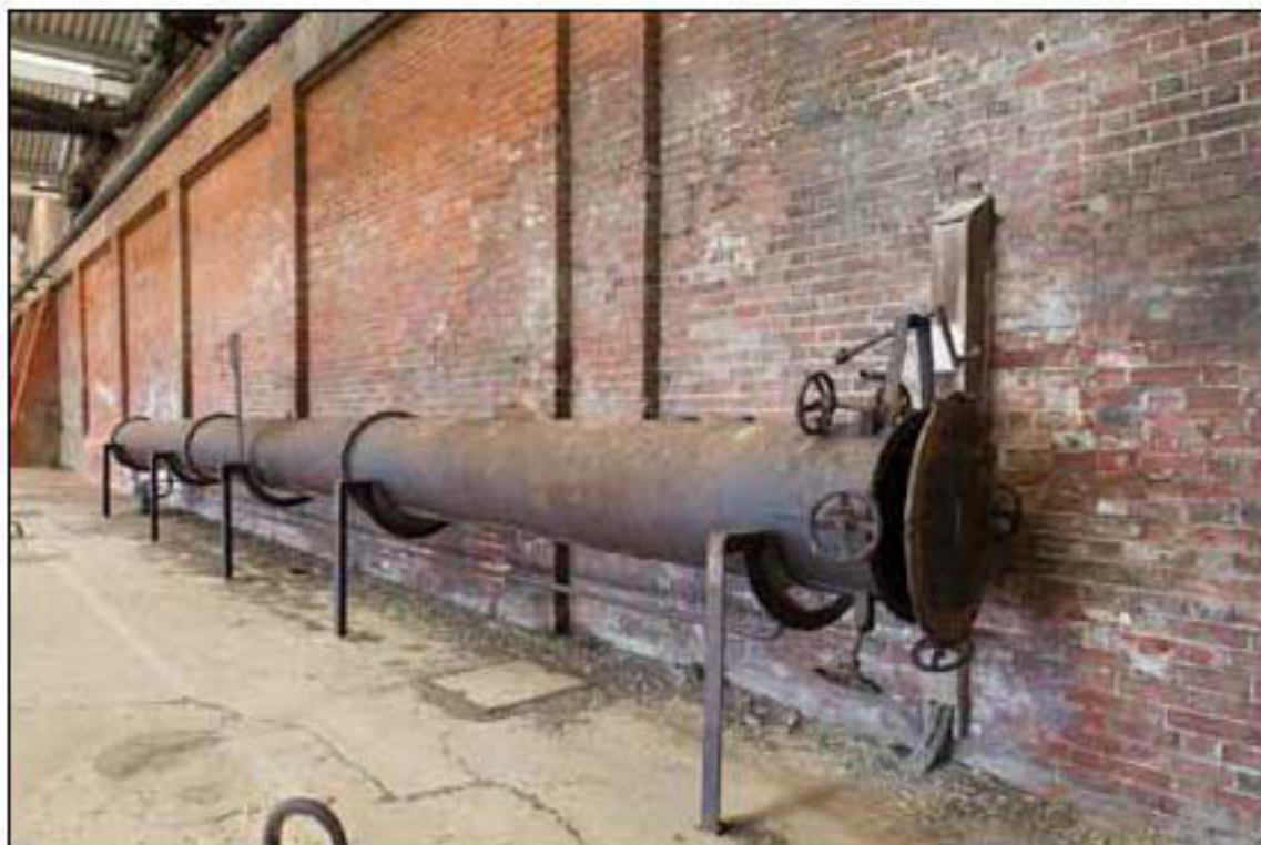
Figure 32. Steam pipe for softening wood (EHA DP161555)
