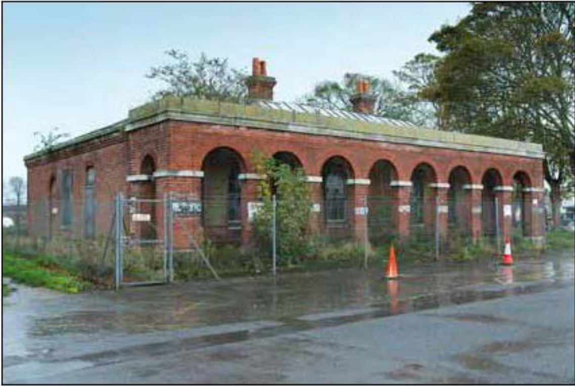
Figure 56. Former police barracks to the south of the main entrance (EHA DP161569)
