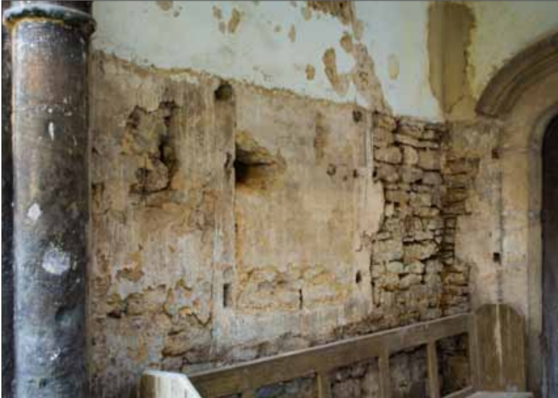
Fig 10. Blocked window in south wall of east porch (H1.04) of Great Hall, exposed by removal of panelling. (DPI61405)
