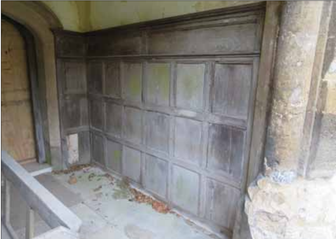
Fig 13. The east porch to the Great Hall, north wall, with panelling in situ. (N. Hill)
