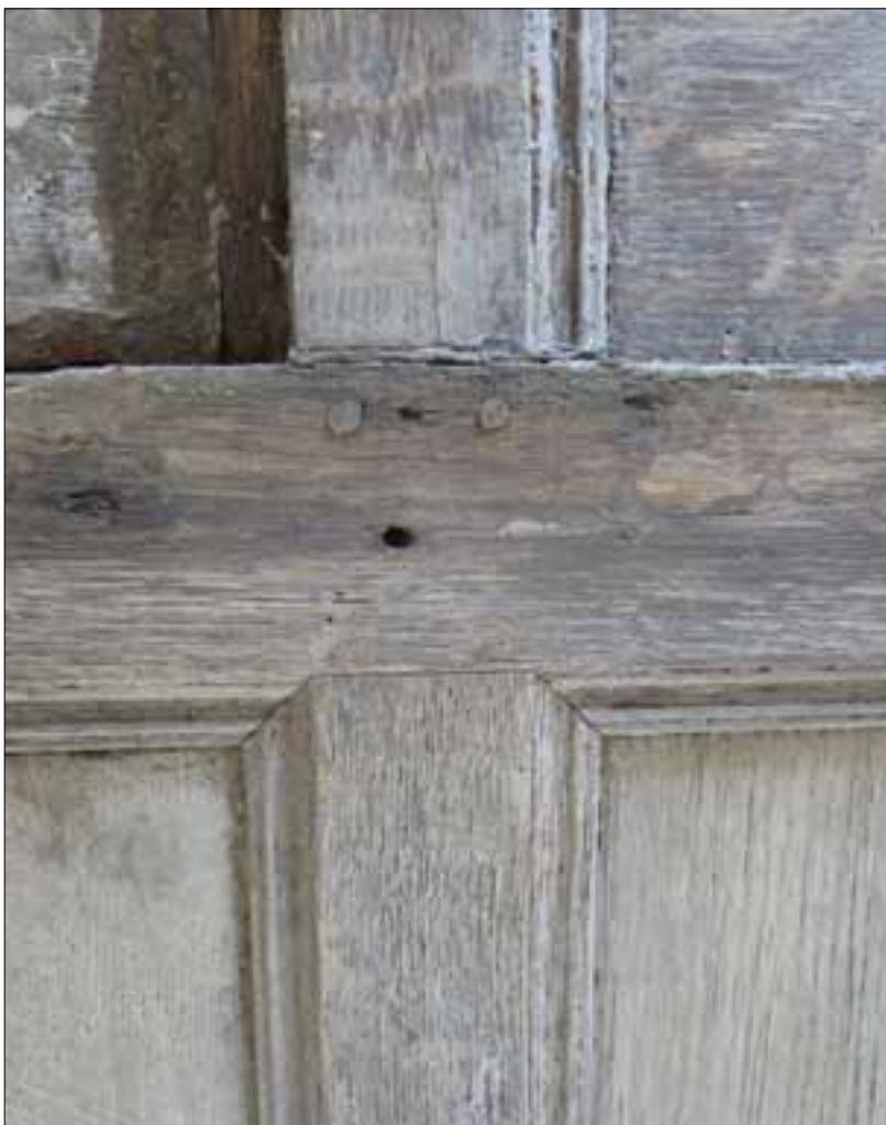
Fig 18. Detail of mitred joint to upper part of north wall panelling. (N. Hill)
