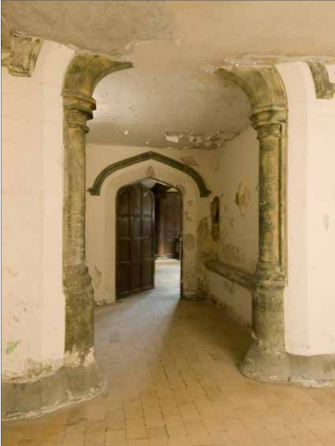
Fig 12. Surviving bench in west porch. (DP068012)
