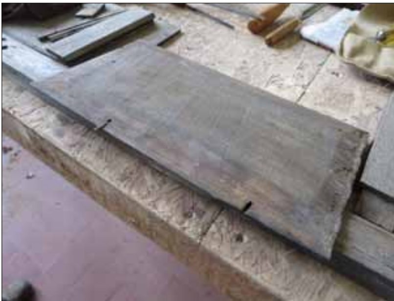
Fig 22. Dismantled section of south wall panelling, with cut-down dowel holes from previous use. (N. Hill)
