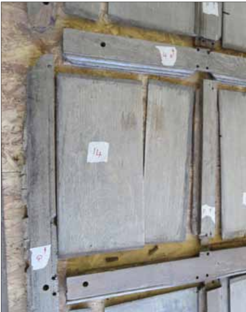
Fig 20. Dismantled section of south wall panelling, with two-piece panel. (N. Hill)
