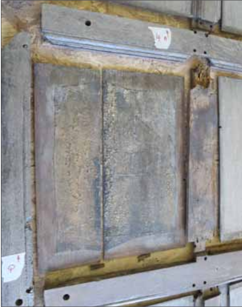
Fig 21. The rear face of the same panel (fig 20), with tar coating and rough chamfering. (N. Hill)
