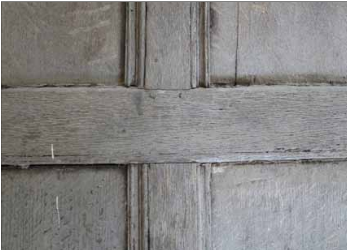
Fig 16. Detail of lower part of north wall panelling, with fine beaded and cavetto moulding to intermediate stiles, and ovolo scratch-moulding to underside of rail. (N. Hill)
