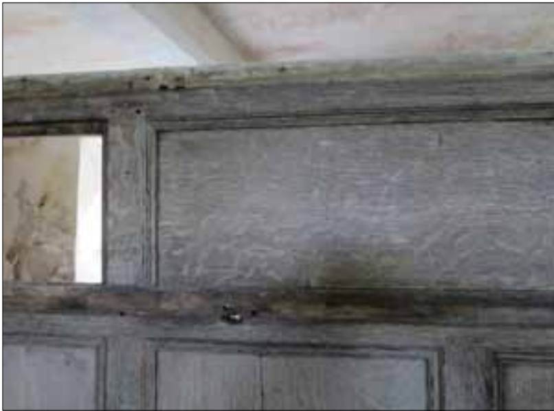
Fig 17. The upper part of the north wall panelling, with mitred joints to the top mouldings of each panel. (N. Hill)
