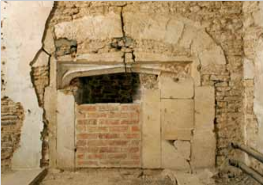
Fig 8. Fireplace in west wall of N3.05, upper chamber of gate tower. (DPI41237)
