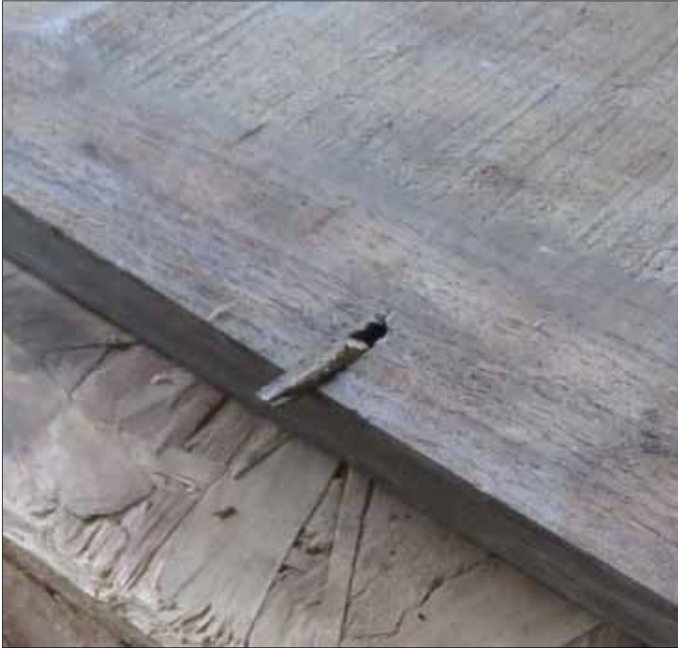
Fig 23. Detail of the same panel (fig 22), with dowel still in situ. (N. Hill)
