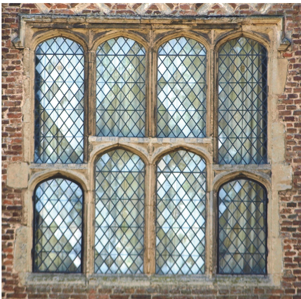
Figure 4. Oxburgh Hall, King's Room, north-facing window (exterior)
