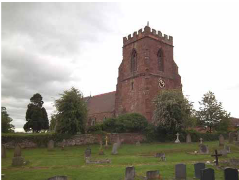
Figure 2: View of All Saints' Church from the northwest showing the buttressed and battlemented tower (photograph Robert Howard)
