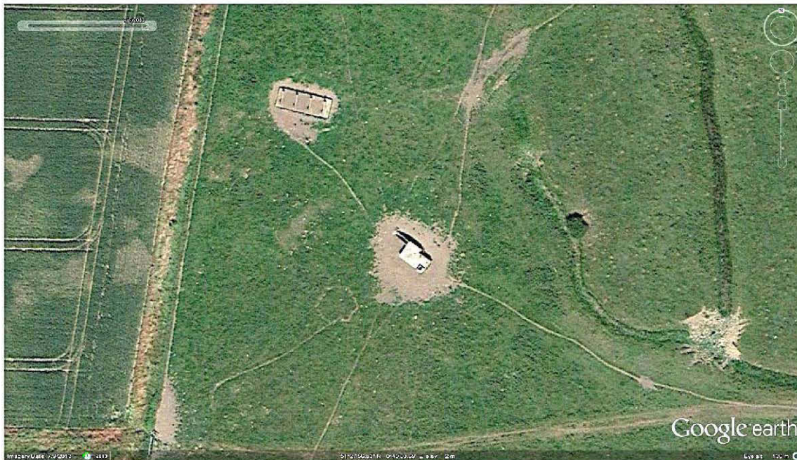
Figure 11 Remains of the remote control building with projecting blast walls (middle) and ancillary store or generator building (top left) at Allhallows decoy. (GOOGLE.EARTH.COM 2013 accessed 14-MAR-2014)
