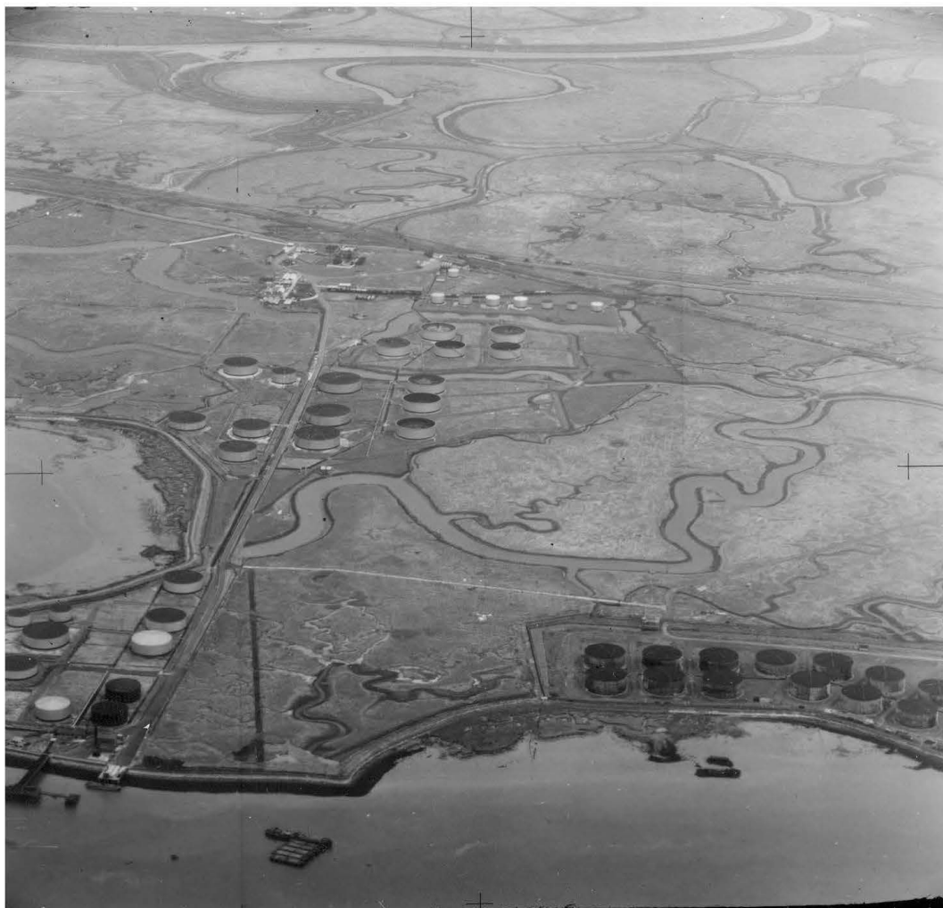
Figure 8 View of the MOSCO oil refinery (left) and Admiralty Oil Depot (right) with the Yantlet Creek and edge of Allhallows Marshes in the far distance. RAF 540/393_20_30-JUL-1950 English Heritage RAF Photography.
