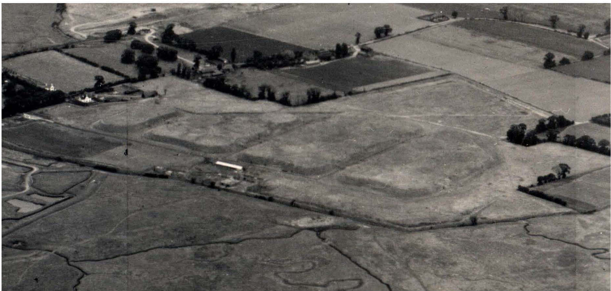
Figure 9 Soil covered oil tanks on Grain camouflaged during the Second World War. They were later incorporated into the BP refinery built there. RAF 540/393 PO-28 30-JUL-1950 English Heritage RAF Photography.
