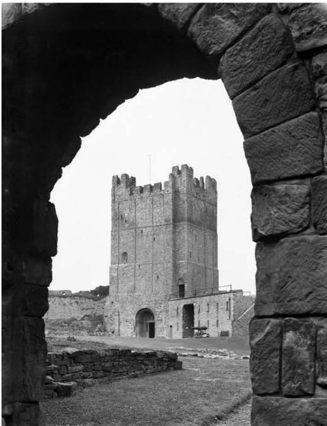
Figure 6: Richmond Castle built after the Norman Conquest on a cliff above the River Swale. Reproduced by permission of English Heritage, Reference Number: BB69/05558
