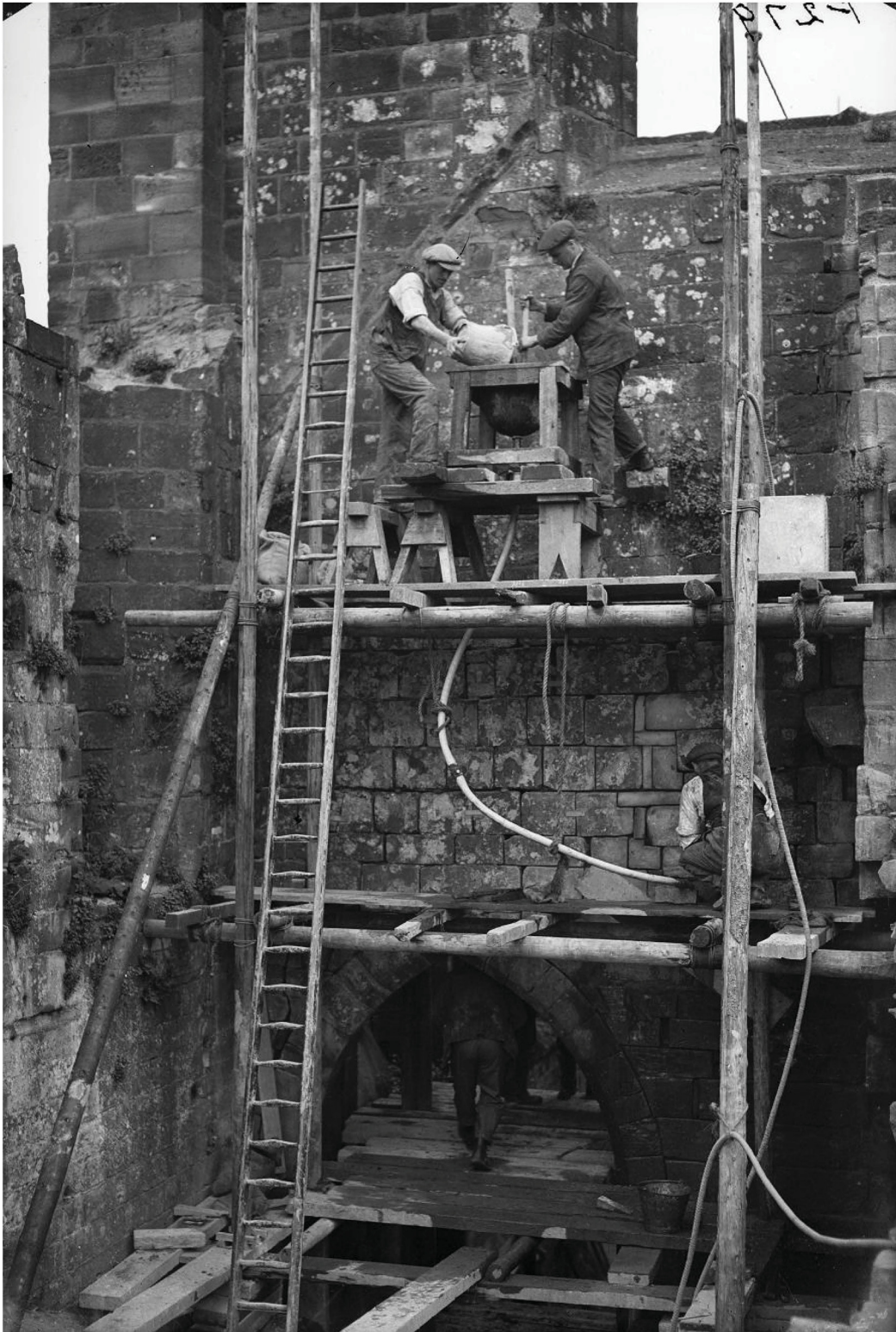
Figure 27: The gravity grouting machine being used to repair the walls at Furness Abbey, Cumbria, in the 1920s. Copyright English Heritage.
