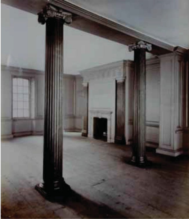
Figures 3 and 4: The interior of 75 Dean Street, Soho. Copyright The National Archives. (File: WORK 14/203)
