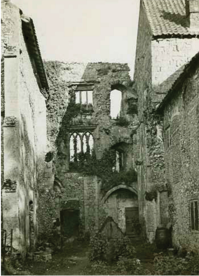
Figure 10: The shored up east wall of the dorter at Castle Acre Priory prior to guardianship. Copyright The National Archives.
