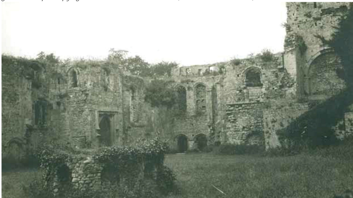
Figure 34: The Great Hall, Solar and Chapel at Portchester in the early 1920s prior to guardianship. Copyright The National Archives. (File: WORK 14/414).
