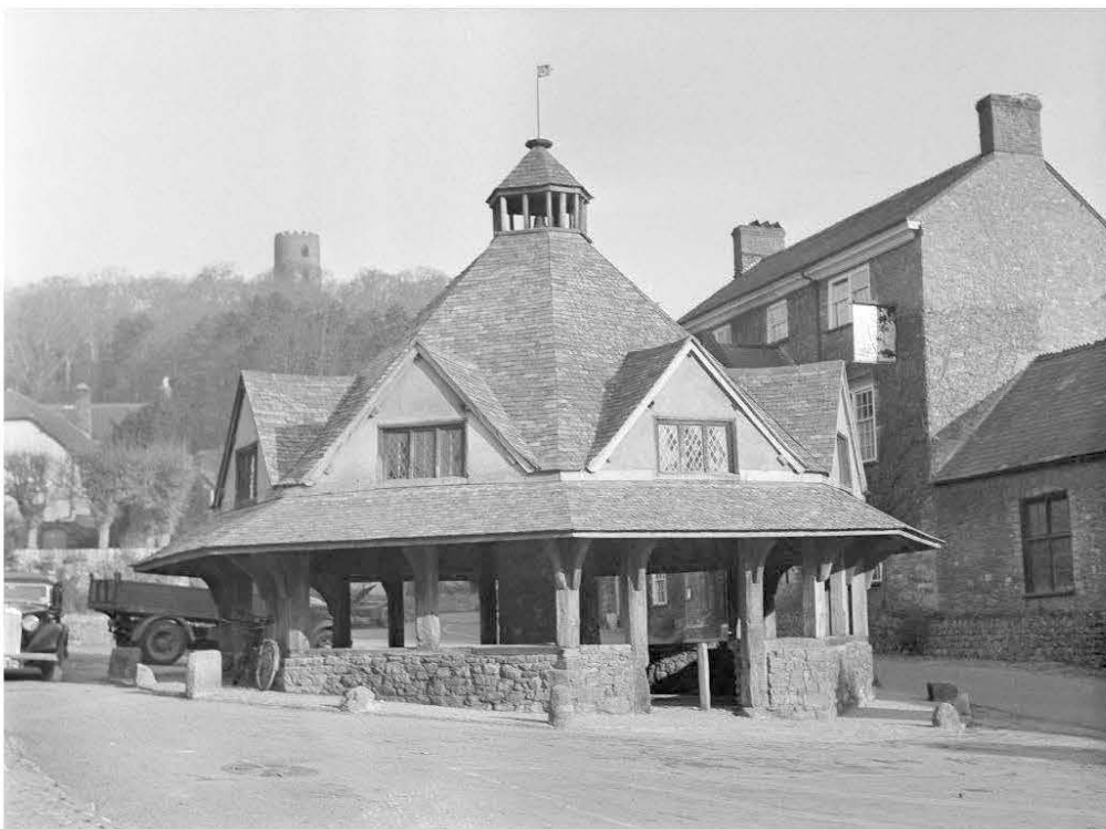
Fig 21 Dunster Yarn Market in 1953 after the Ministry had finished work on the monument. Reproduced by permission of English Heritage
