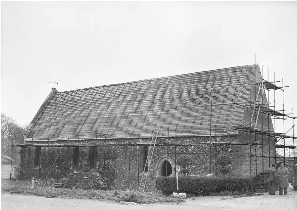
Fig 25: Duxford Chapel during restoration, 1953; the former roof covering of thatch is being replaced with tiles. Reproduced by permission of English Heritage
